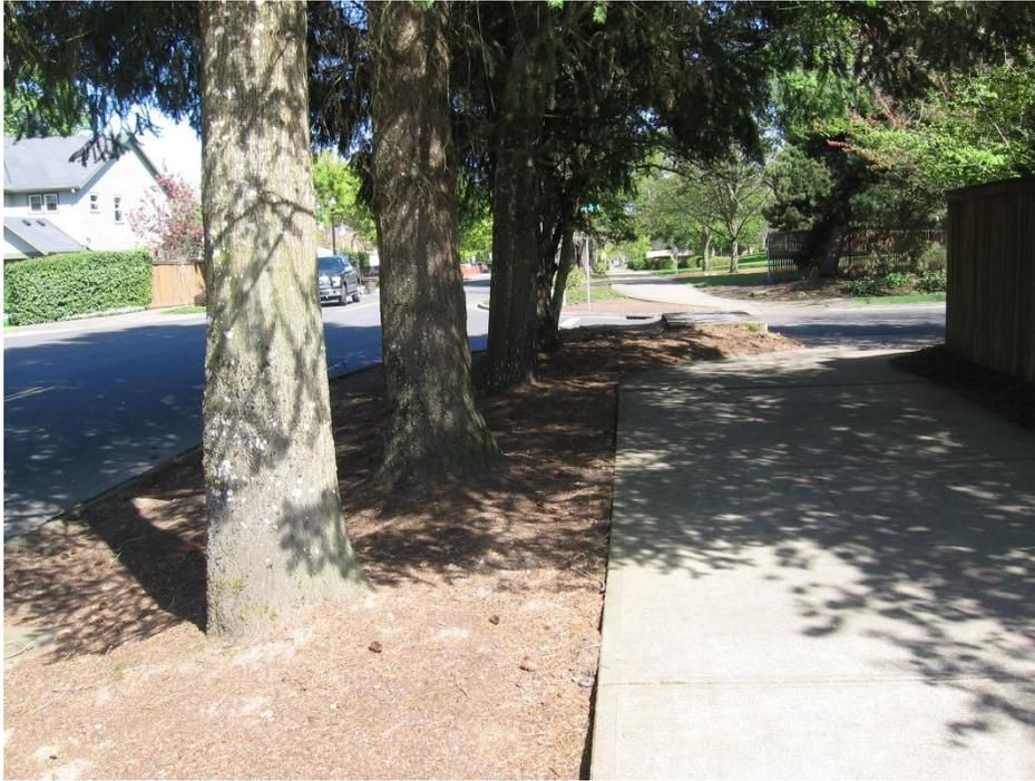
Alignment of the sidewalk veers prior to street crossing. This is to make room for the utility vault which is located within public right-of-way, and elevated significantly above proper grade.
