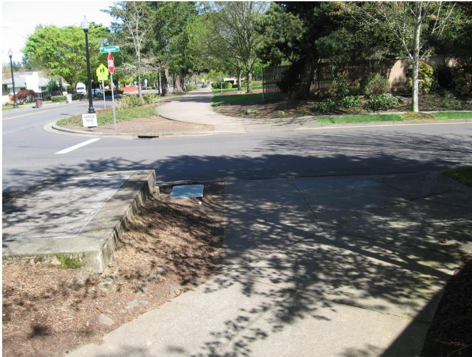
Photo of the actual existing pedestrian crossing conditions. Note that the stop sign and stop bar are located in front of the pedestrian crossing. Essentially, stopped vehicles will stack back into and through the pedestrian crossing. There is no existing pedestrian crossing striping that delineates the crosswalk area. Also, there are no ADA truncated dome textile inserts in the ramp areas of the crossing. This crossing does not meet current FHWA standards.
