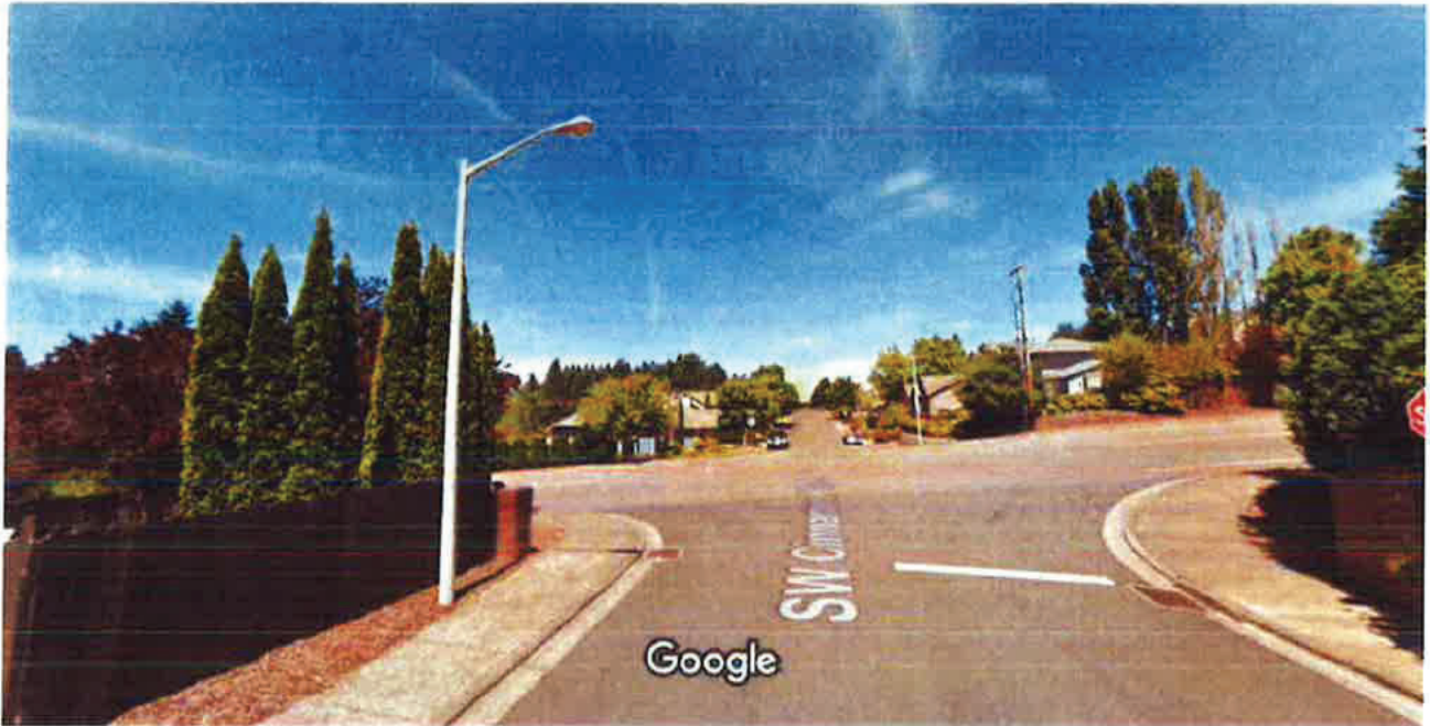
Cinnamon Hills Place (South Side) Looking North Sunset Blvd road grade approximately 6%+ Significant road crown crossing north to south on Cinnamon Hills Pl. Sight distance issues readily apparent. Possible safety concerns
