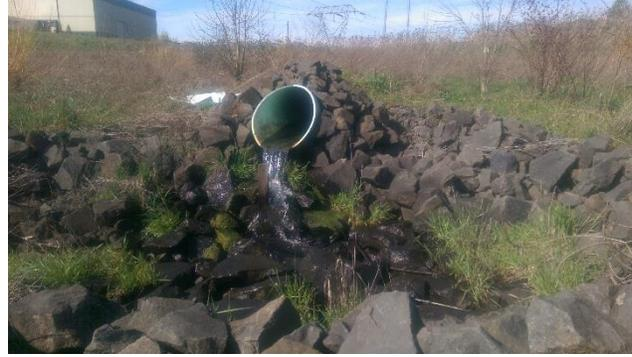
**Figure 6. Outfall piped across floodplain to Rock Creek**
