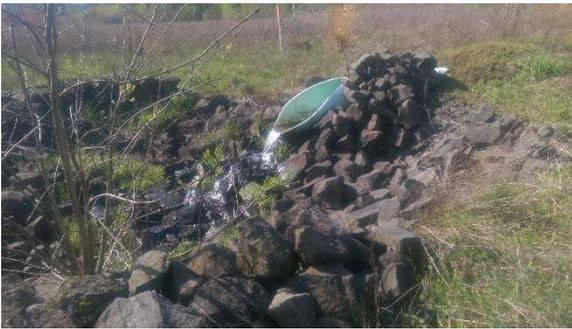
Figure 1. Outfall piped to the edge of Rock Creek
