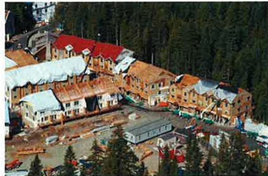
Collins Lake Resort, Government Camp, OR, during new roof truss installation
