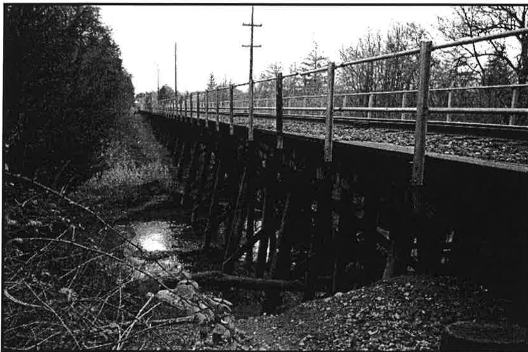
Figure 3.8-6 - Durham Trestle, East Side (Timber Pile Trestle Ballast Deck)
