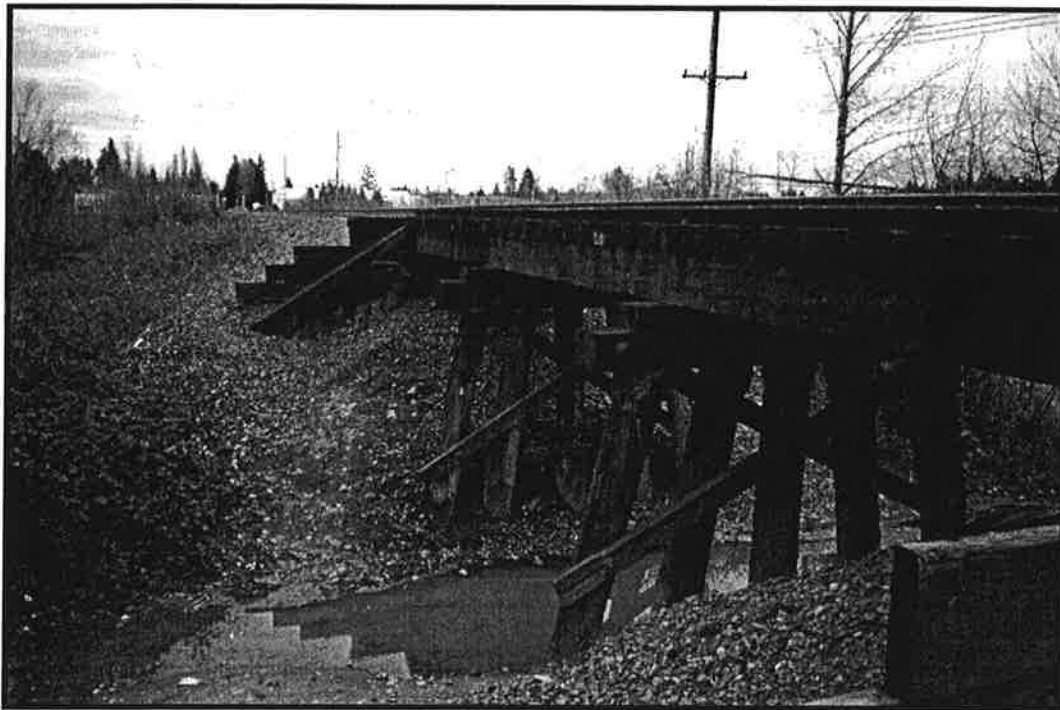
Figure 3.8-5 - Ash Street Trestle, looking South (Timber Pile Trestle open Deck)
