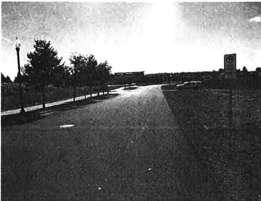
Photo 1: Looking south on Copper Terrace from Edy Road
