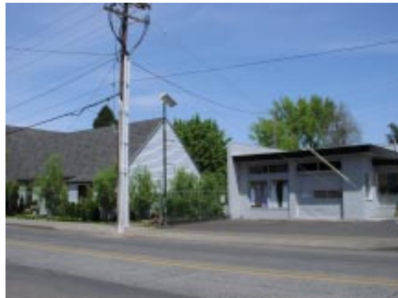
Sidewalk on Pine Street is inhospitable with the absence of a pedestrian buffer zone.
