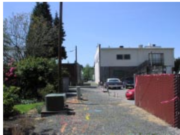
Alleyway enhancement will necessitate the relocation of existing above grade utilities.
