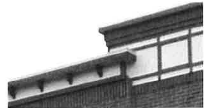
EXAMPLE OF CORNICE
