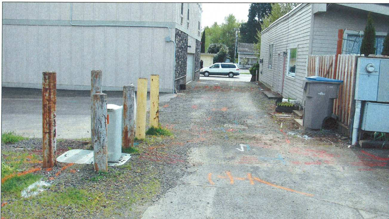
EXISTING CONDITIONS LOOKING SW ALONG ALLEY TOWARDS SW MAIN STREET
