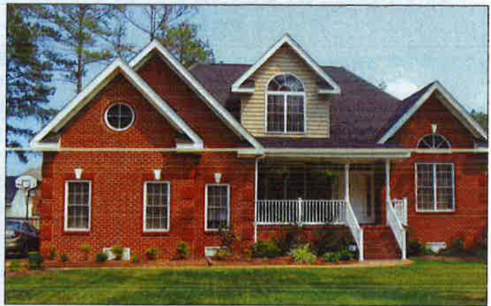
Elevated home on crawl space foundation
