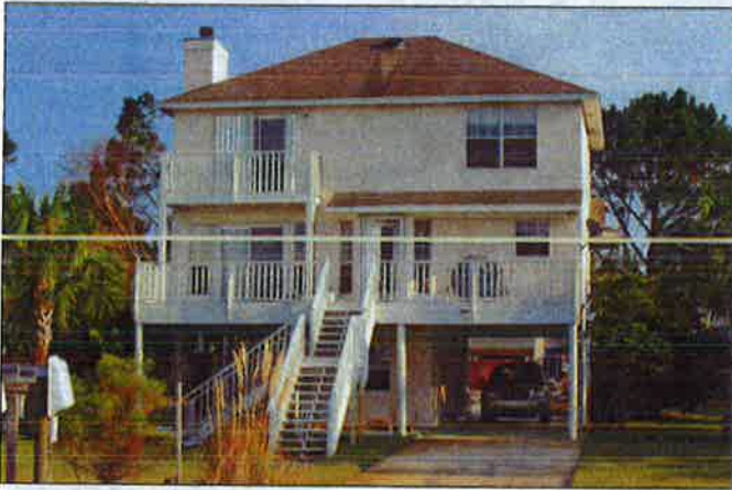
Elevated home on pile foundation
