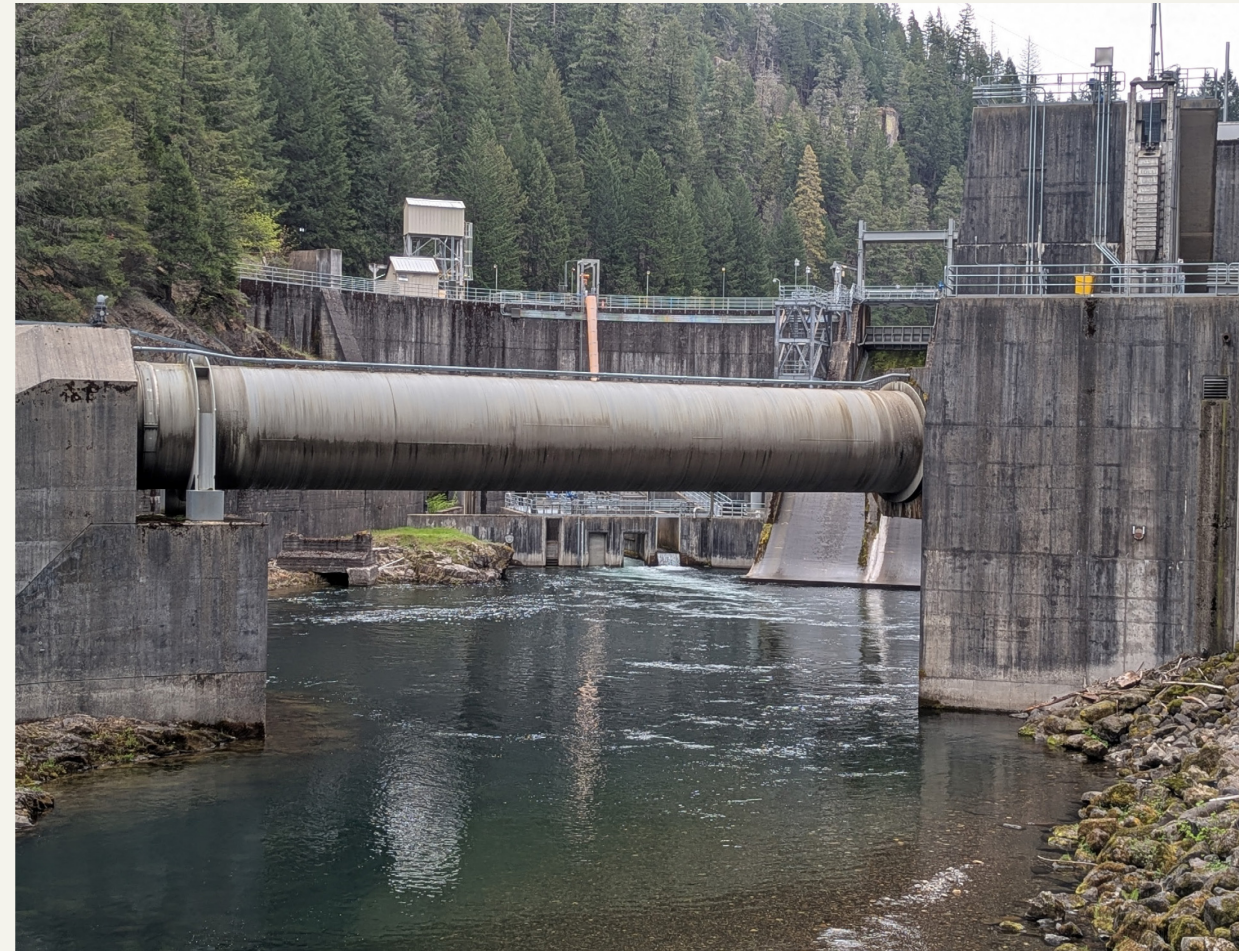
Soda Springs Dam
