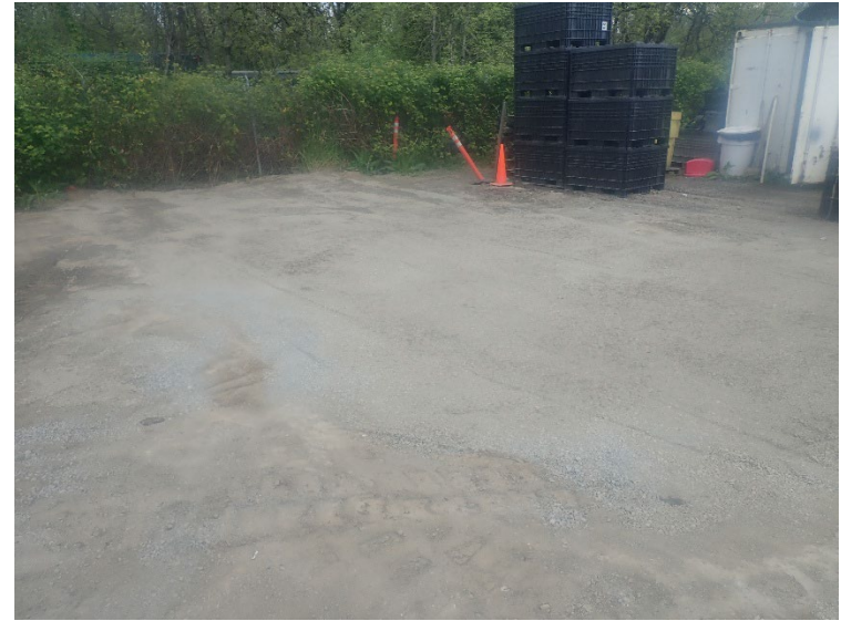
Following removal, both areas were backfilled with clean imported gravel.
