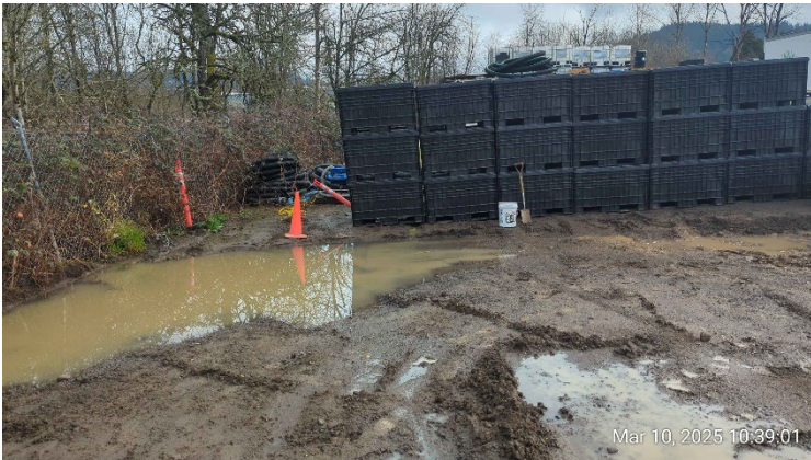
Ponding of rainwater observed in the vicinity of the spill area provided visual evidence of the possible extent of impacts from the acid spill and was utilized to inform decisions regarding the decision unit area.
