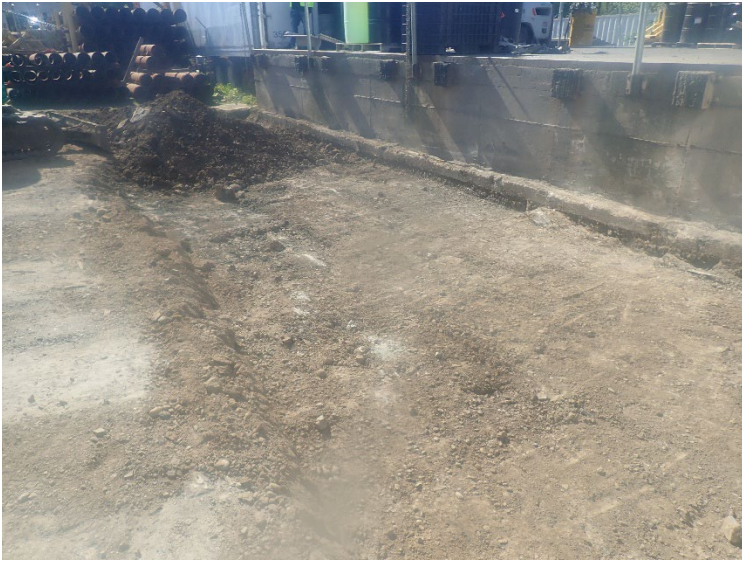
View of soil removal within the DU01 area.
