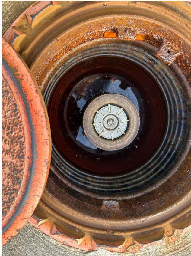
13: Regular #2 vapor return with water present
