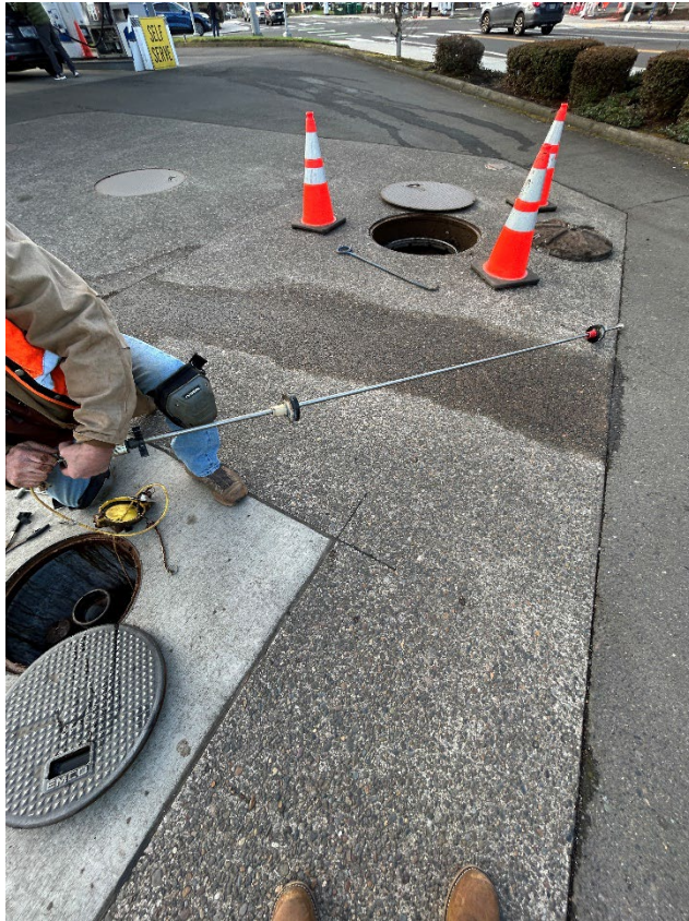
5: Pulling of the probe to enable the alarm
