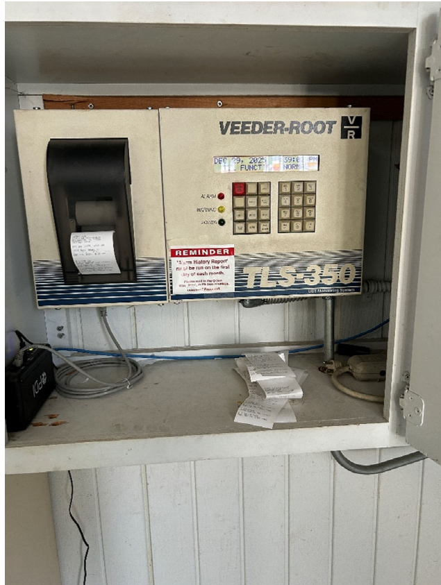
3: ATG – TLS 350 – All functions normal
