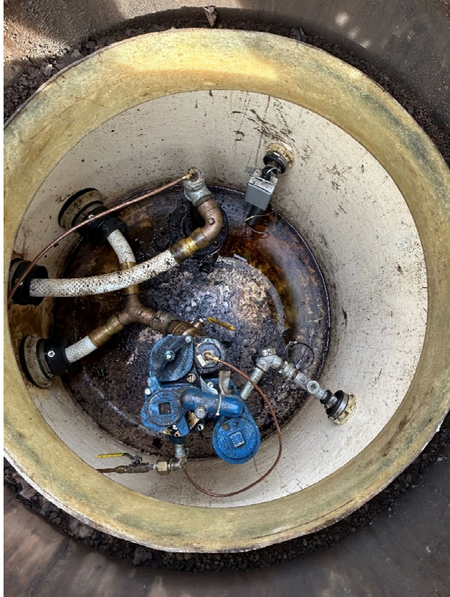
29: Regular sump #1 – Less than 2” of product present in sump
