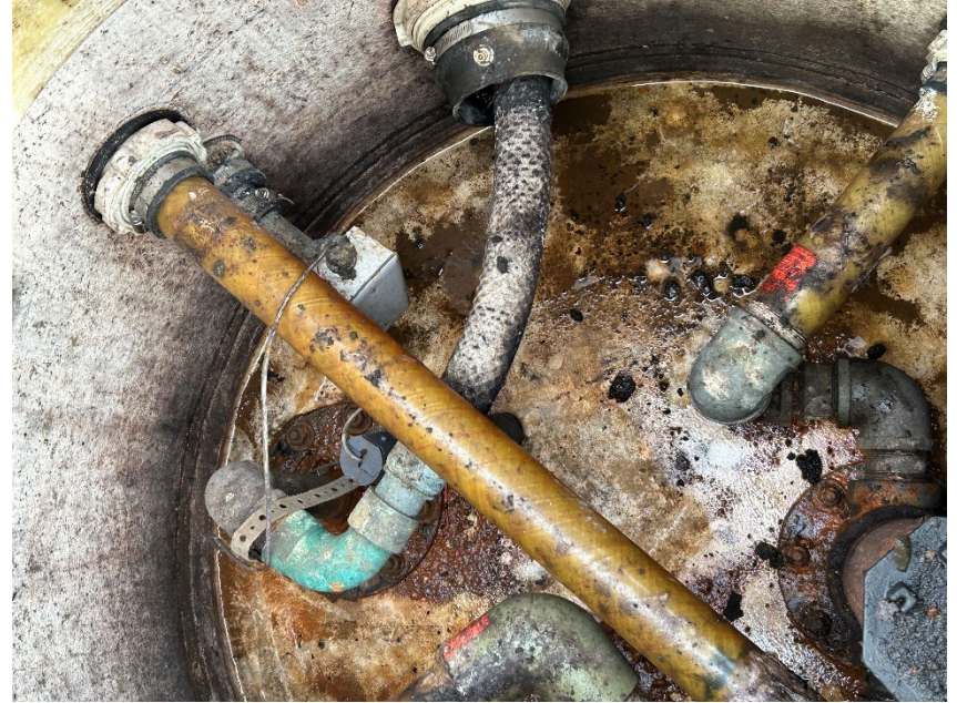
34: Regular transition sump
