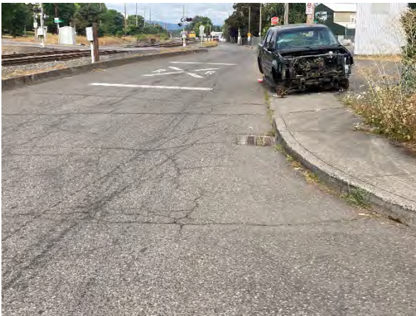
Photo #5 ANB988: Receiving from N Colombia Blvd – Tax Lot 900 (view West looking down N Frontage Rd, NW Cast is to the right).
