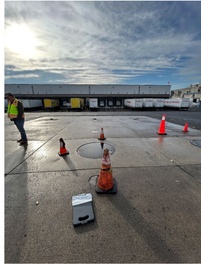
2: Tank nest for dispensing tanks looking south
