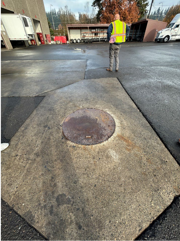
12: Transition sump area looking north
