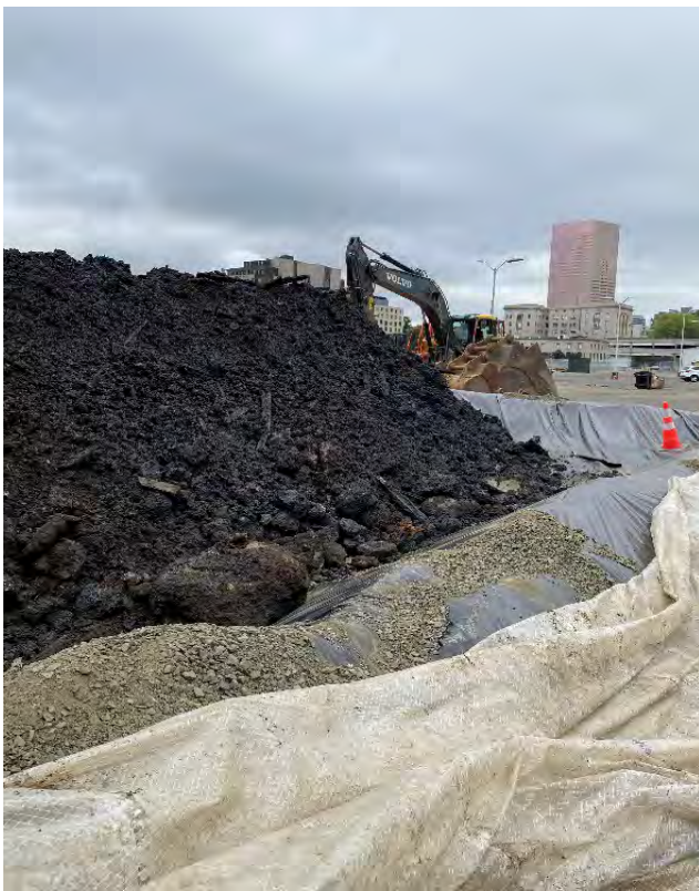
Photo 13: Contaminated Soil Stockpile
