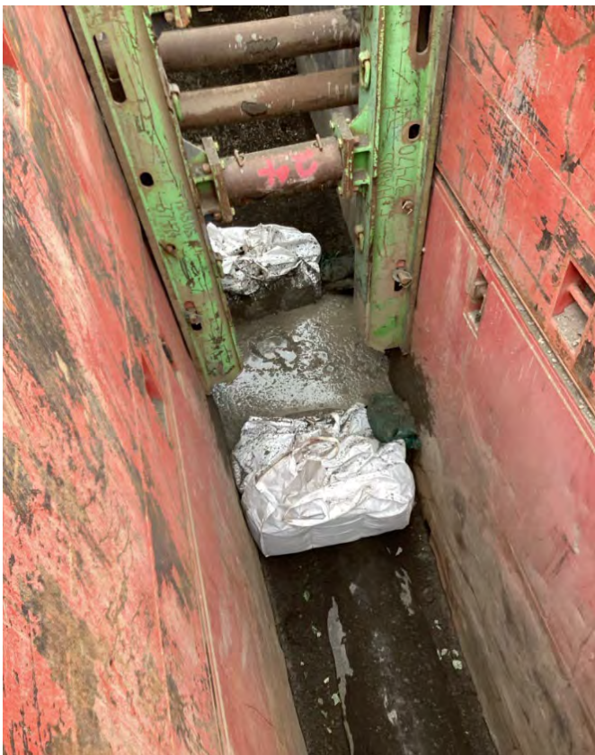
Photo 17: Trench Plug Construction - NW 9th Ave at Johnson
