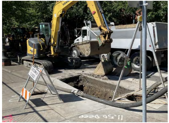
Photo 2: Excavating Bursting Pit at NW 9th and Kearney
