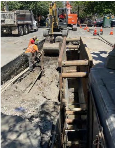
Photo 3: Bursting Pit with Shoring - NW 9th Ave and Johnson
