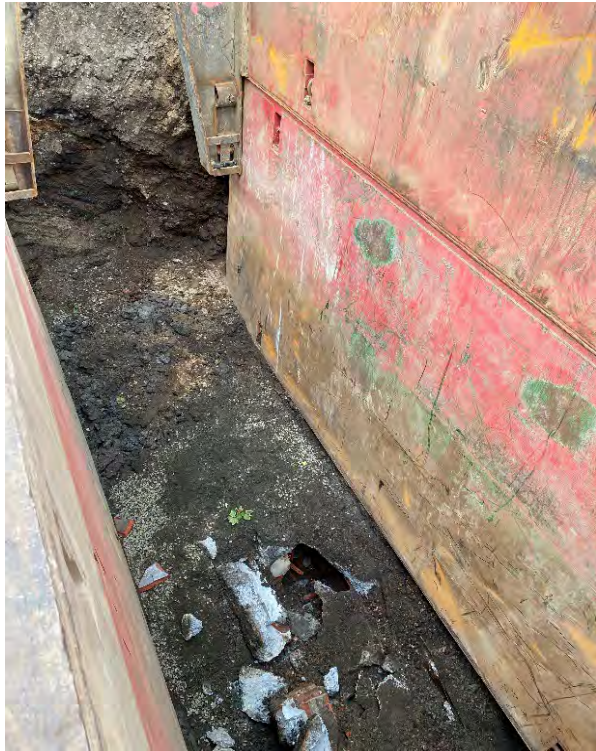
Photo 7: 24-inch Storm Sewer - NW 9th Ave and Lovejoy
