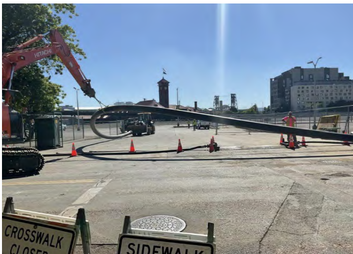
Photo 5: Preparing to install HDPE Sanitary Sewer
