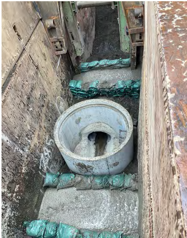
Photo 15: Trench Plug Construction - NW 9th Ave at Kearney
