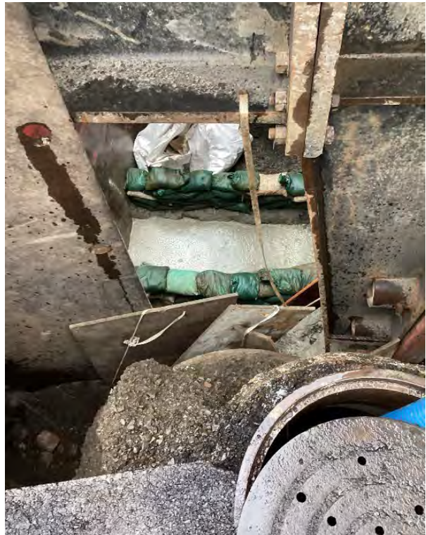
Photo 16: Trench Plug Construction - NW 9th Ave at Lovejoy
