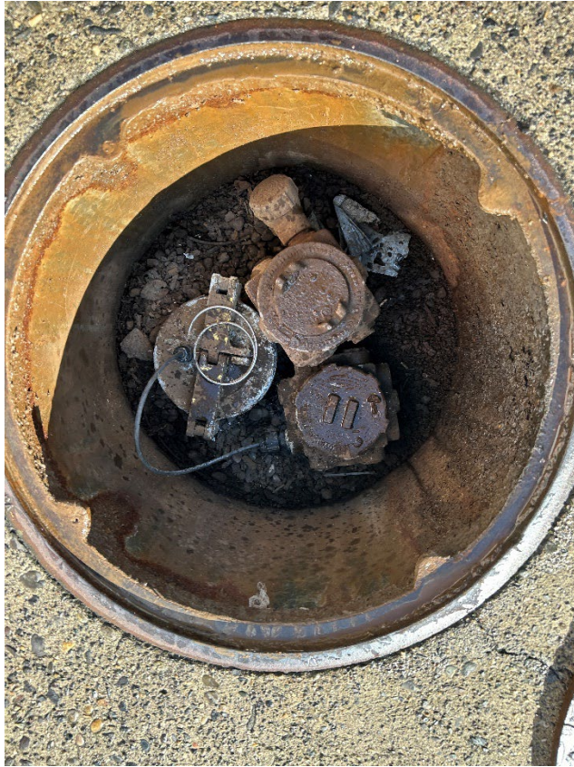
9: Diesel probe and interstice
