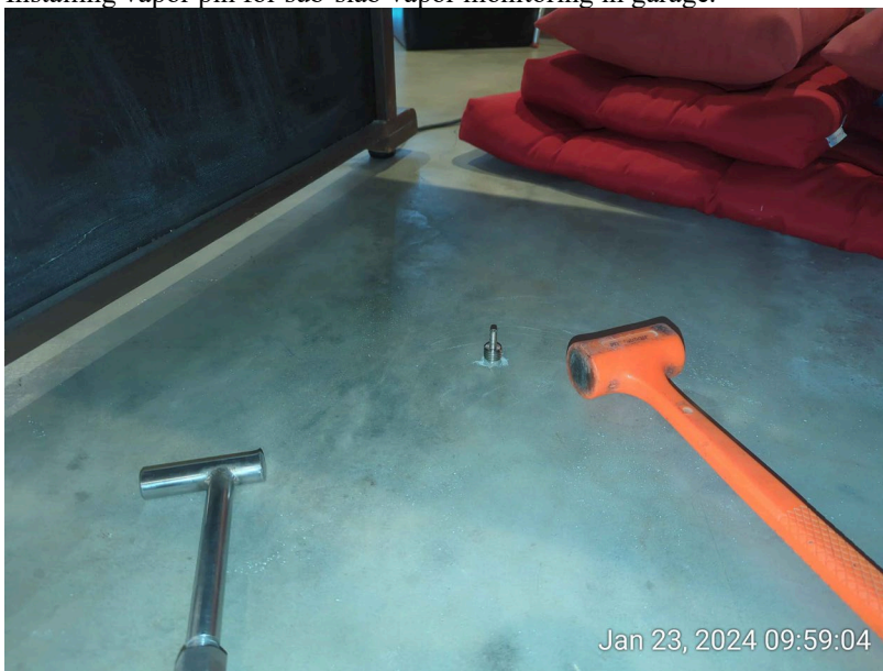
Vapor pin installed.
