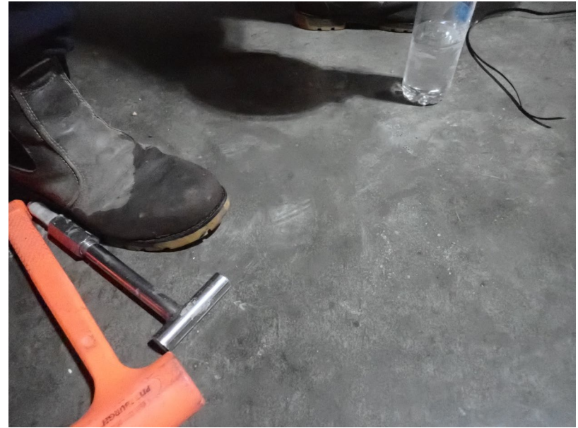
Vapor pin removed and floor restored.
