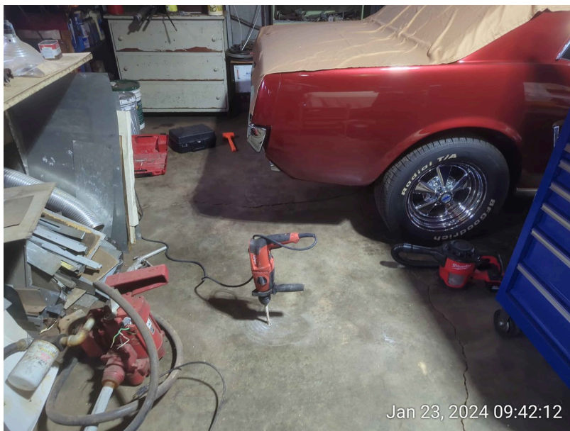
Installing vapor pin for sub-slab vapor monitoring in garage.
