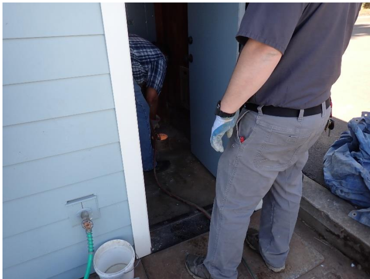
Cutting off well casing below concrete grade
