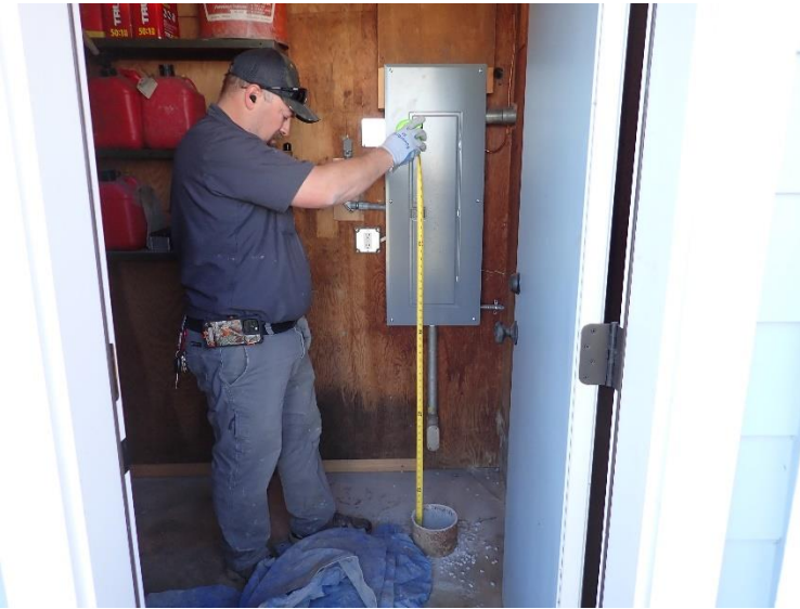
Measuring depth of bentonite in well
