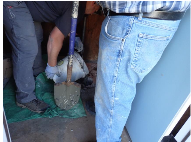
Topping off decommissioned well with concrete
