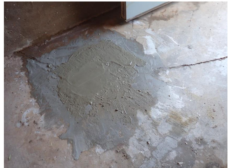
Concrete brought up to grade with the floor
