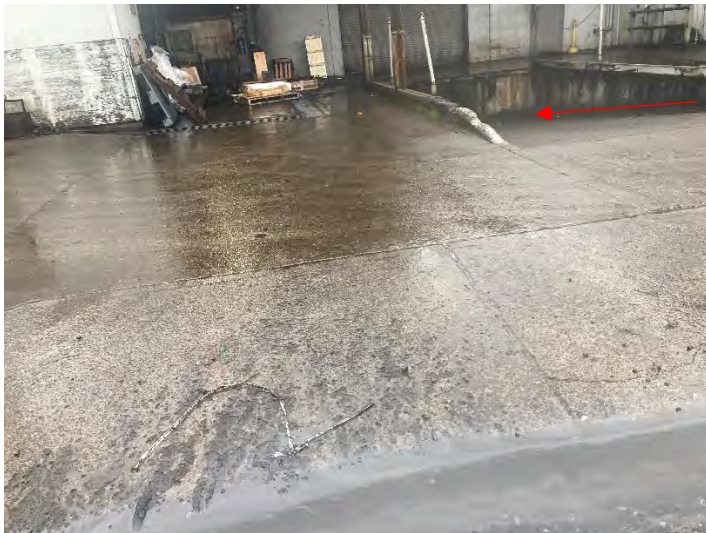
Area on east side that sheet flows to MS4. Catch basin noted with arrow and trench drain on left. Note sediment-laden, oily discharge to MS4. 11/23/20; K. Balogh
