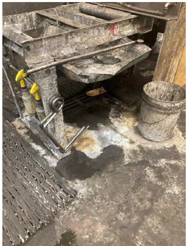
Interior floor drain under pressure test area. 11/23/20; K. Balogh
