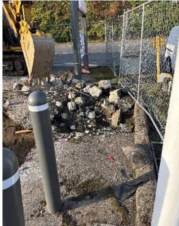
Photo #9 Removing kerosene dispenser
