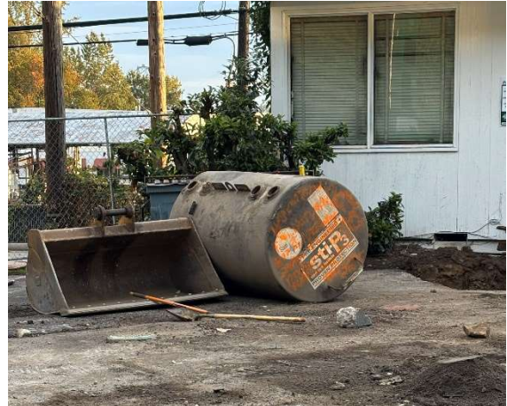
Photo #4 View of removed Kerosene UST
