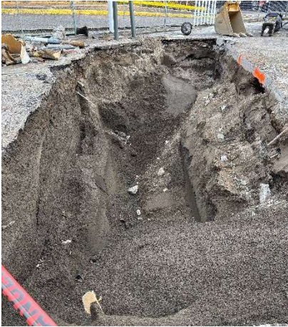
Photo #7 View of UST pit after diesel and kerosene USTs removed
