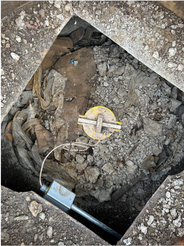
9: Tank gauge probe for clean premium
