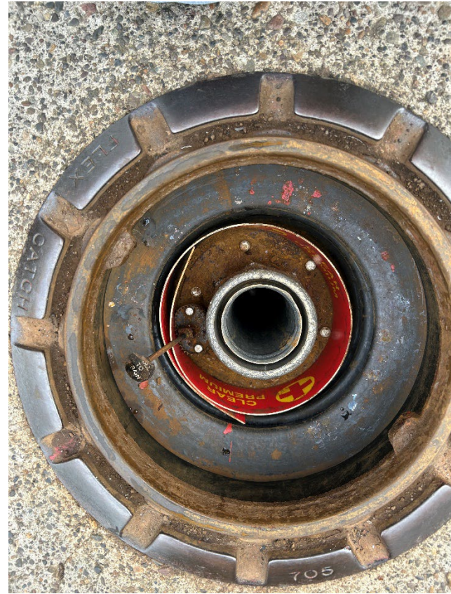
8: Clean premium fill with coaxial drop tube
