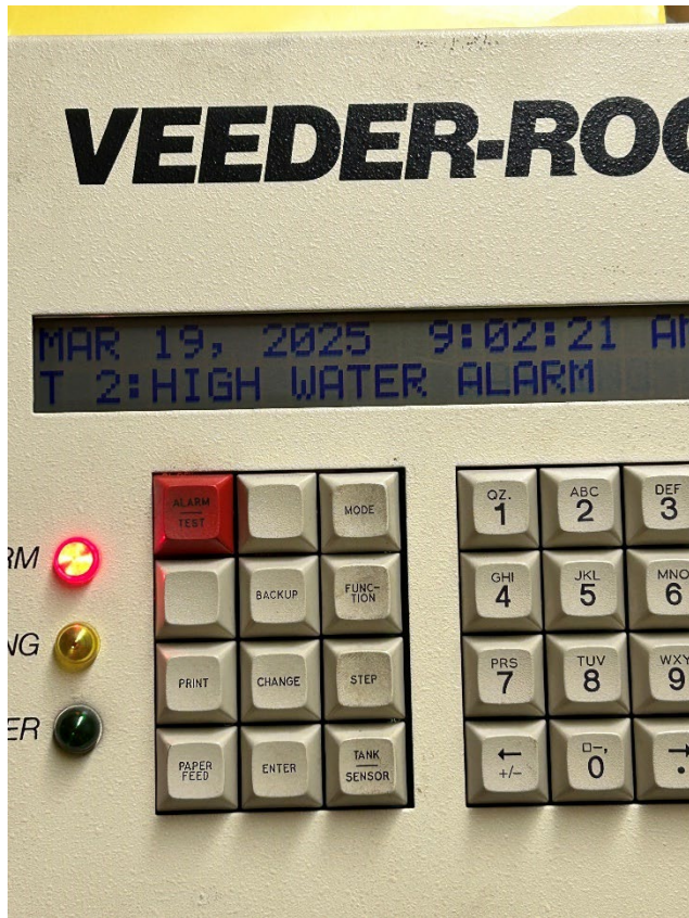
13: Tank 2 midgrade unleaded in alarm for high water
