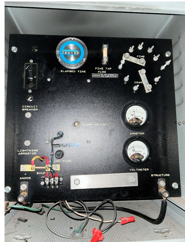
14: Impressed current system
