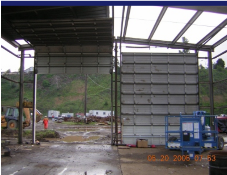
Photo 5 Shop building with siding removed. Direction: East
