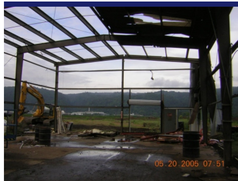
Photo 4 Shop building with siding removed. Direction: West
