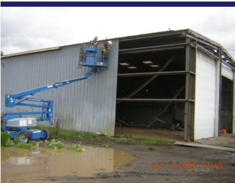
Photo 3 Shop siding being removed. Direction: West
