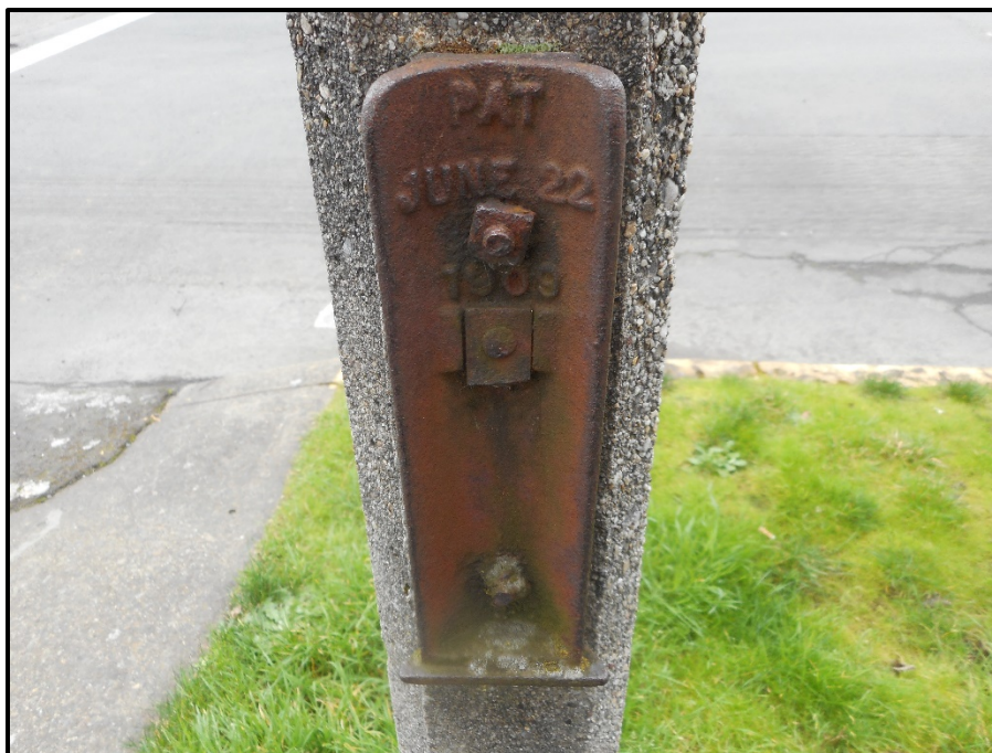
Figure 26. Close up of the broken bracket that was observed on three out of the five Mail Posts.
