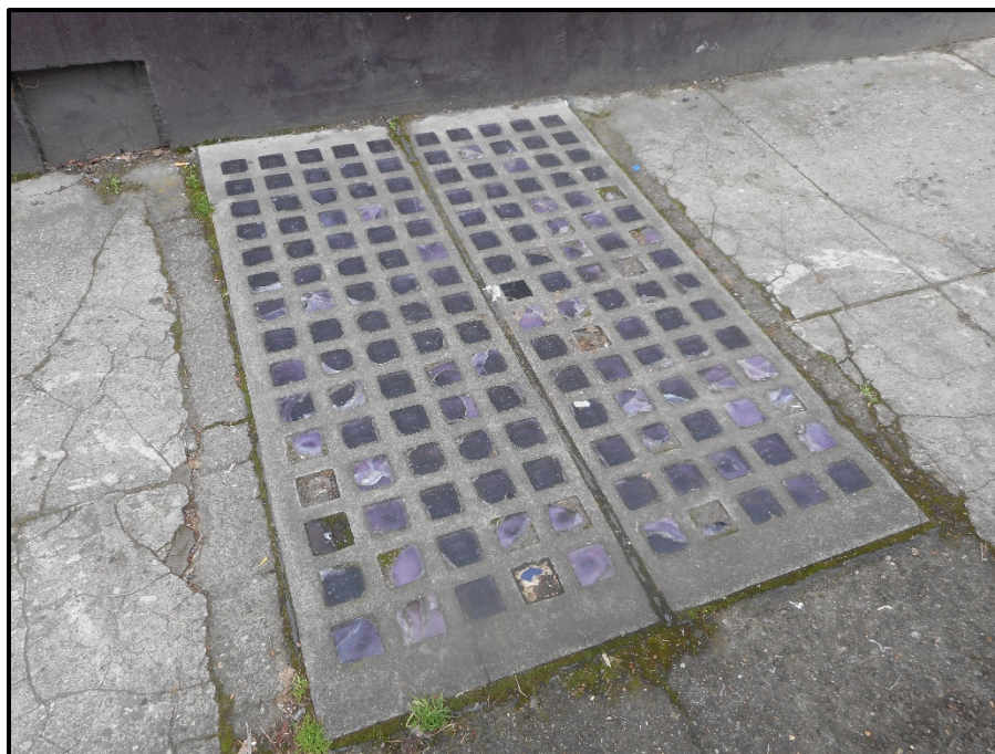
Figure 82. Feature 1, sidewalk vault light along the west side of S College Street.
