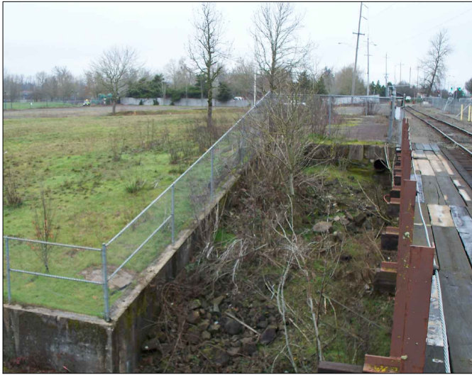
PHOTO 1 Soil removal area and adjacent property prior to commencement of excavation.
