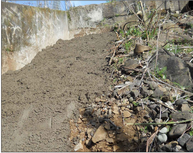
PHOTO 4 Placement of CDF as part of cover and site restoration.
