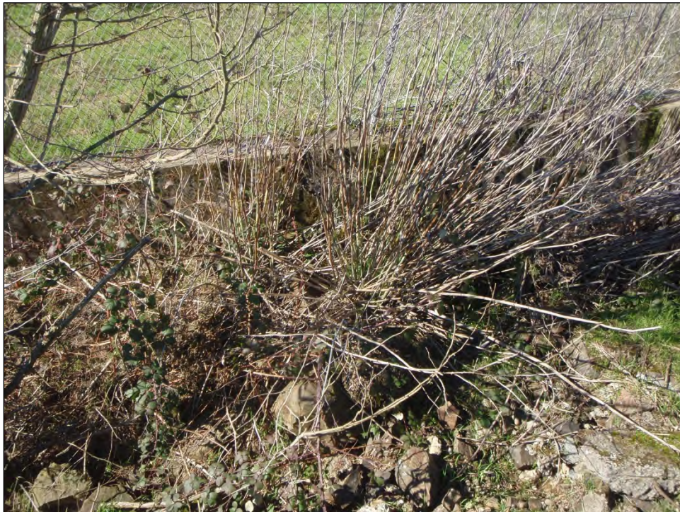
Photo B. Downslope of Photo A.
