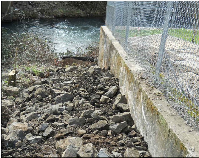
PHOTO 5 Completed restoration as seen from the northern retaining wall.
