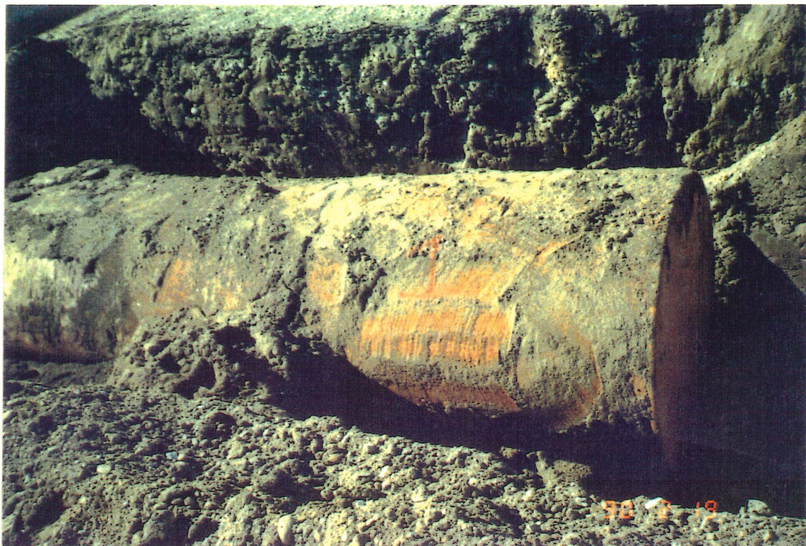
Figure 3: Hamrick site 1,000 gallon UST, labeled H-UST-1. The soil around the fill pipe, left of picture, is visually stained.
