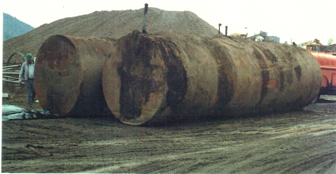
Figure 16: Kirtland Road UST's. The tanks are visually stained on the fill pipe end.
