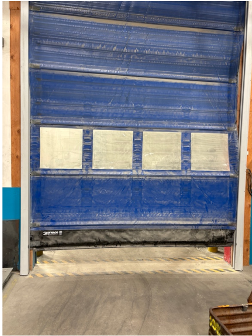
Photos: Tarp-type doors into areas controlled by DC#2 and DC#3 showing response (deformation) to vacuum for dust control equipment.
