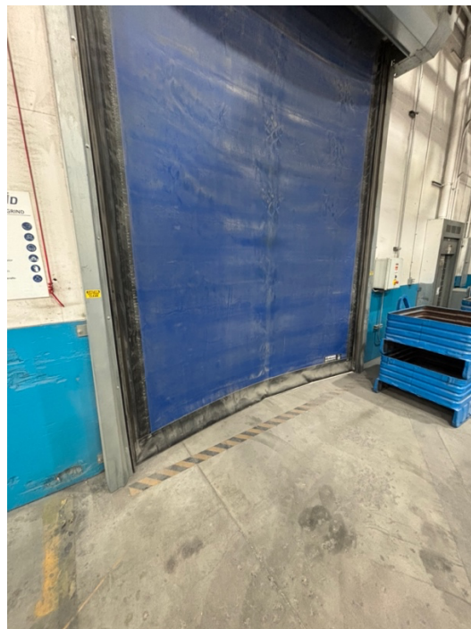
The preferential pathway for casting emissions to leave the building will be through dust control equipment, preferentially to DC#3. Therefore, a 99% control efficiency reflective of baghouse filters is appropriate for casting emissions.
