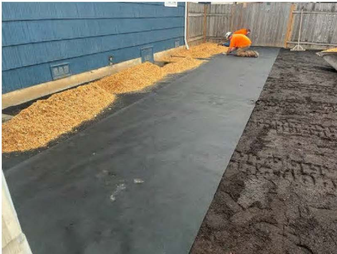
Photograph 3. Demarcation fabric/weed barrier and PlayAway fiber chip placing at [REDACTED] Baxter. Photo taken facing north.
