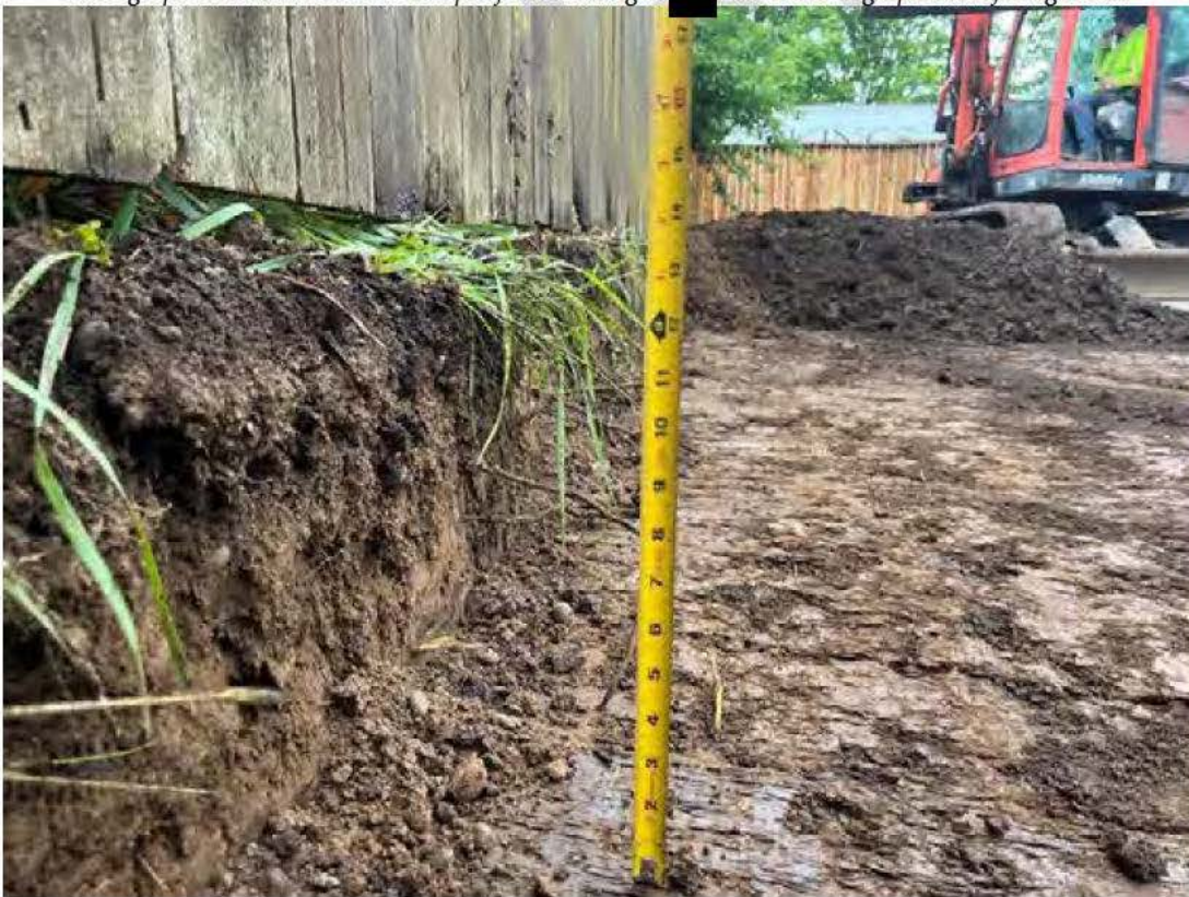
Photograph 4. Manual excavation depth field truthing at [REDACTED] Baxter. Photograph taken facing south.
