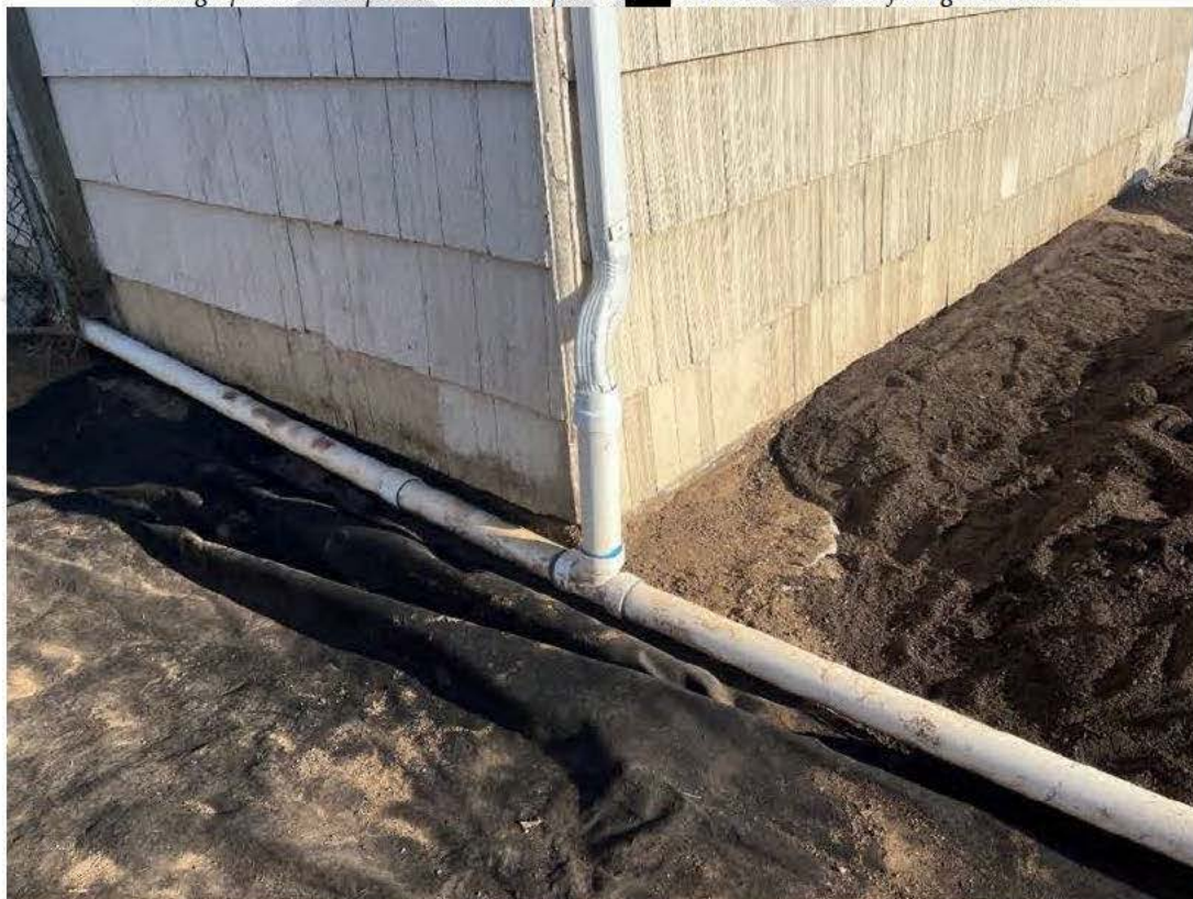
Photograph 2. Downspout drain line repair at [REDACTED] Baxter. Photo taken facing northwest.
