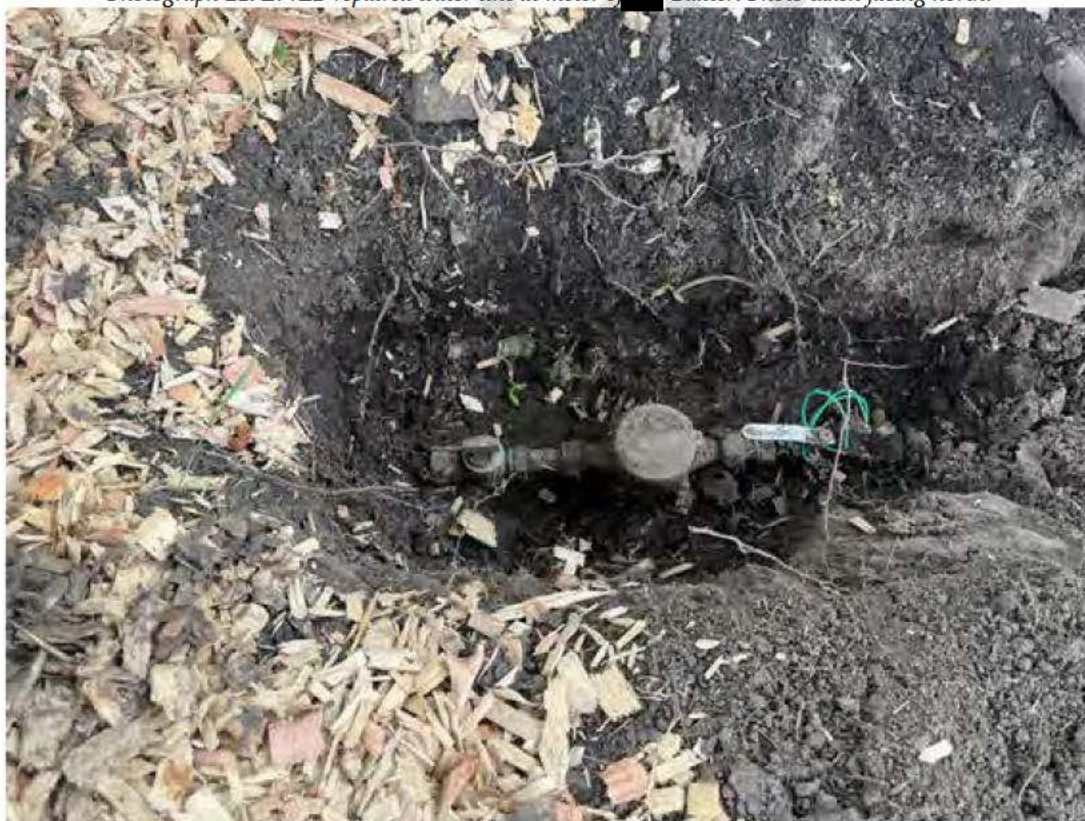
Photograph 21. EWEB repaired water line at meter of [REDACTED] Baxter. Photo taken facing north.
