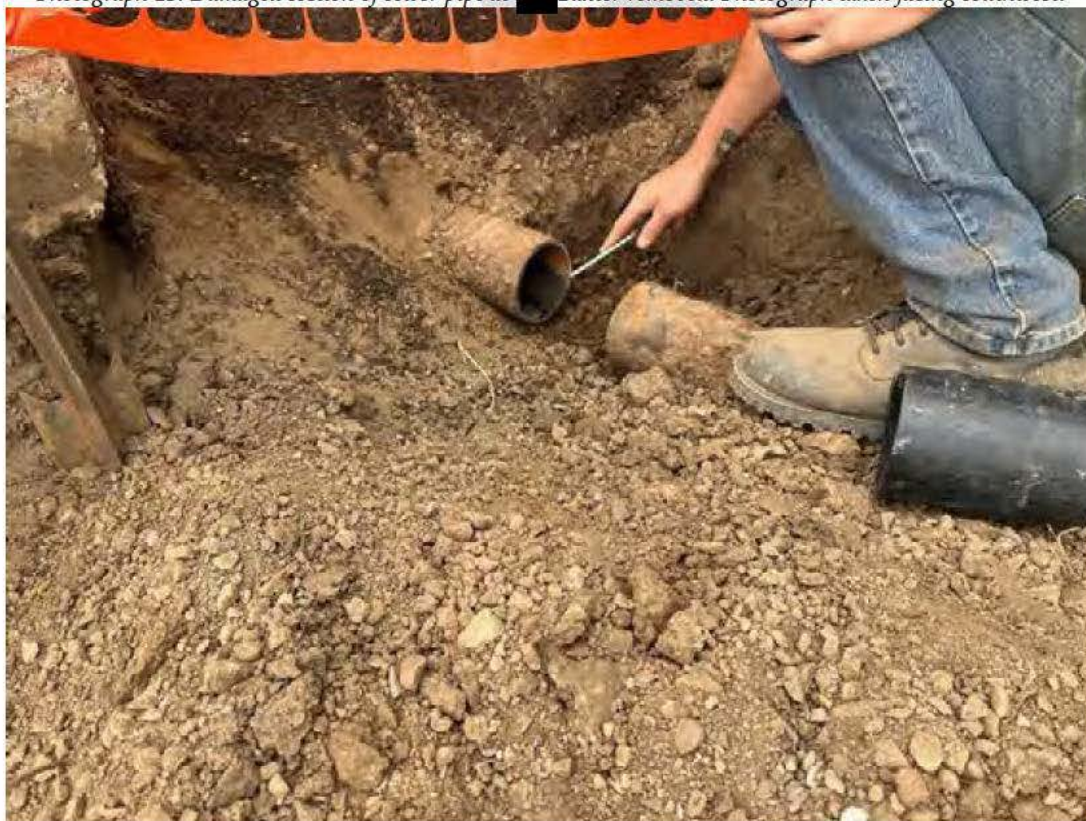
Photograph 13. Damaged section of sewer pipe at [REDACTED] Baxter removed. Photograph taken facing southwest.
