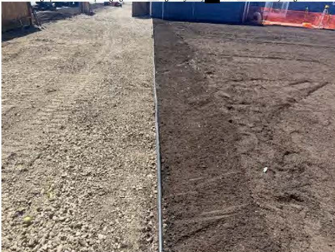
Photograph 22. Landscape edging installed along backyard of [REDACTED] Baxter. Photo taken facing west.
