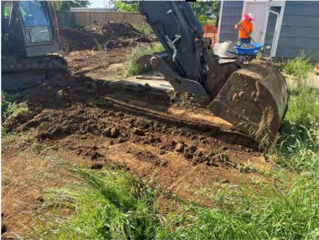
Photograph 4. Compacting additional gravel placed at [REDACTED] Baxter. Photo taken facing northeast.
