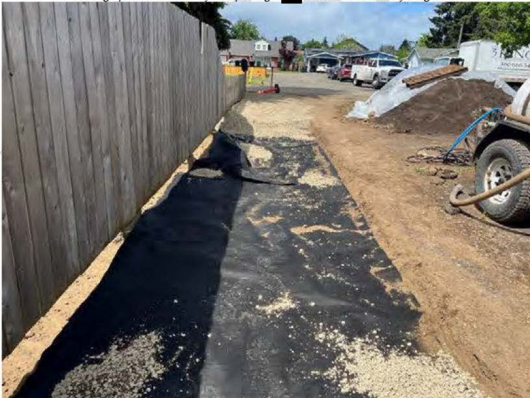
Photograph 19. Gravel and fabric placing at [REDACTED] Baxter. Photo taken facing west.
