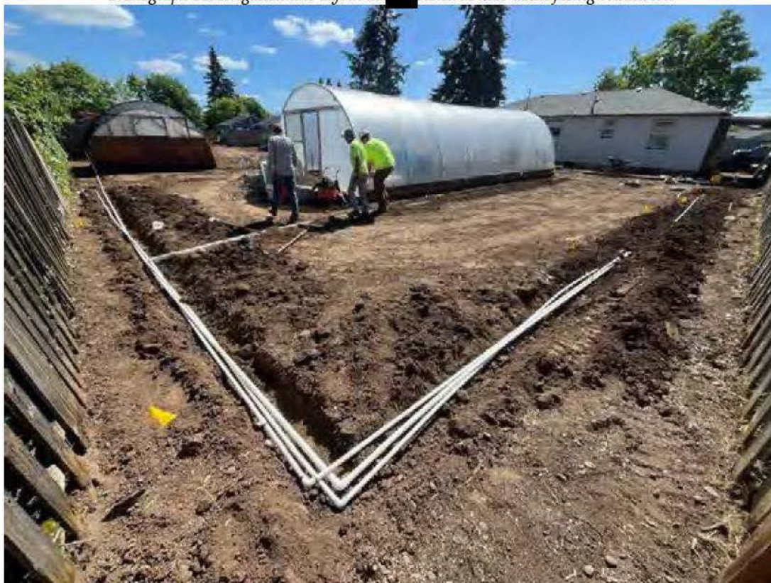
Photograph 31. Irrigation line layout at [REDACTED] Baxter. Photo taken facing southwest.
