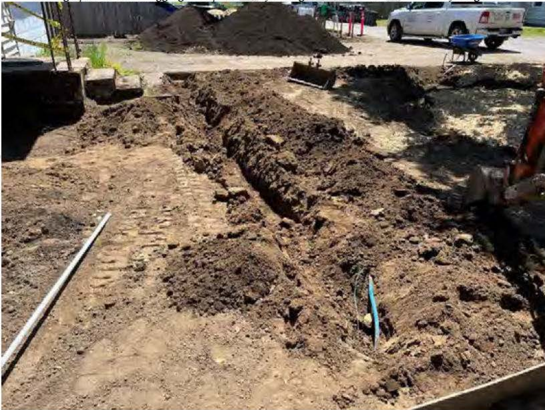
Photograph 16. Trench digging in imported soil for irrigation line install. Photo taken facing south.
