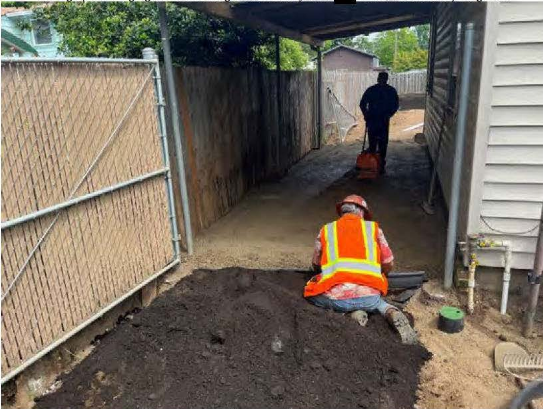
Photograph 26. Edging installation at gravel/soil interface at [REDACTED] Baxter. Photo taken facing east.
