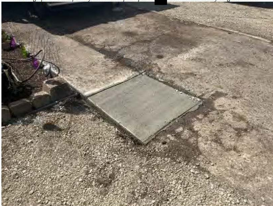
Photograph 19. Form pulled from concrete pad repair at [REDACTED] Baxter. Photo taken facing northwest.
