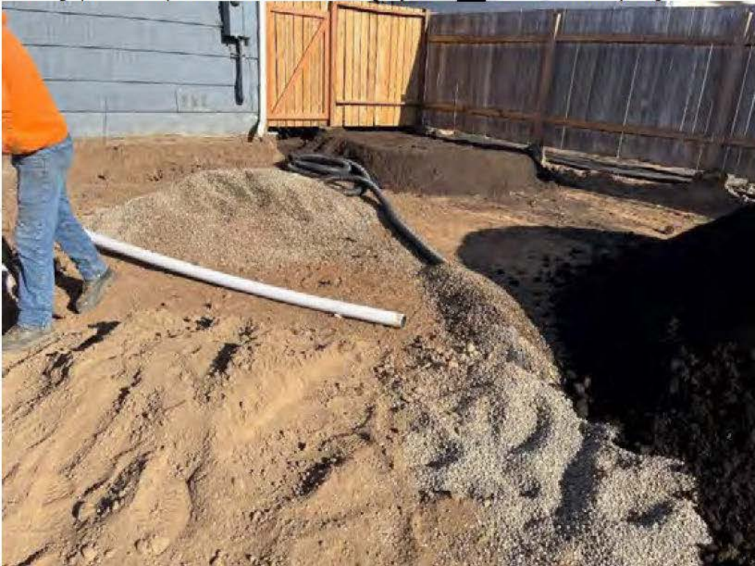
Photograph 6. Downspout drain line tie in to existing drywell at [REDACTED] Baxter. Photo taken facing northwest.
