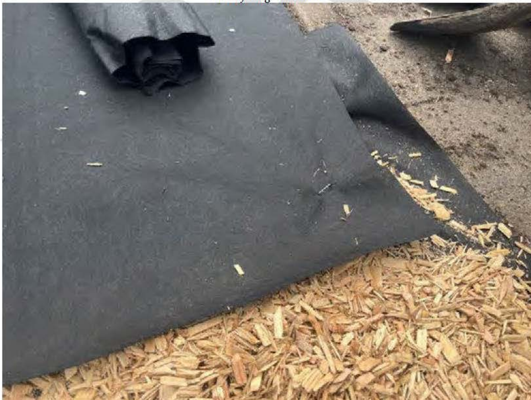
Photograph 16. Nonwoven construction fabric and landscape staples used for weed barrier at [REDACTED] Baxter. Photo taken facing southwest.
