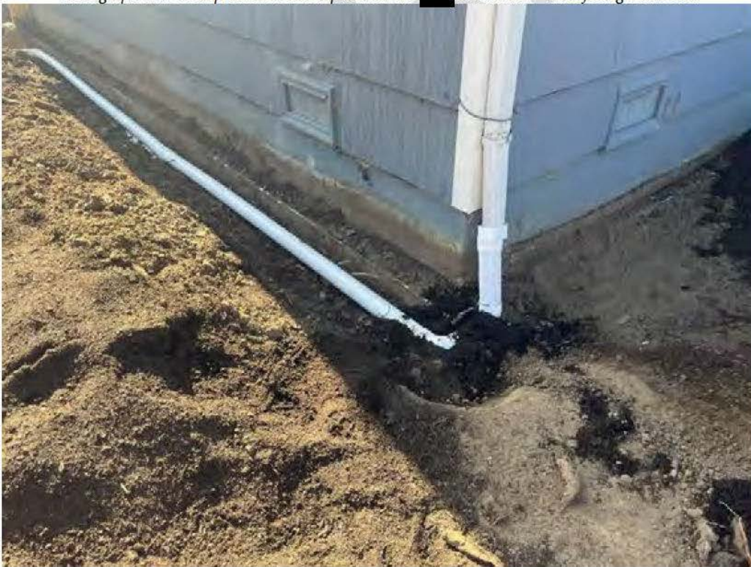
Photograph 10. Downspout drain line replacement at [REDACTED] Baxter. Photo taken facing southeast.
