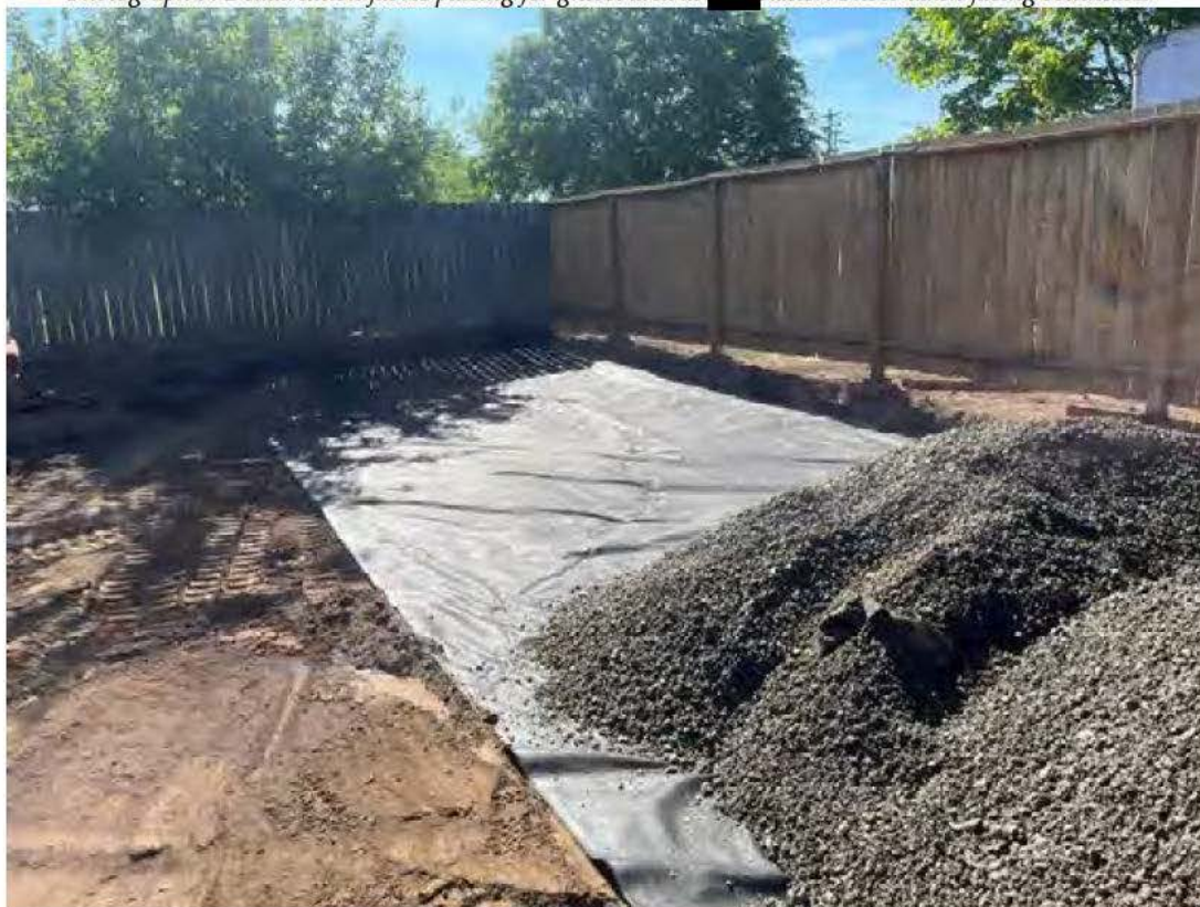
Photograph 8. Returning pea gravel to aquaponic system at [REDACTED] Baxter. Photo taken facing northwest.
