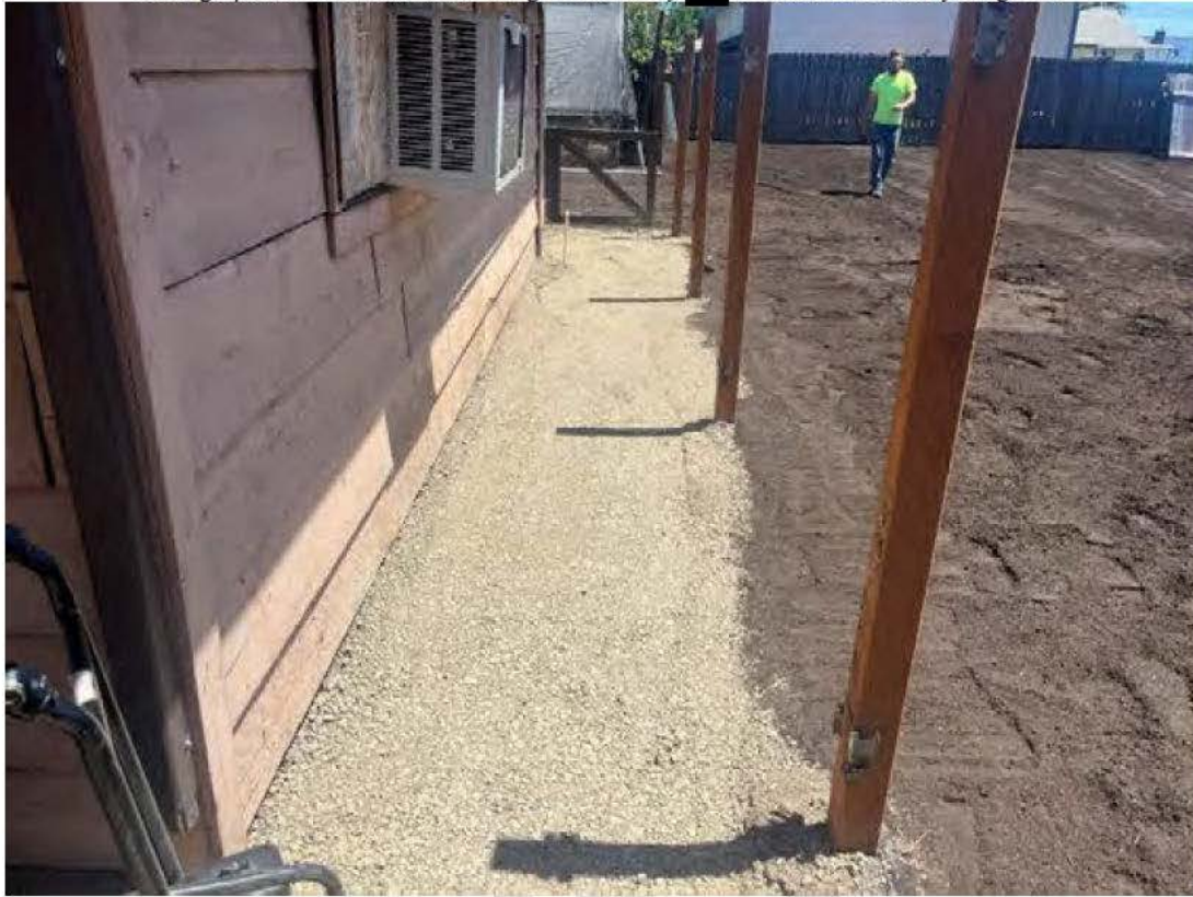
Photograph 18. Gravel mulch interface after spot backfilling at [REDACTED] Baxter. Photo taken facing west.
