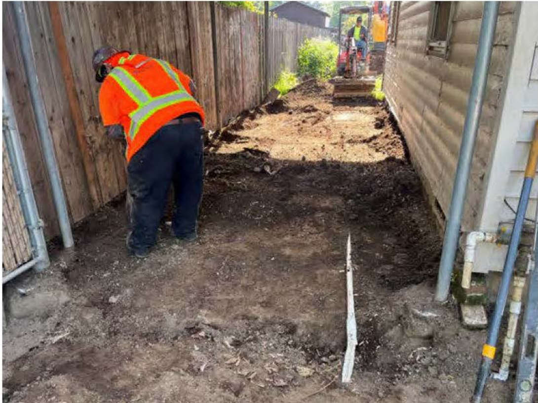
Photograph 4. Hand tools and mini-excavator used to remove soil from covered area at [REDACTED] Baxter. Photo taken facing east.
