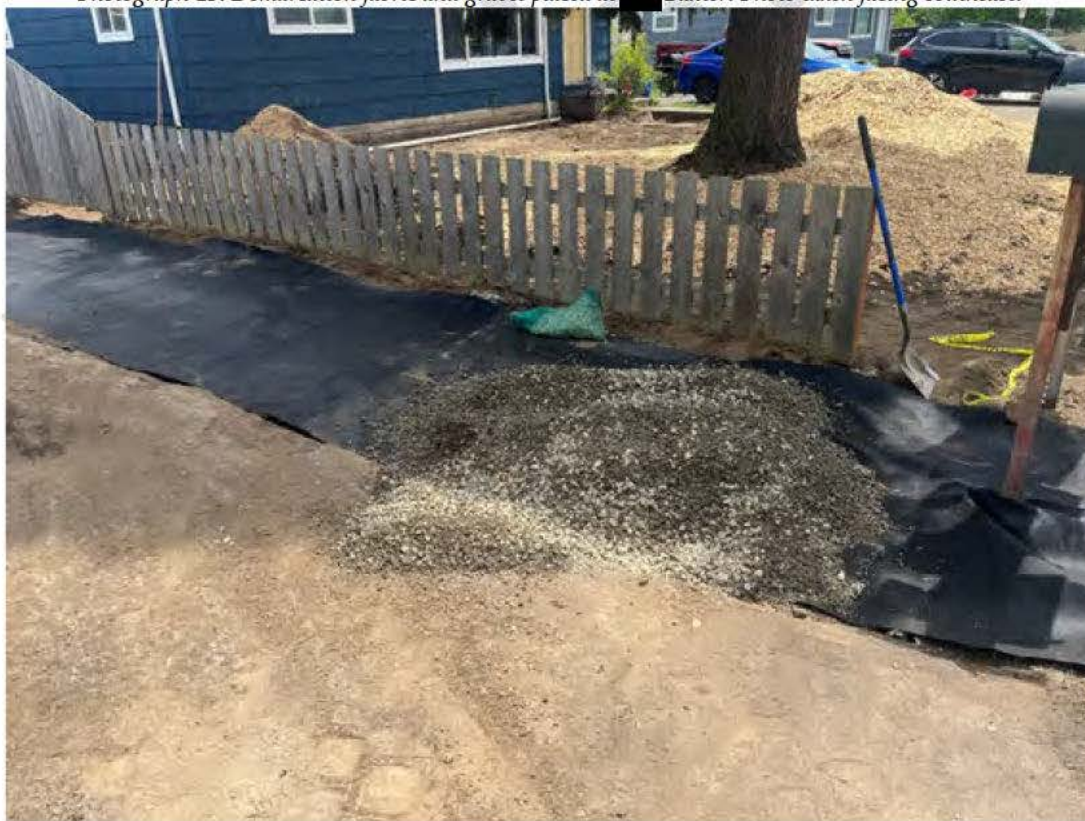
Photograph 15. Demarcation fabric and gravel placed at [REDACTED] Baxter. Photo taken facing southeast.
