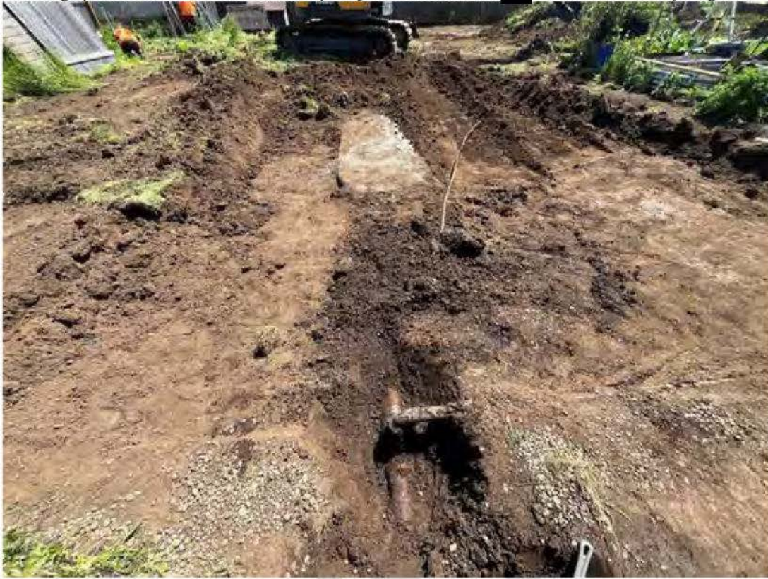
Photograph 10. Damaged downspout drain line at [REDACTED] Baxter. Photo taken facing south.
