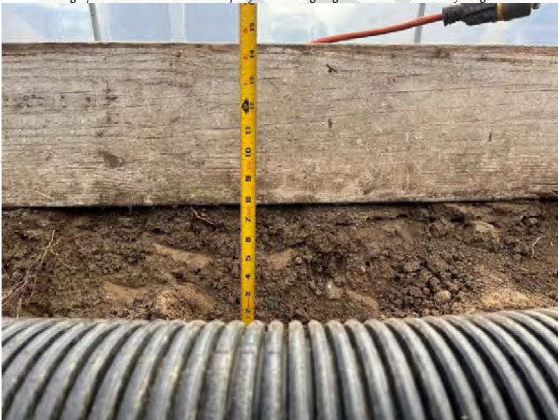
Photograph 31. Manual excavation depth field truthing in greenhouse. Photo taken facing south.
