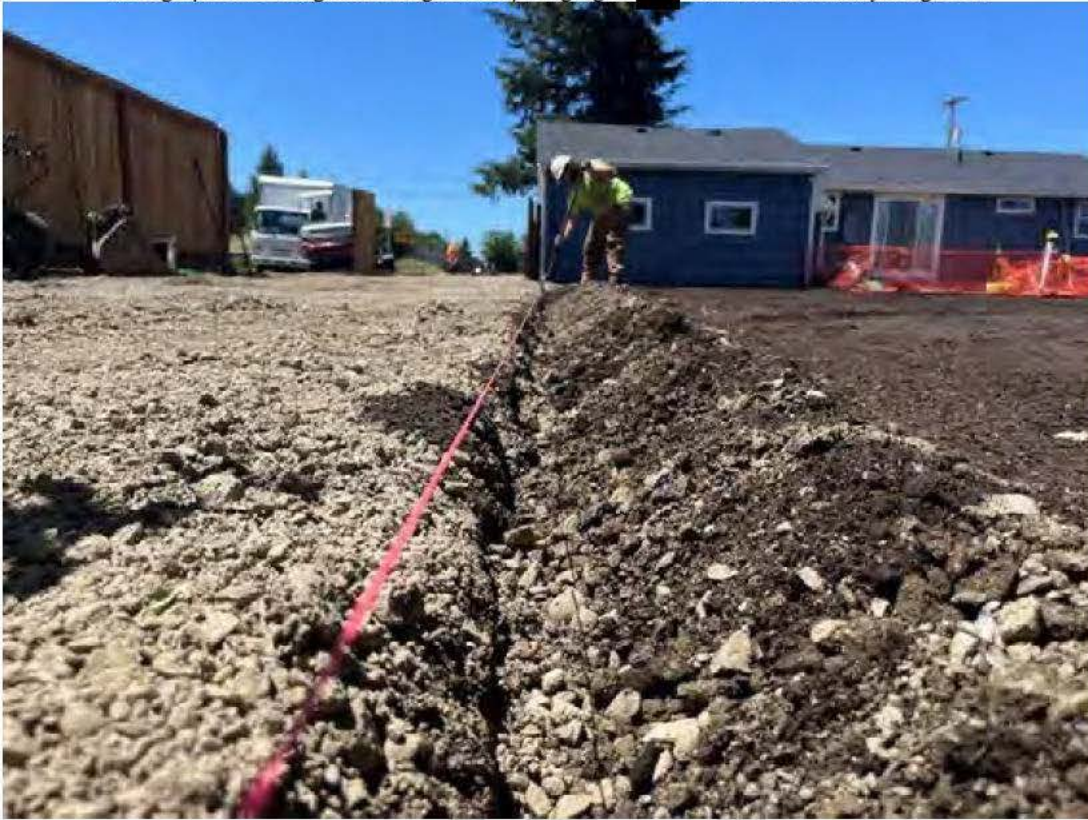
Photograph 18. Installing landscape edging at [REDACTED] Baxter. Photo taken facing east.
