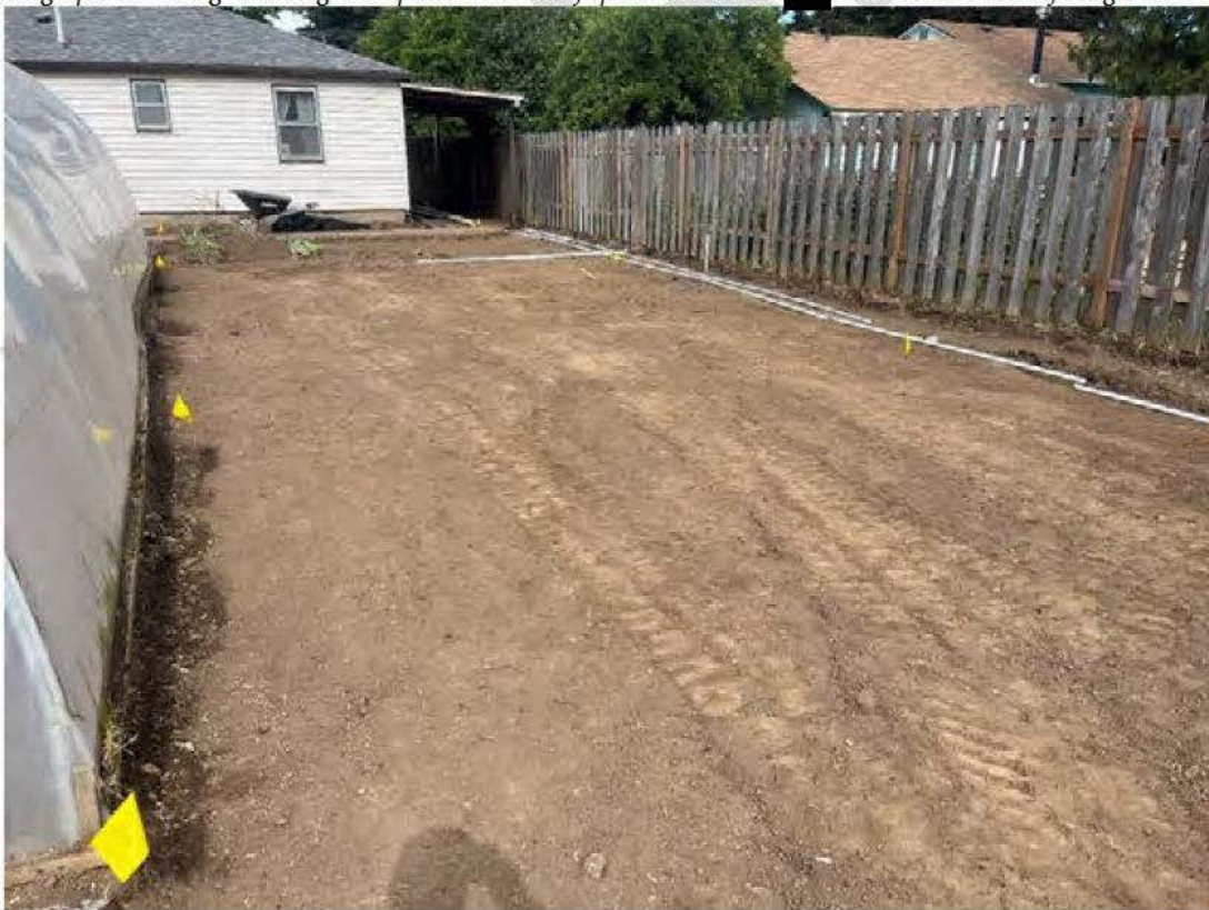
Photograph 10. 3 Kings marking anticipated locations of sprinkler heads at [REDACTED] Baxter. Photo taken facing northwest.
