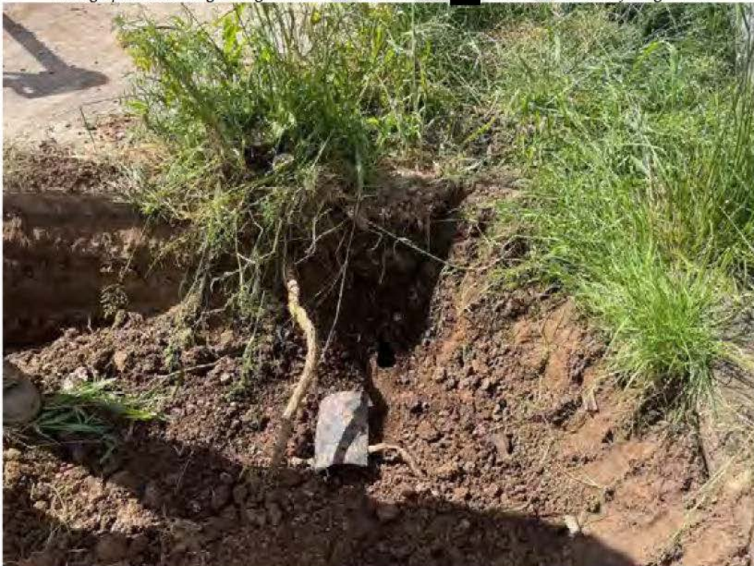
Photograph 14. Existing damaged sewer line encountered at [REDACTED] Baxter. Photo taken facing south.
