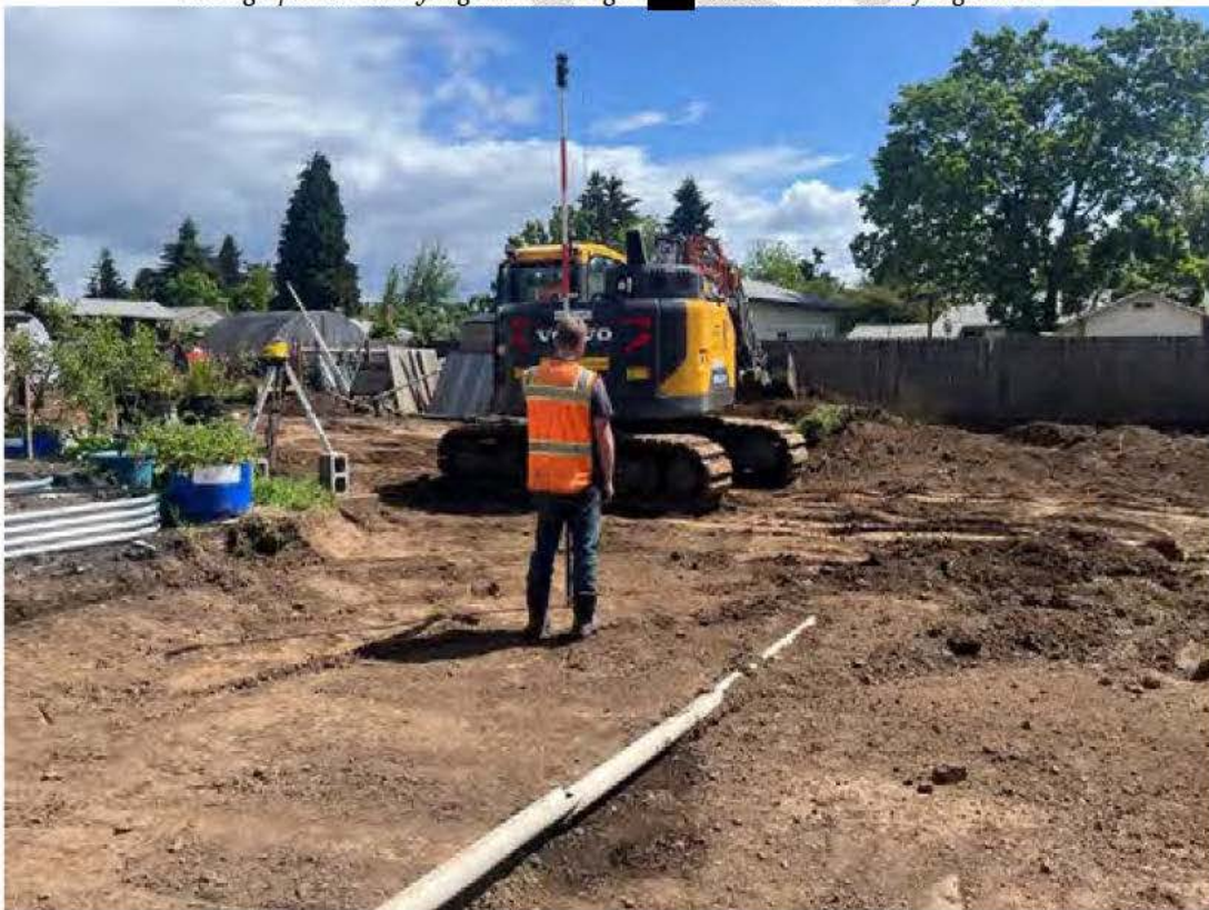
Photograph 15. Surveyor grade checking at [REDACTED] Baxter. Photo taken facign east.
