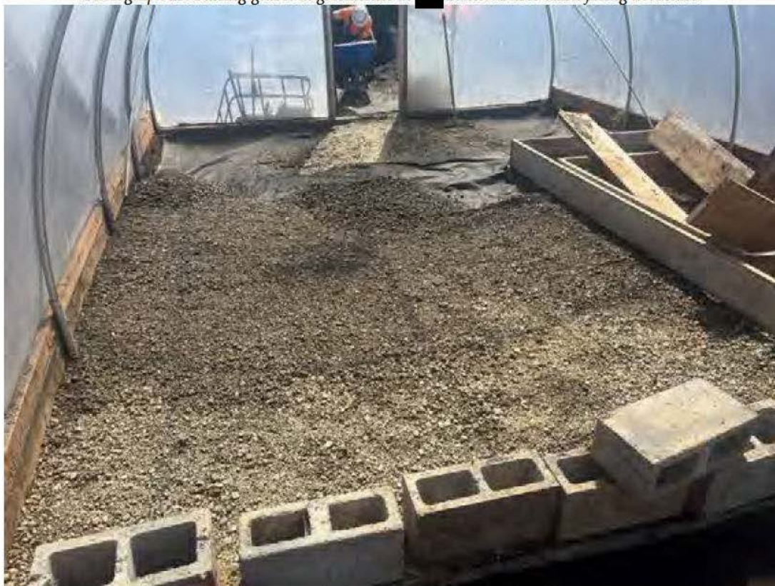
Photograph 14. Spot backfilling and improving mulch/gravel tie in at [REDACTED] Baxter. Photo taken facing southwest.
