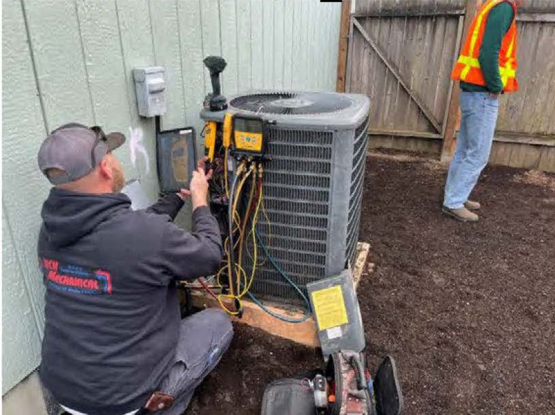
Photograph 1. Supplemental HVAC unit diagnosis at [REDACTED] Baxter. Photo taken facing south.
