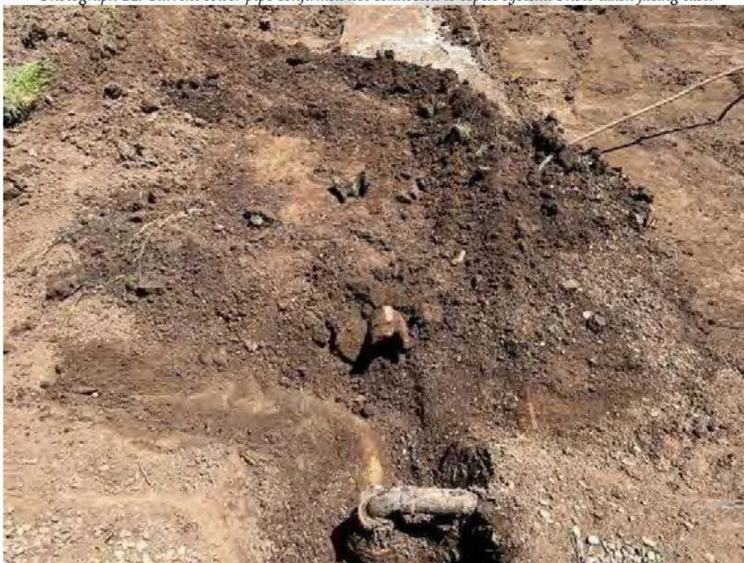
Photograph 14. Current sewer pipe confirmed not connected to septic system. Photo taken facing east.
