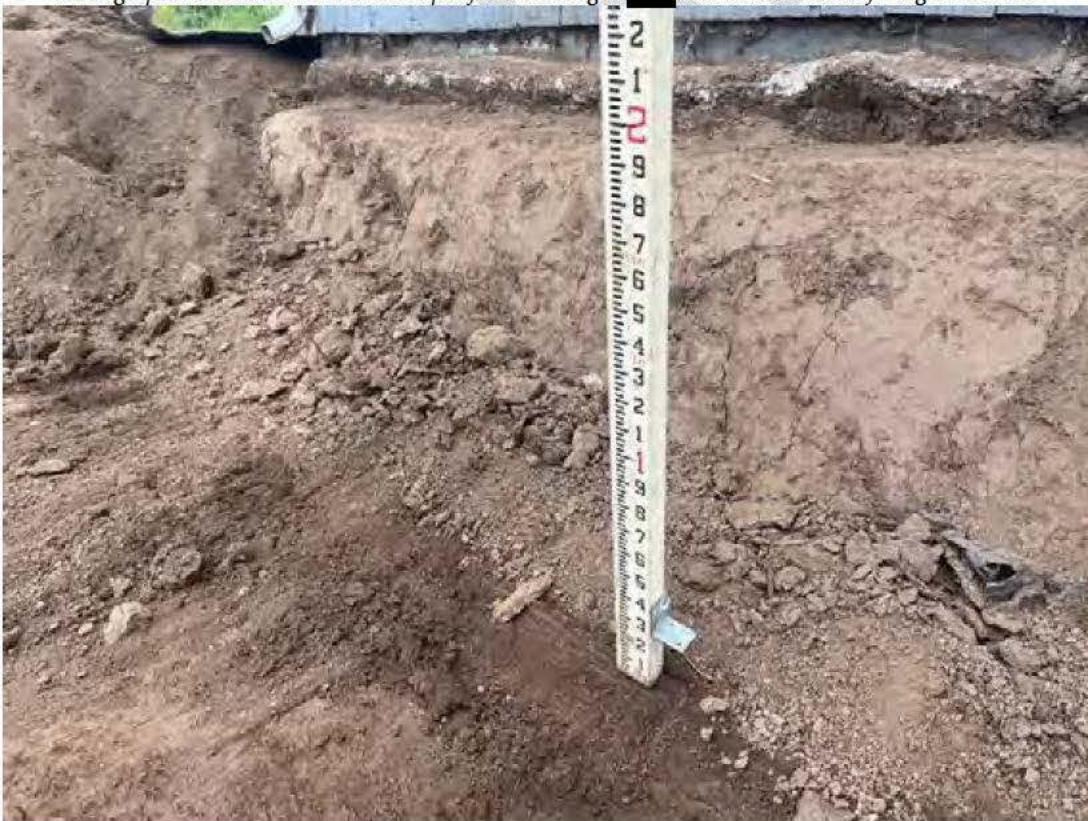
Photograph 10. Manual excavation depth field truthing at [REDACTED] Baxter. Photo taken facing southwest.
