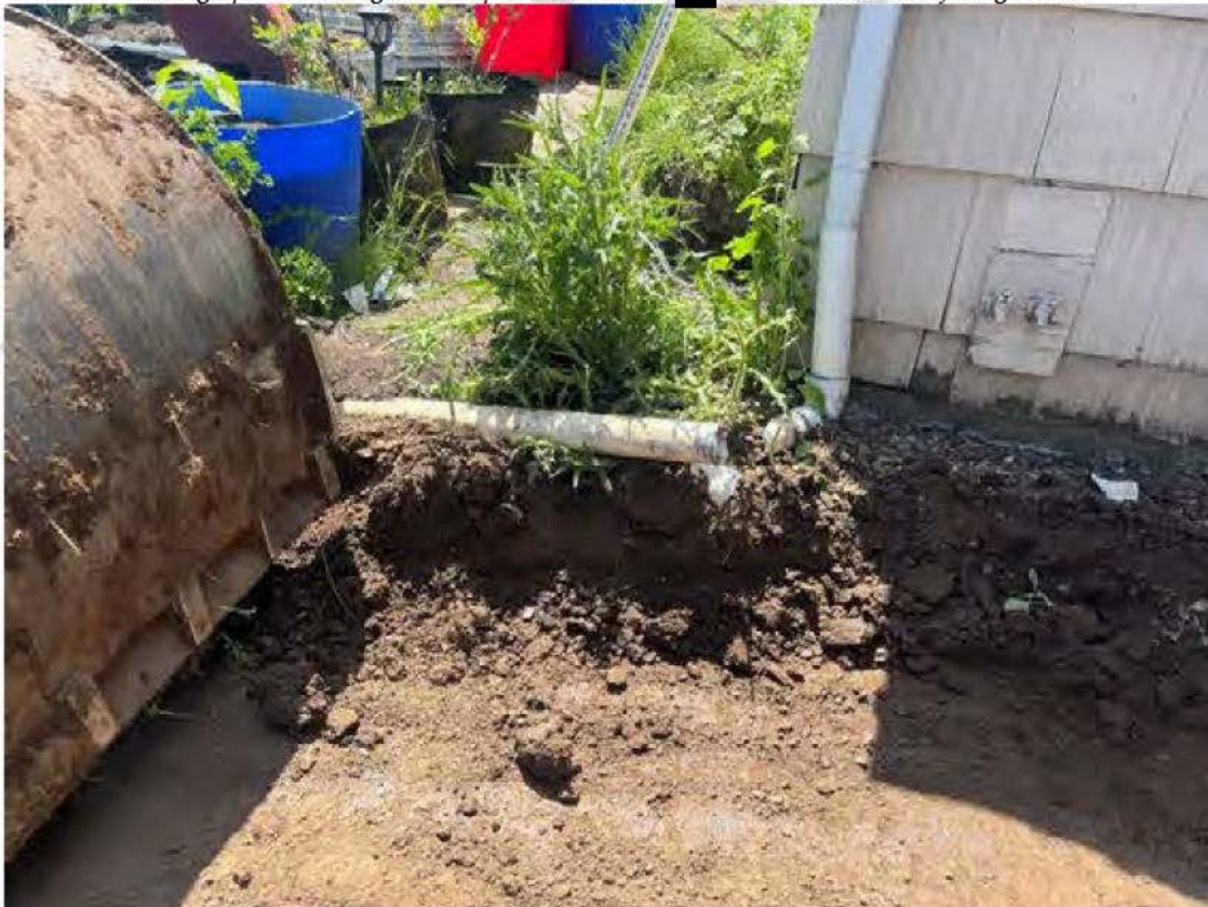
Photograph 10. Damaged downspout drain line at [REDACTED] Baxter. Photo taken facing south.
