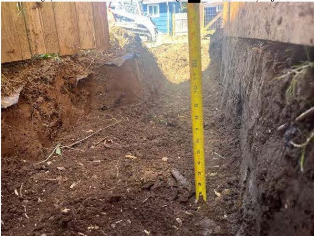
Photograph 13. Manual excavation depth field truthing at [REDACTED] Baxter. Photo taken facing west.
