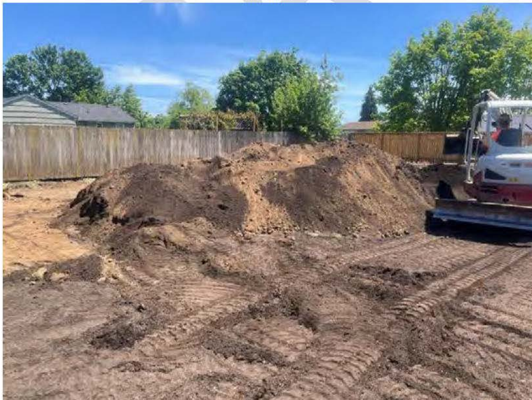
Photograph 20. Delta 'screened loam' product mixed with Rexius topsoil prior to final placing. Photo taken facing southeast.
