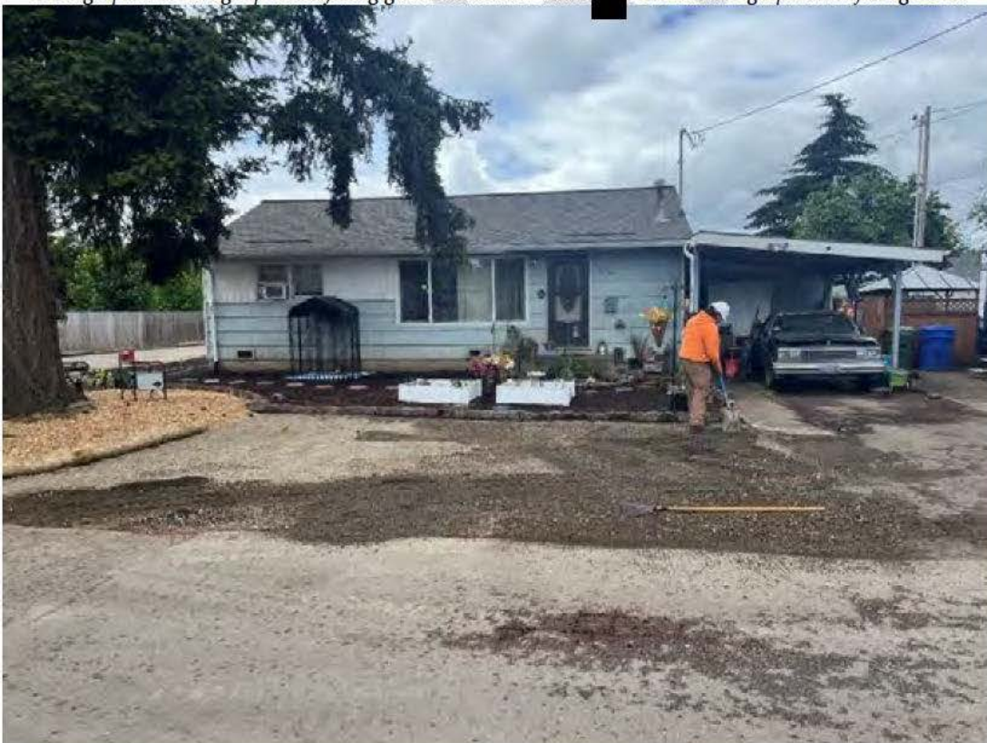
Photograph 18. 3 Kings spot backfilling gravel area in ROW at [REDACTED] Baxter. Photograph taken facing west.
