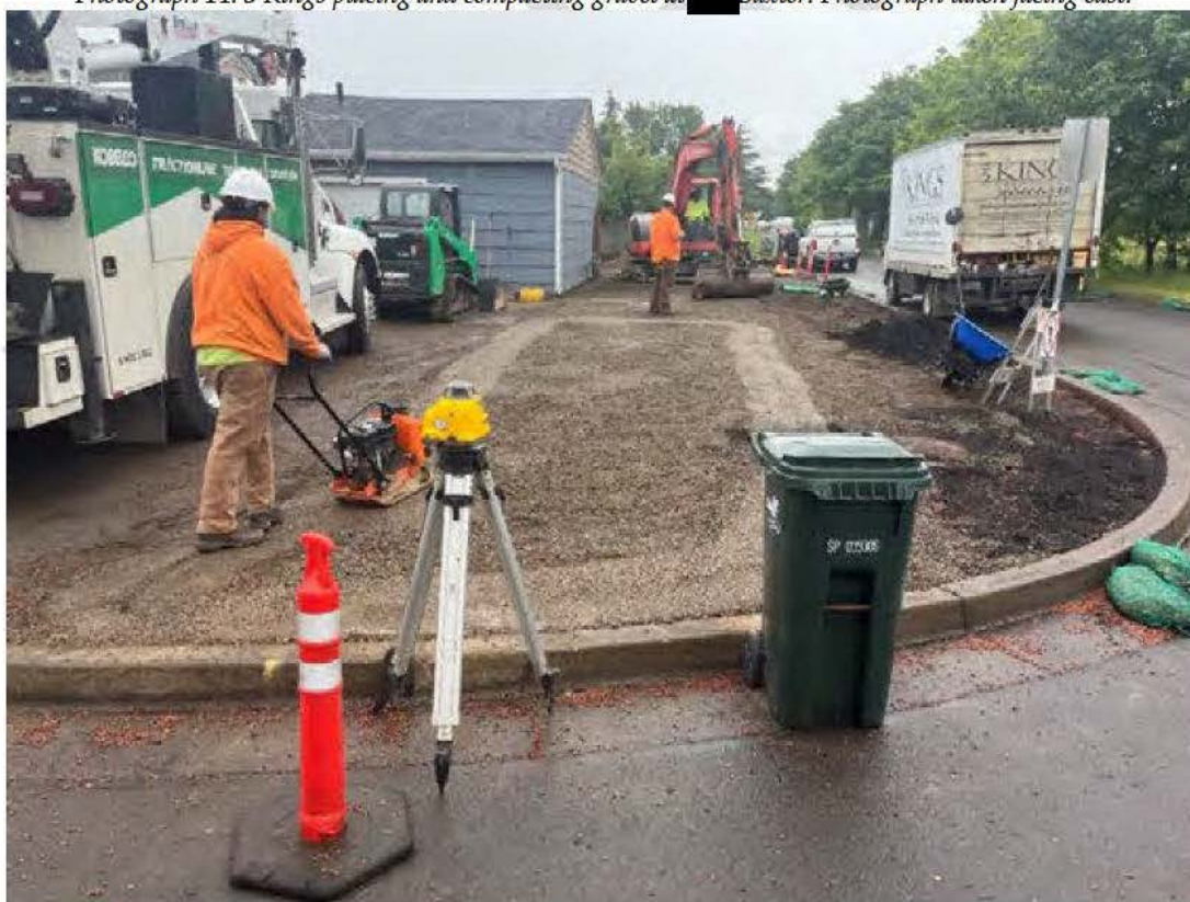
Photograph 14. 3 Kings placing and compacting gravel at [REDACTED] Baxter. Photograph taken facing east.
