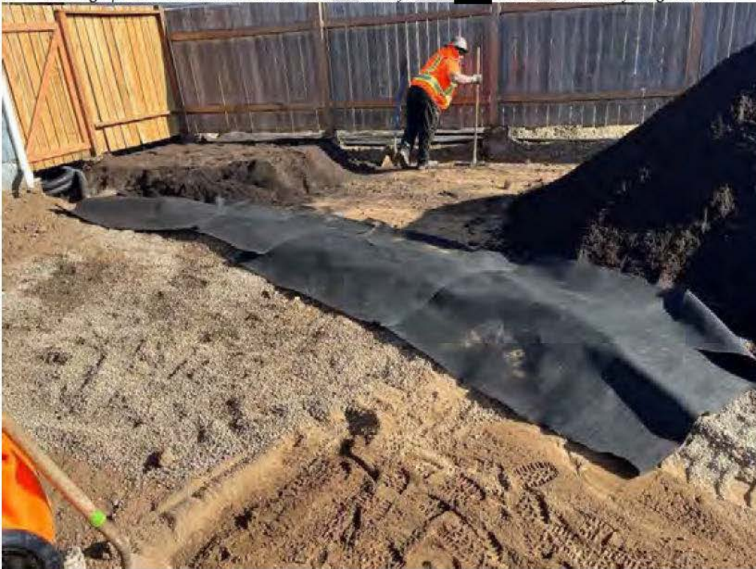
Photograph 8. Drain line covered with demarcation fabric at [REDACTED] Baxter. Photo taken facing north.
