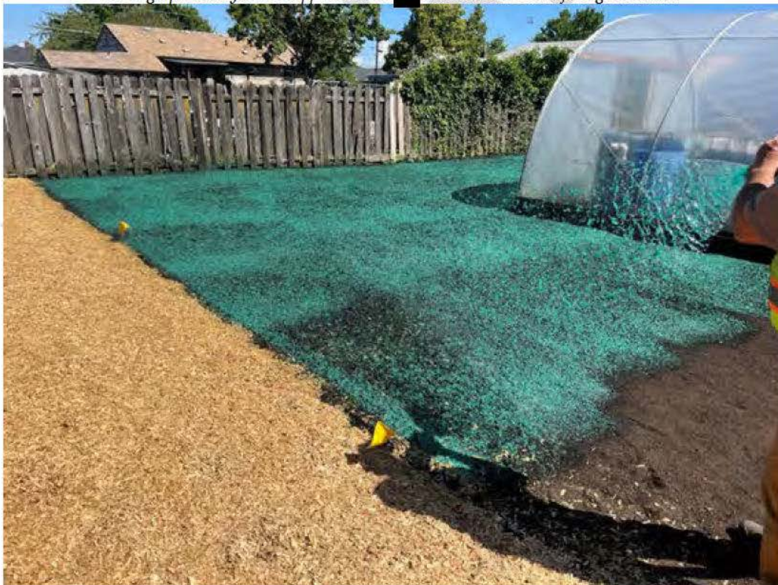
Photograph 25. Hydroseed application at [REDACTED] Baxter. Photo taken facing southeast.
