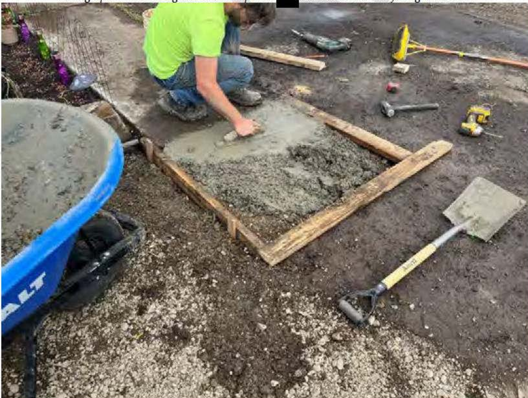
Photograph 12. Installing new concrete pad at [REDACTED] Baxter. Photo taken facing northwest.
