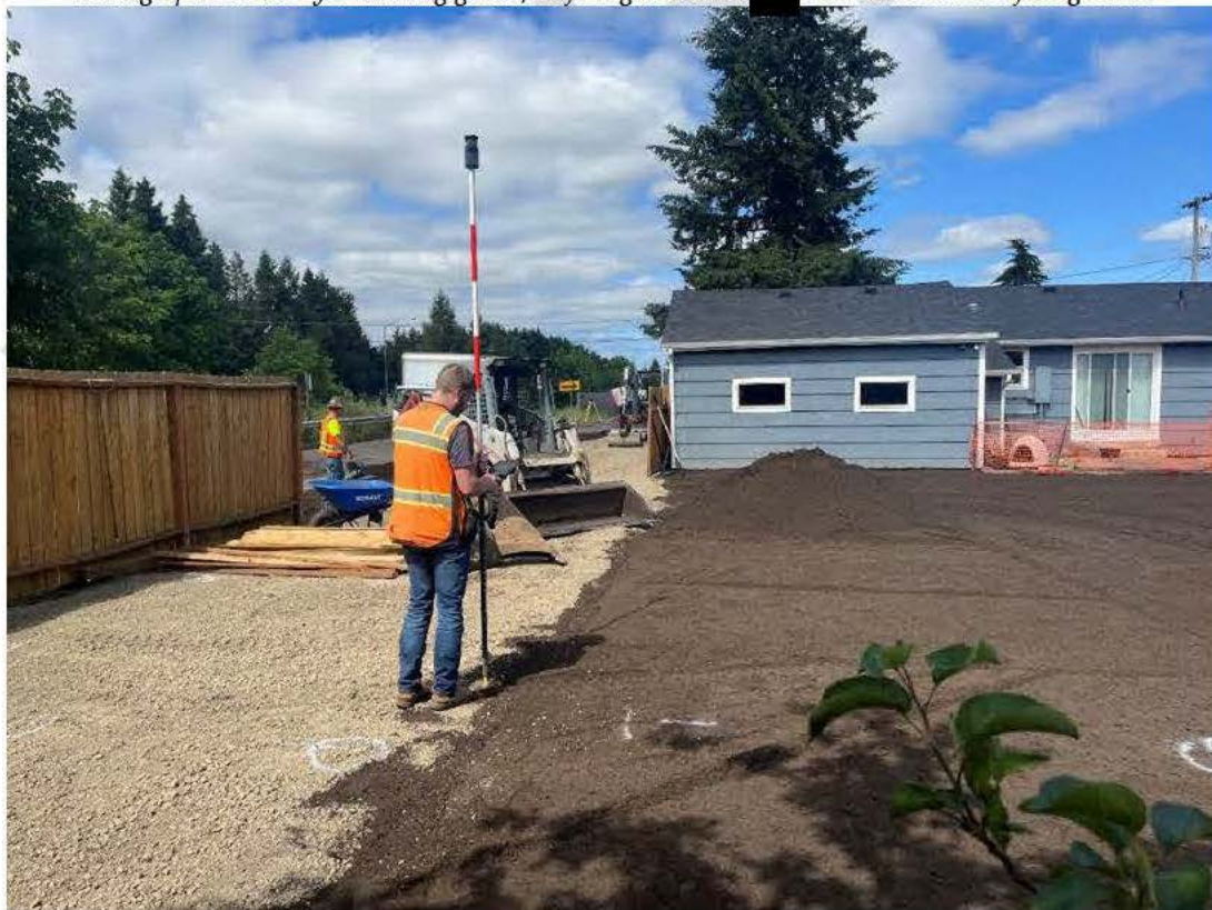
Photograph 10. Surveyor checking grades/surfacing extents at [REDACTED] Baxter. Photo taken facing west.
