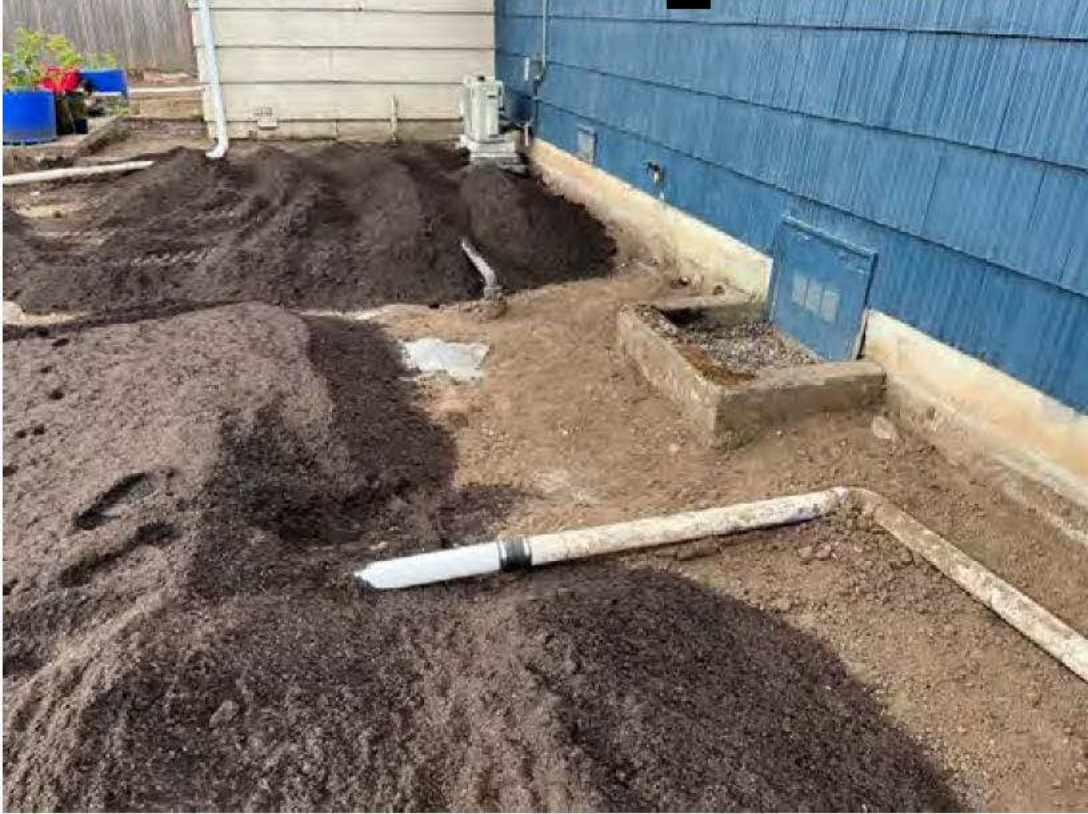
Photograph 4. Backfill placement around repaired utility features at [REDACTED] Baxter. Photograph taken facing south.
