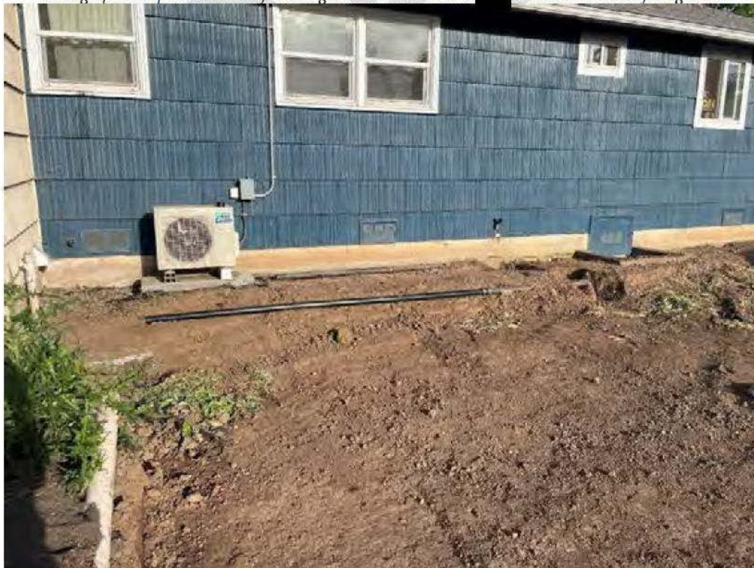
Photograph 2. Repaired section of washing machine drain line at [REDACTED] Baxter. Photo taken facing west.
