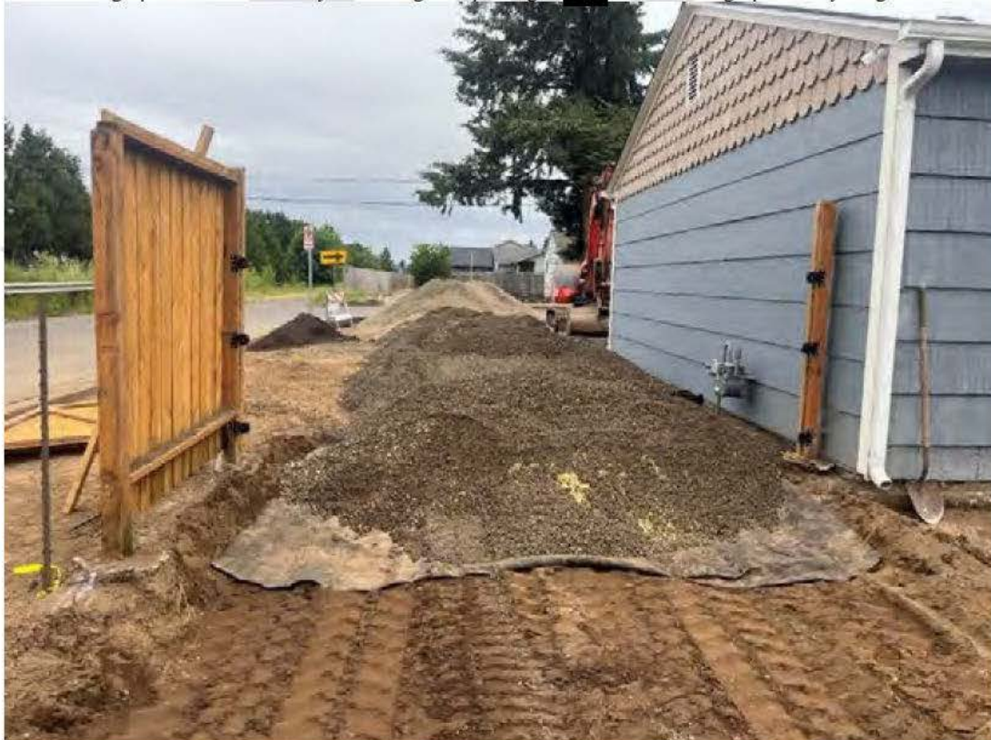
Photograph 11. Demarcation fabric and gravel placing at [REDACTED] Baxter. Photograph taken facing west.
