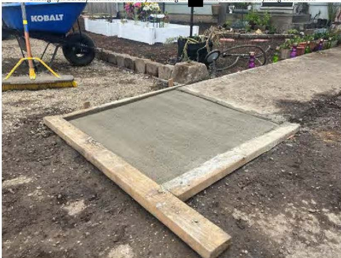
Photograph 14. Replacement concrete pad curing at [REDACTED] Baxter. Photo taken facing southwest.
