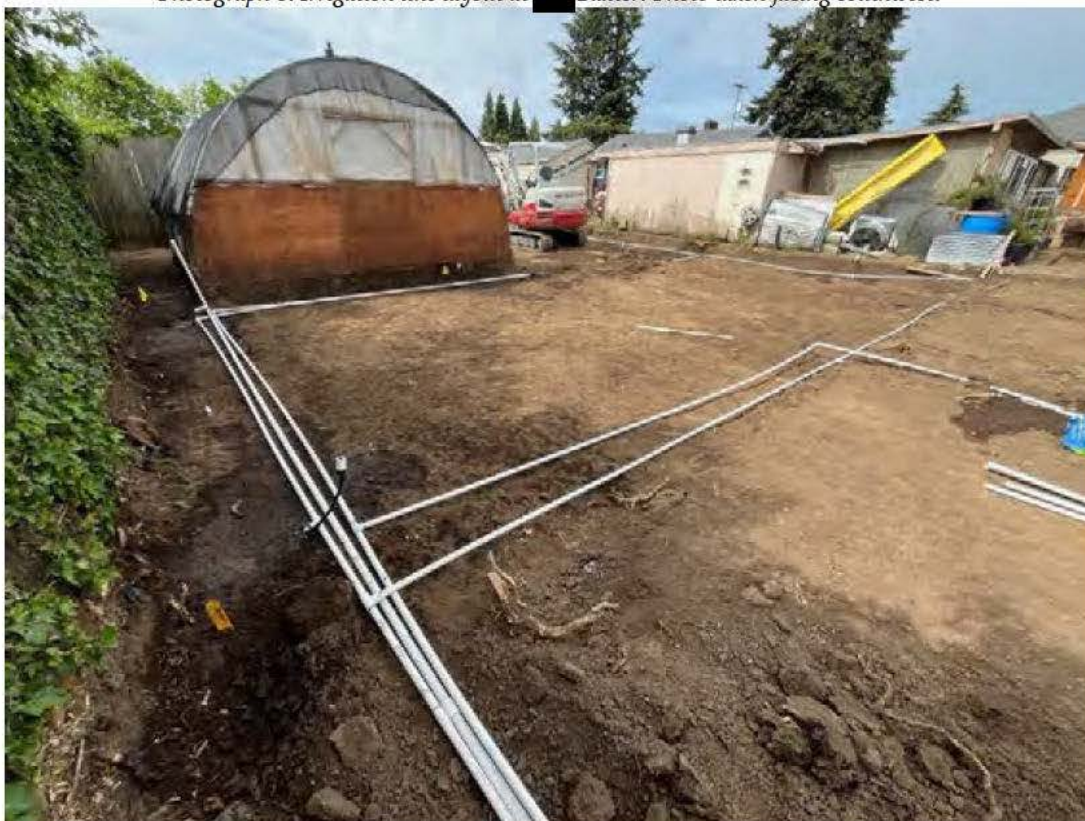
Photograph 8. Irrigation line layout at [REDACTED] Baxter. Photo taken facing southwest.
