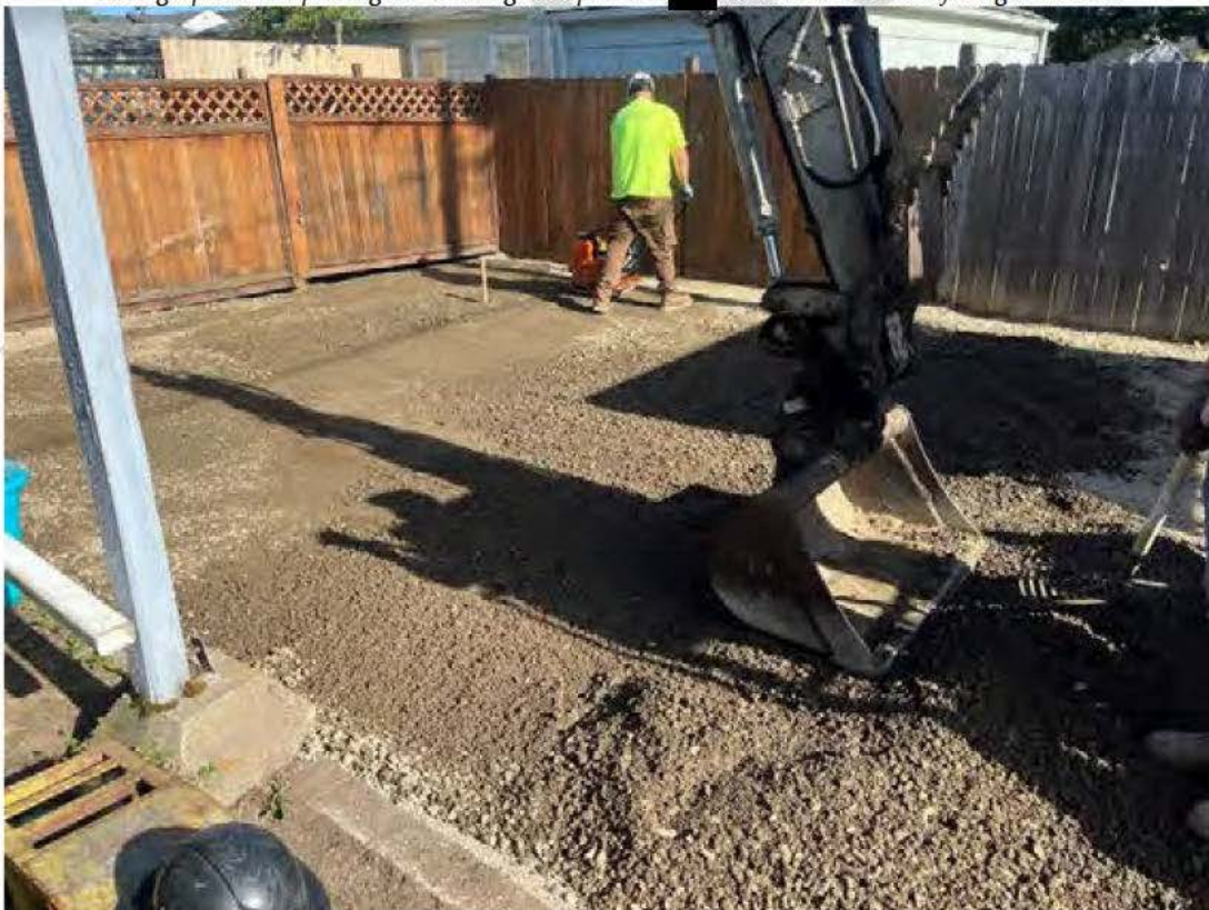
Photograph 4. Compacting additional gravel placed at [REDACTED] Baxter. Photo taken facing northeast.
