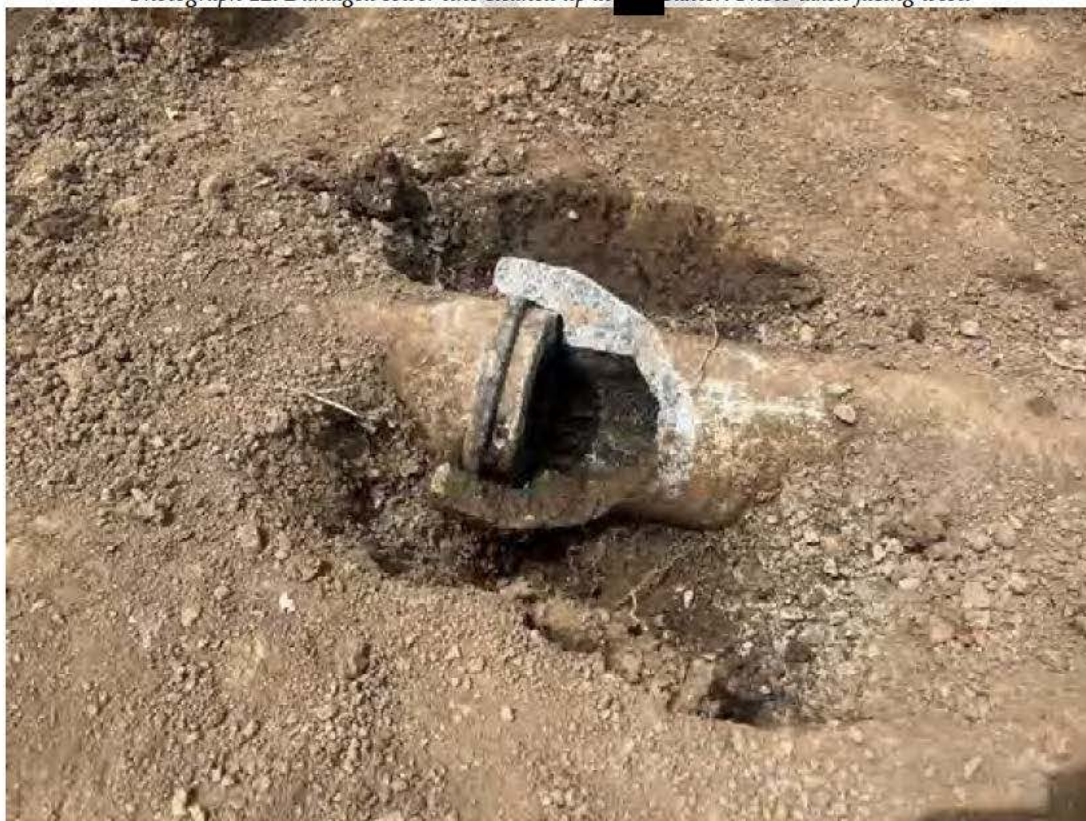
Photograph 12. Damaged sewer line cleaned up at [REDACTED] Baxter. Photo taken facing west.
