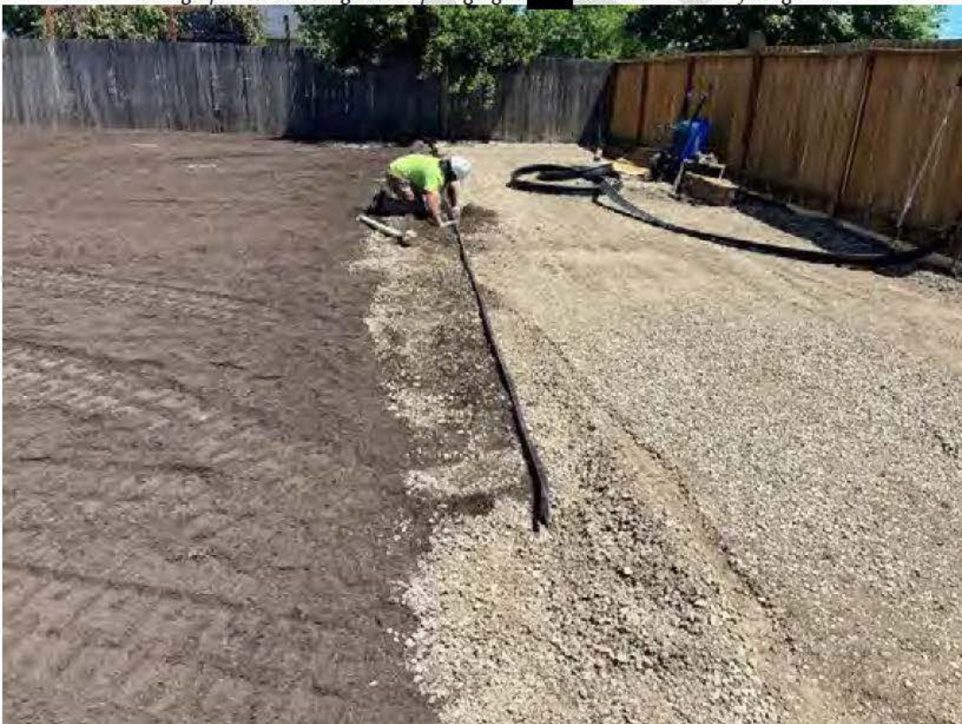
Photograph 18. Installing landscape edging at [REDACTED] Baxter. Photo taken facing east.
