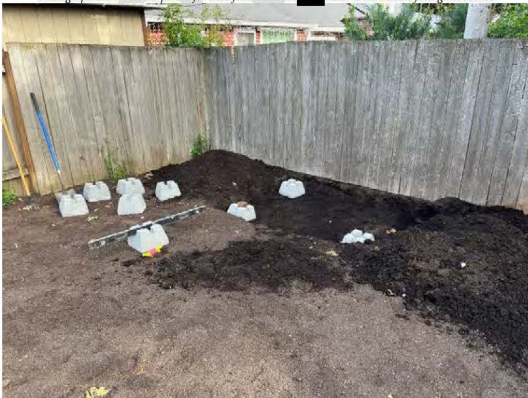
Photograph 2. Pier blocks placed for shed foundation at [REDACTED] Baxter. Photo taken facing northwest.
