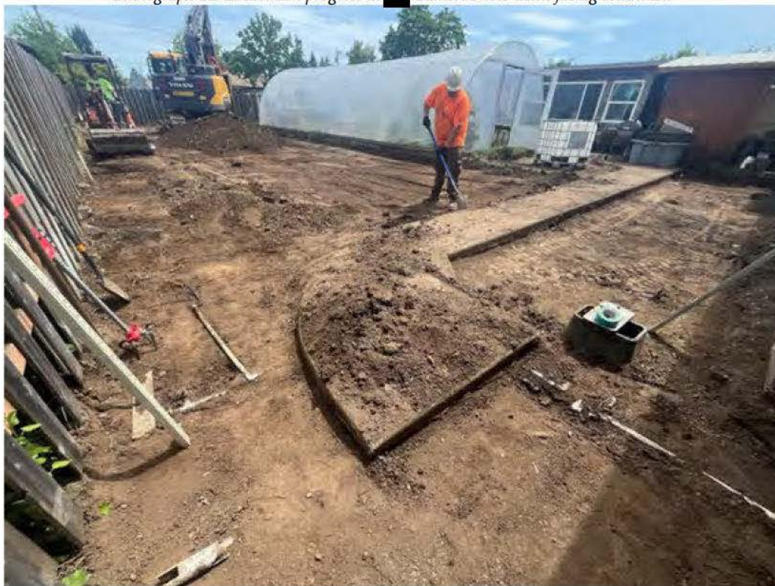
Photograph 15. Demarcation fabric and gravel placed at [REDACTED] Baxter. Photo taken facing southeast.
