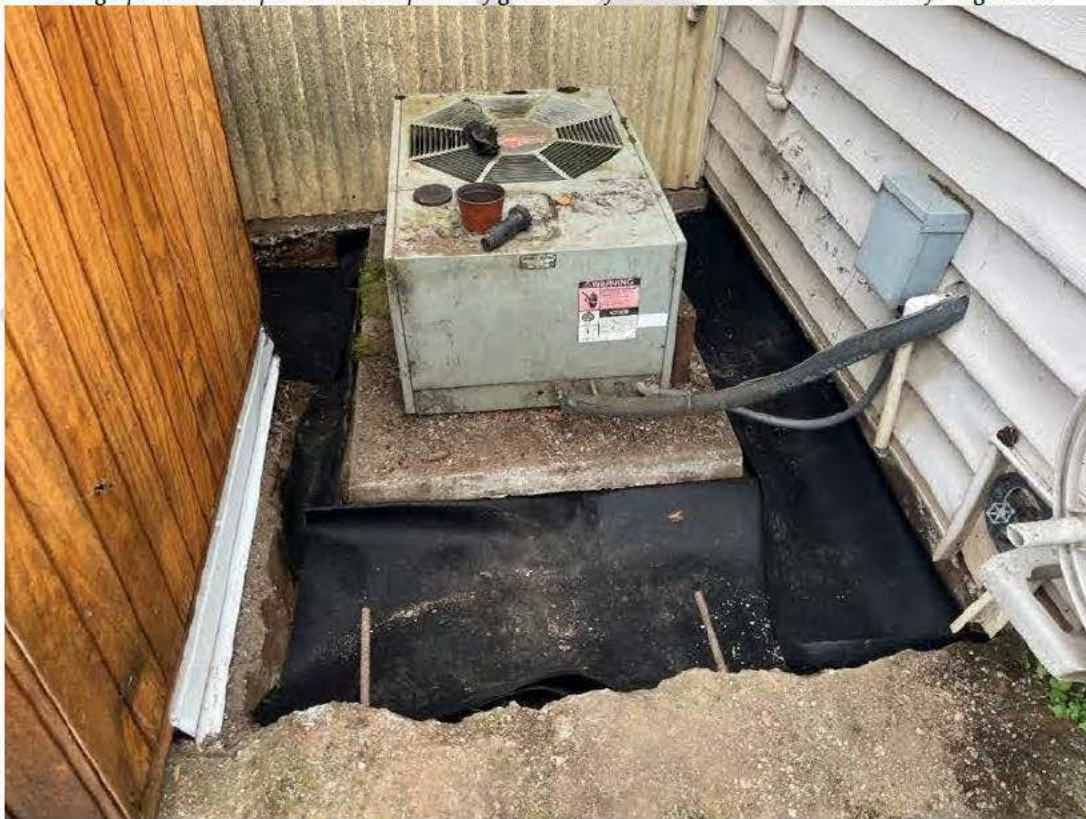
Photograph 12. Fabric placed in anticipation of gravel backfill around AC unit. Photo taken facing south.
