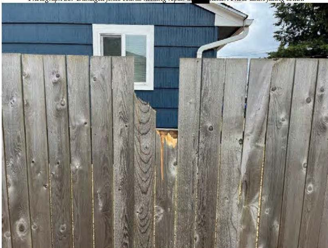
Photograph 26. Damaged fence boards needing repair at [REDACTED] Baxter. Photo taken facing south.
