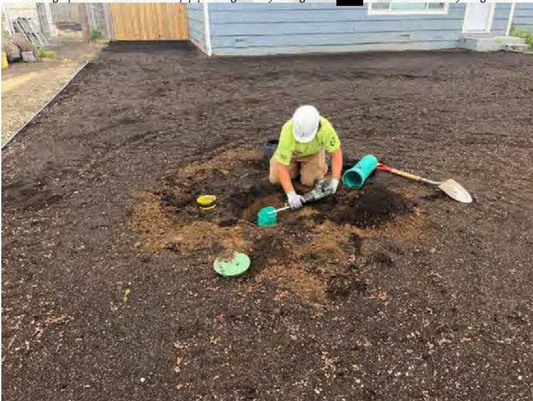
Photograph 10. Cleanout stub up pipe being cut to finish grade at [REDACTED] Baxter. Photo taken facing east.
