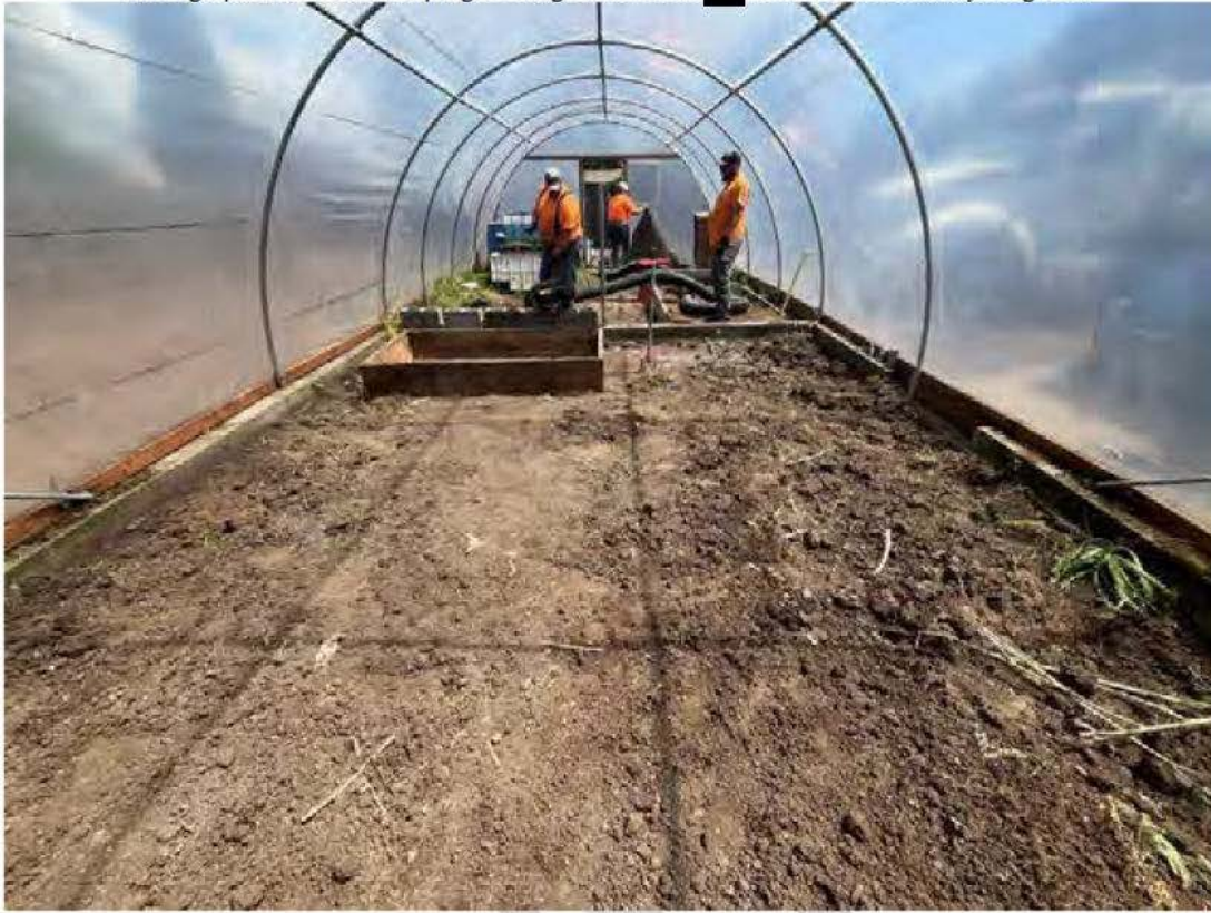
Photograph 23. Follow up grading based on surveyor marks. Photo taken facing south.
