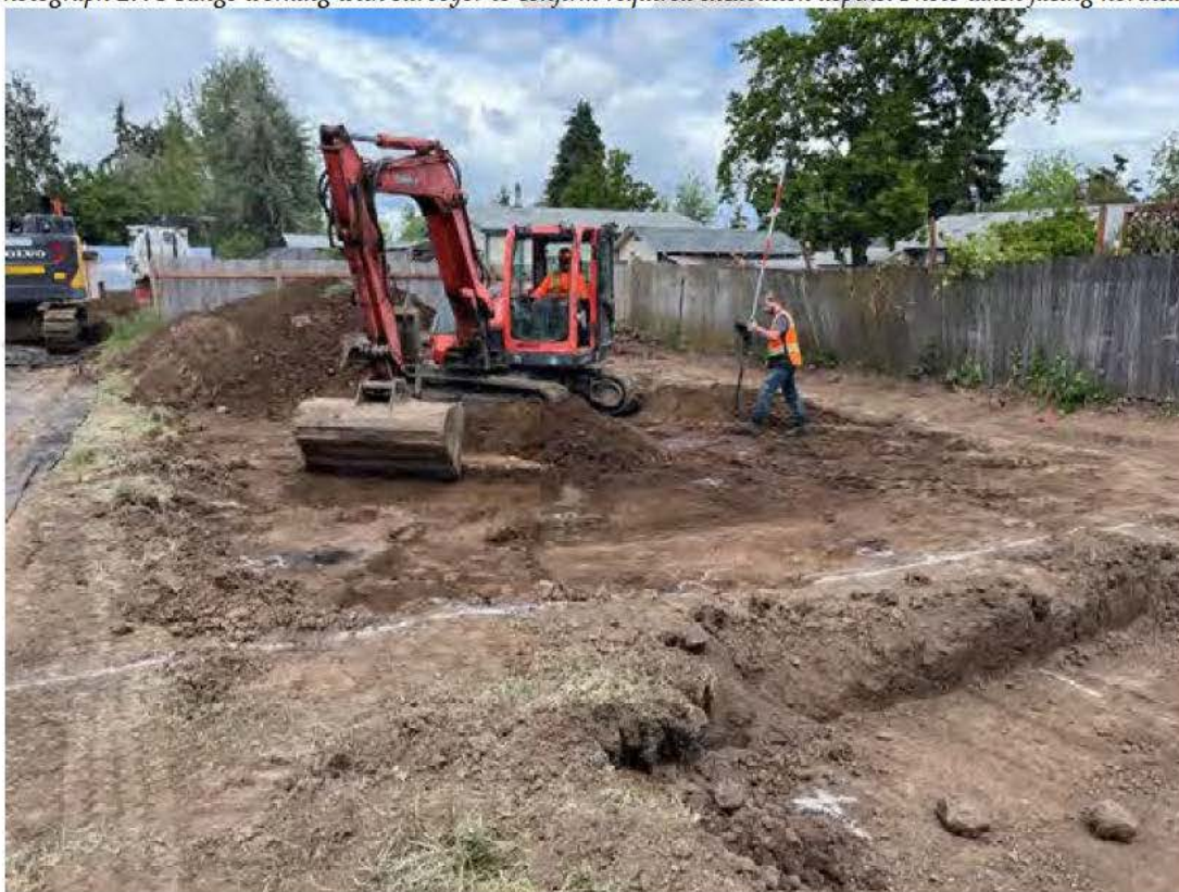
Photograph 27. 3 Kings working with surveyor to confirm required excavation depths. Photo taken facing northeast.
