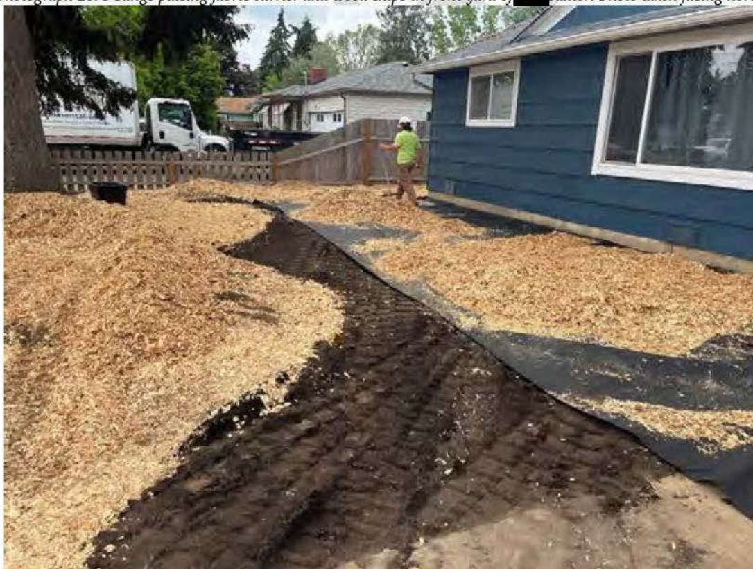
Photograph 20. 3 Kings placing fabric barrier and wood chips in front yard of [REDACTED] Baxter. Photo taken facing north.
