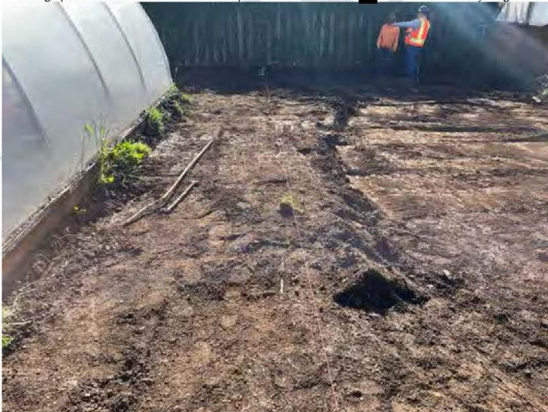
Photograph 3. 6 inch to 12 inch excavation depth transition marked at [REDACTED] Baxter. Photo taken facing east.
