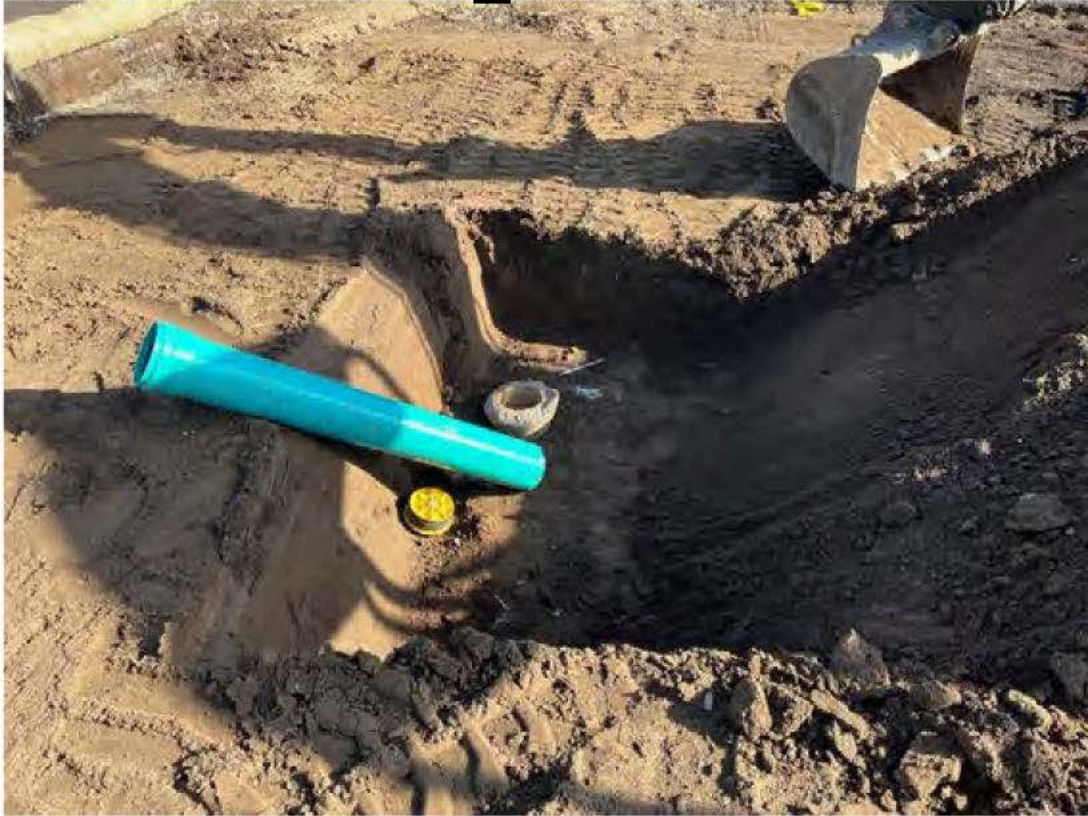
Photograph 3. 6 inch to 12 inch excavation depth transition marked at [REDACTED] Baxter. Photo taken facing east.
