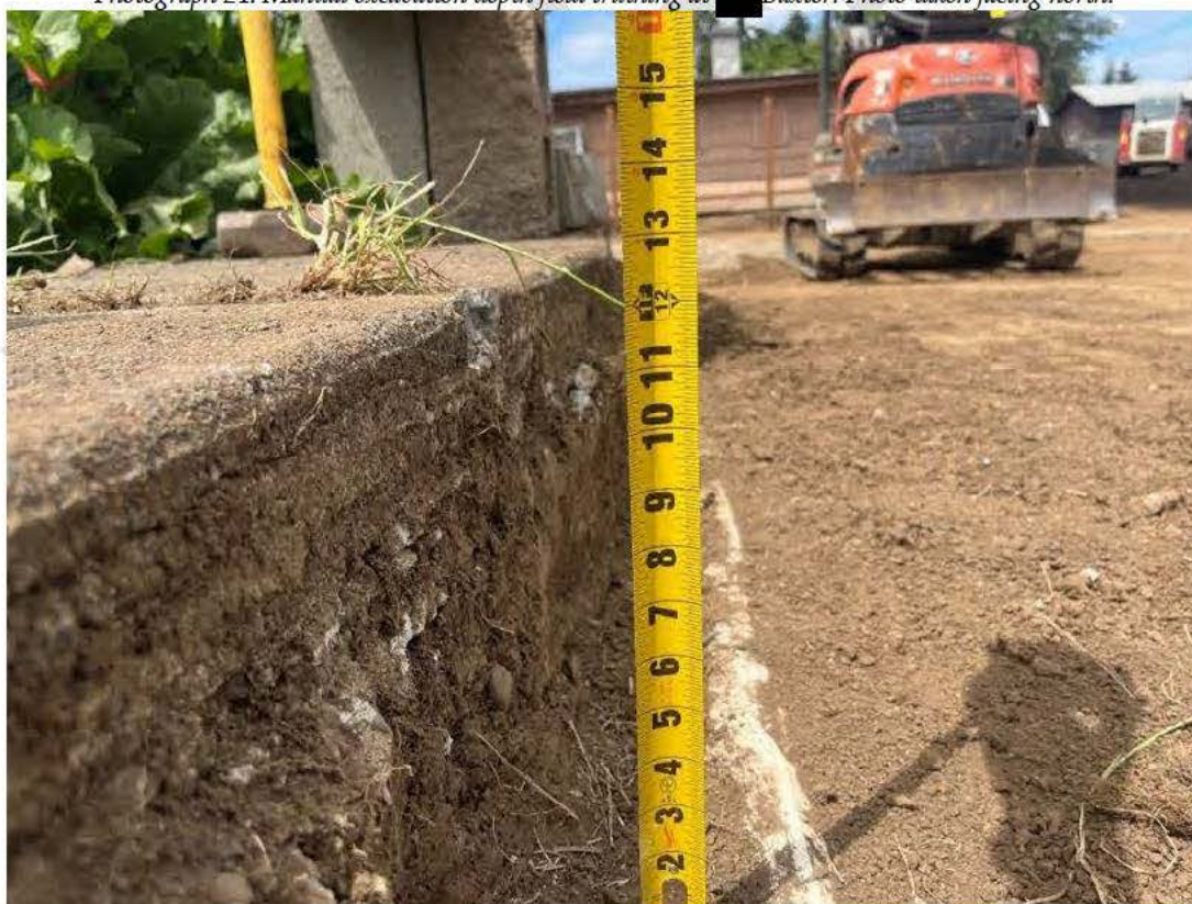
Photograph 24. Manual excavation depth field truthing at [REDACTED] Baxter. Photo taken facing north.
