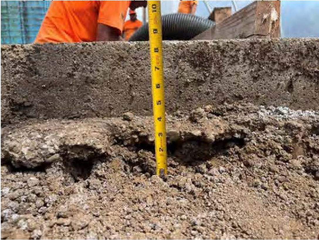
Photograph 31. Manual excavation depth field truthing in greenhouse. Photo taken facing south.
