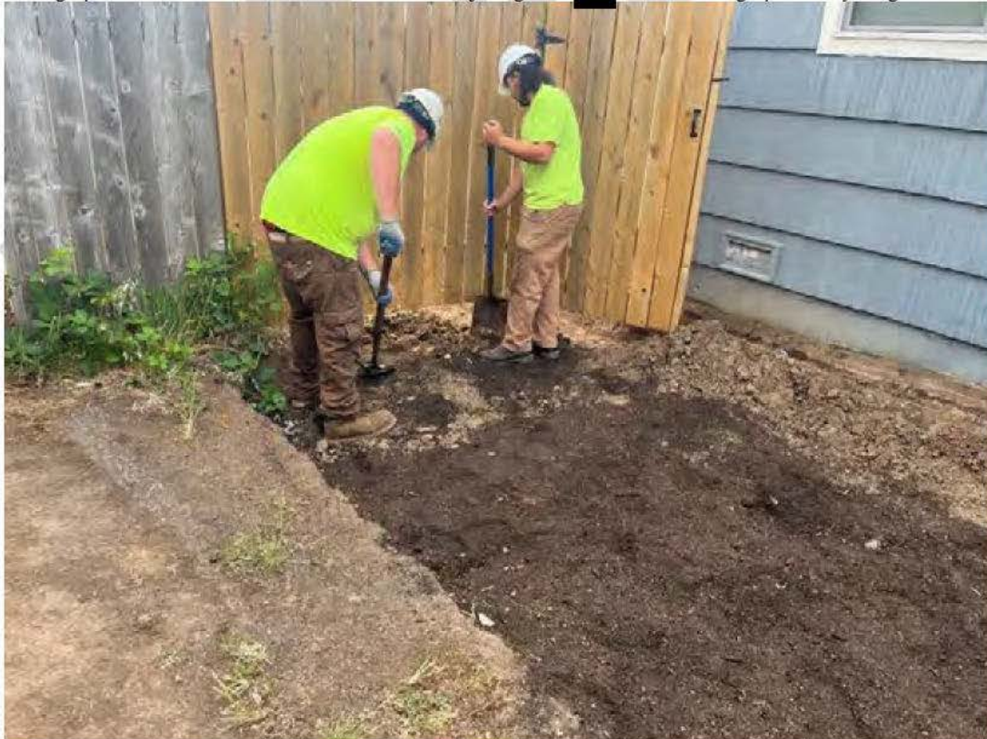
Photograph 3. Hand tool removal beneath north side yard gate at [REDACTED] Baxter. Photograph taken facing southeast.
