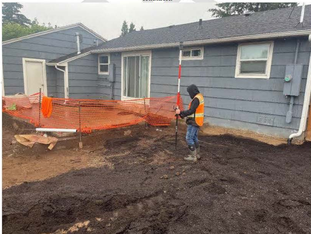
Photograph 12. Surveyor checking excavation grade to north of back porch at [REDACTED] Baxter. Photograph taken facing southwest.
