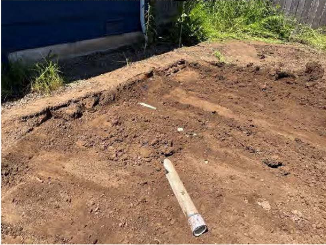
Photograph 16. Trench digging in imported soil for irrigation line install. Photo taken facing south.
