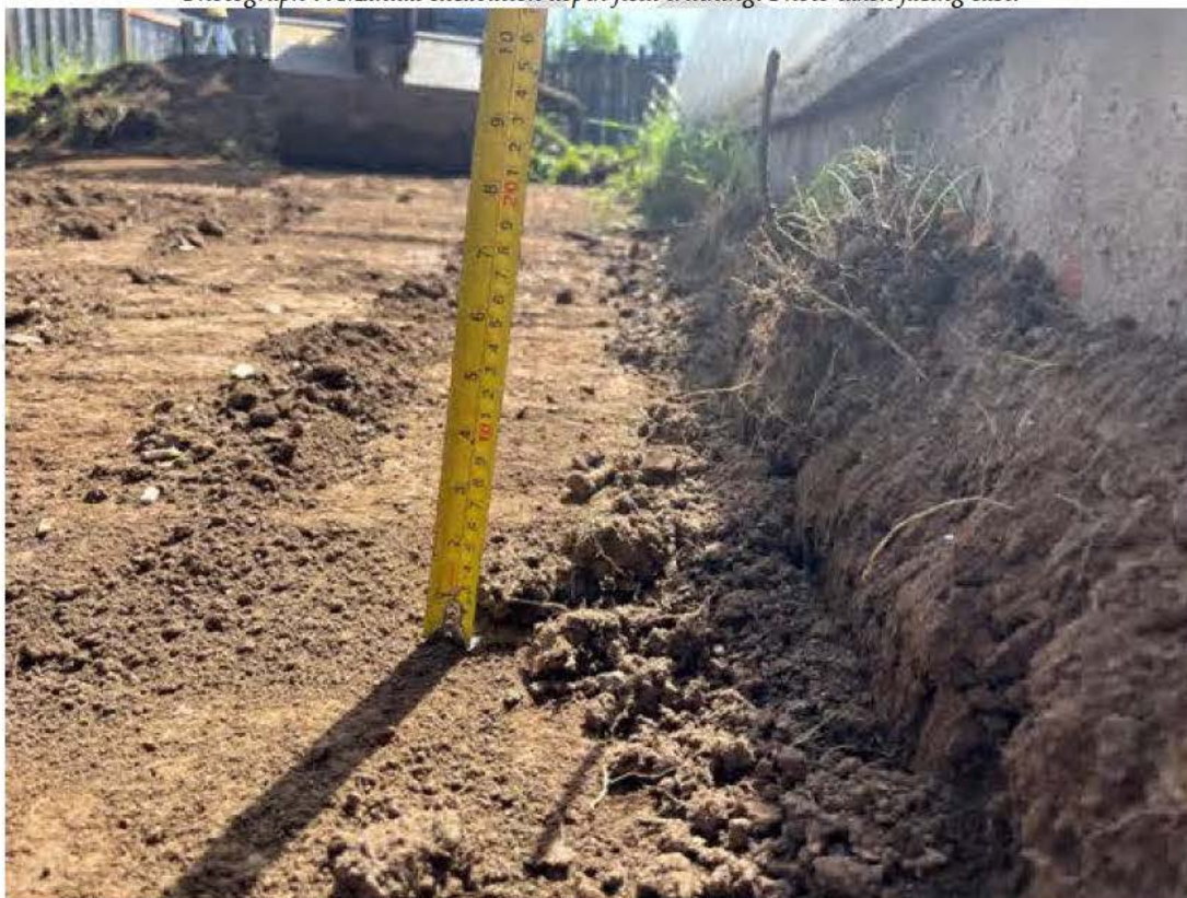
Photograph 7. Manual excavation depth field truthing. Photo taken facing east.
