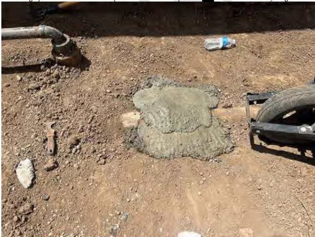
Photograph 20. Additional concrete poured over sewer line patch at [REDACTED] Baxter. Photo taken facing west.
