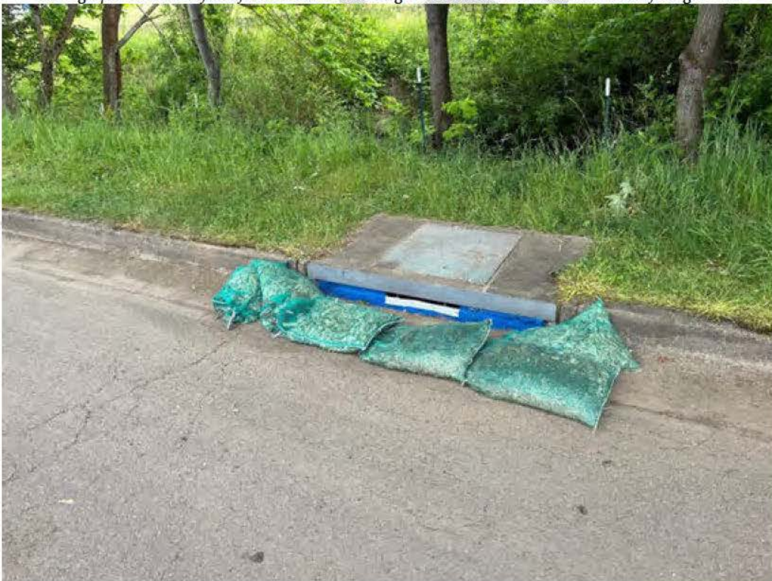
Photograph 19. BMP refresh for side road connecting Baxter and Alva Park. Photo taken facing south.
