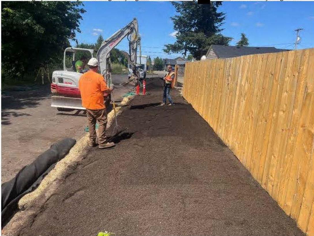
Photograph 12. Surveyor checking backfill grades in ROW along [REDACTED] Baxter. Photo taken facing west.
