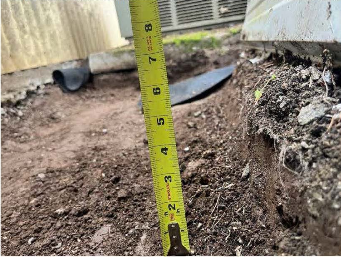
Photograph 12. Fabric placed in anticipation of gravel backfill around AC unit. Photo taken facing south.
