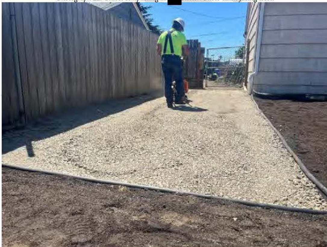
Photograph 22. Gravel compacting at [REDACTED] Baxter. Photo taken facing west.
