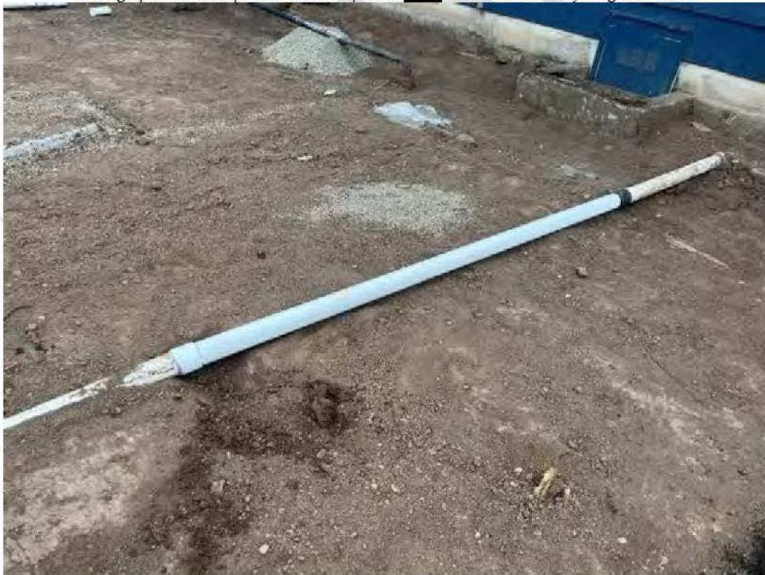
Photograph 16. Downspout drain line repairs at [REDACTED] Baxter. Photo taken facing southwest.
