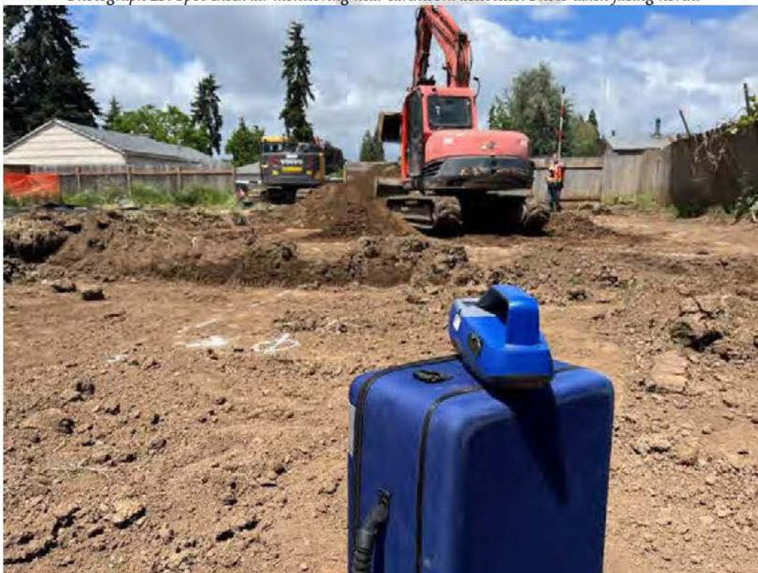
Photograph 25. Spot check air monitoring near earthwork activities. Photo taken facing north.
