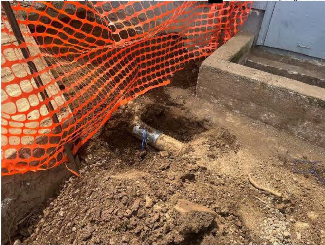
Photograph 22. Existing damaged sewer line with temp cover installed at [REDACTED] Baxter. Photo taken facing southwest.
