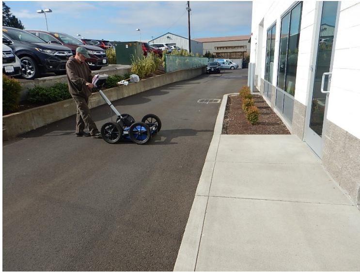
Scanning TL2200 using Ground Penetrating Radar equipment.
