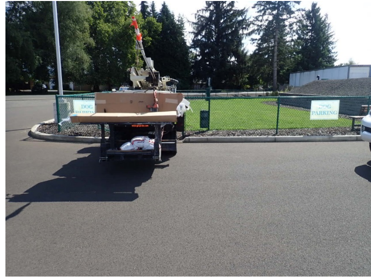
Drilling equipment was steam cleaned between borings to prevent cross-contamination.
