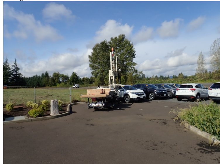
Drilling near the former Evaporation Pond (boring B04).
