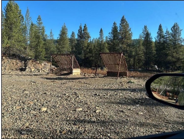
Figure 12. Tailings Area-01, Grizzly Feeders, October 7, 2025, facing Northeast, approximately 150 yards west of Clear Creek, DEQ
