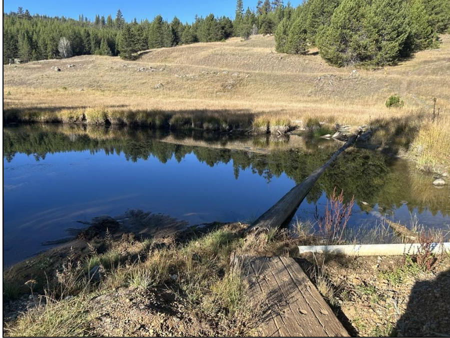
Figure 13. Discharge Point-01, Pond and piping, October 7, 2025, facing west approximately 220 yards west of Clear Creek and 260 yards southwest of Granite Creek, DEQ
