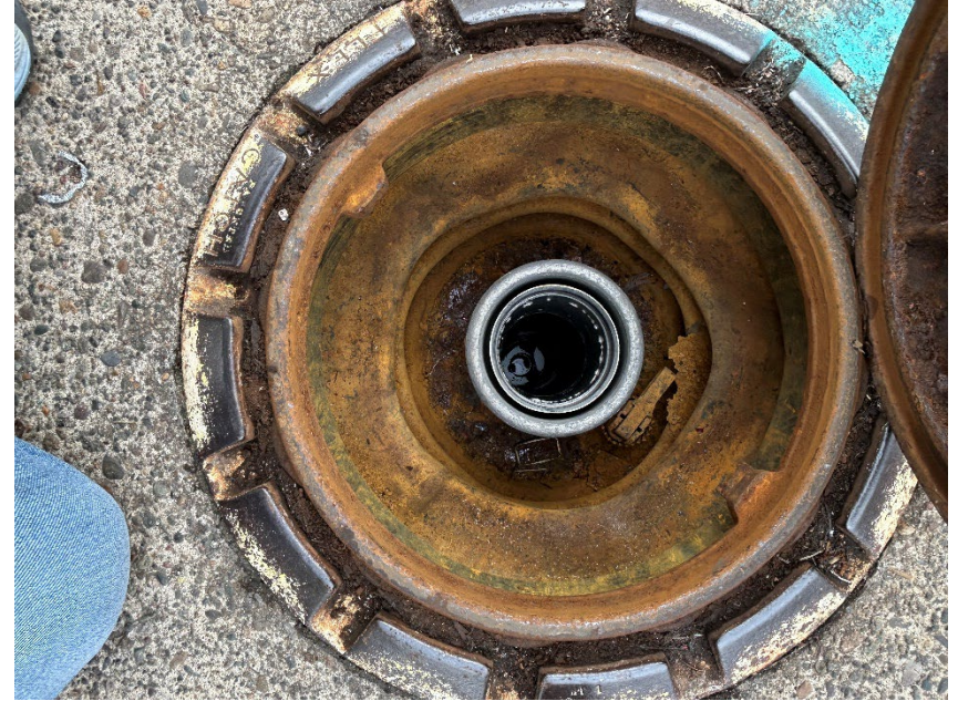
8: Regular fill with coaxil drop tube
