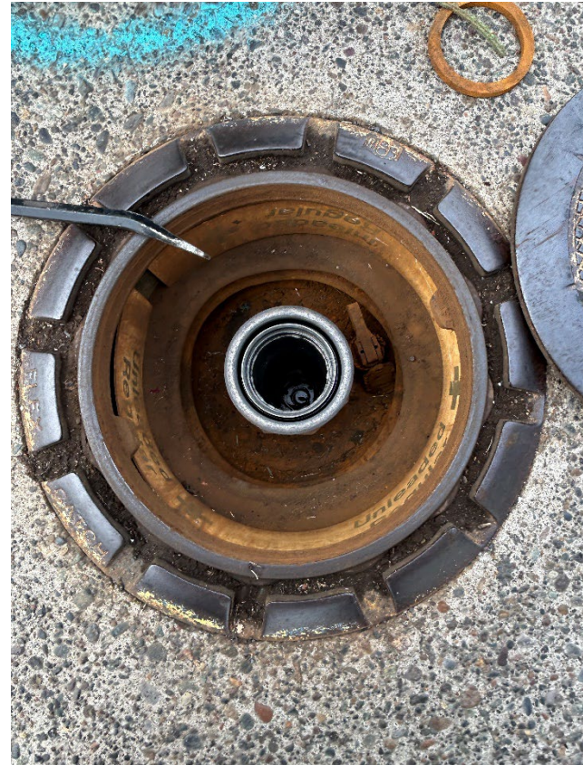
10: Regular fill with coaxial drop tube
