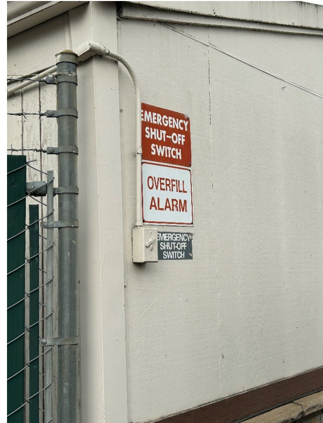
16: Emergency shut-off and overfill alarm
