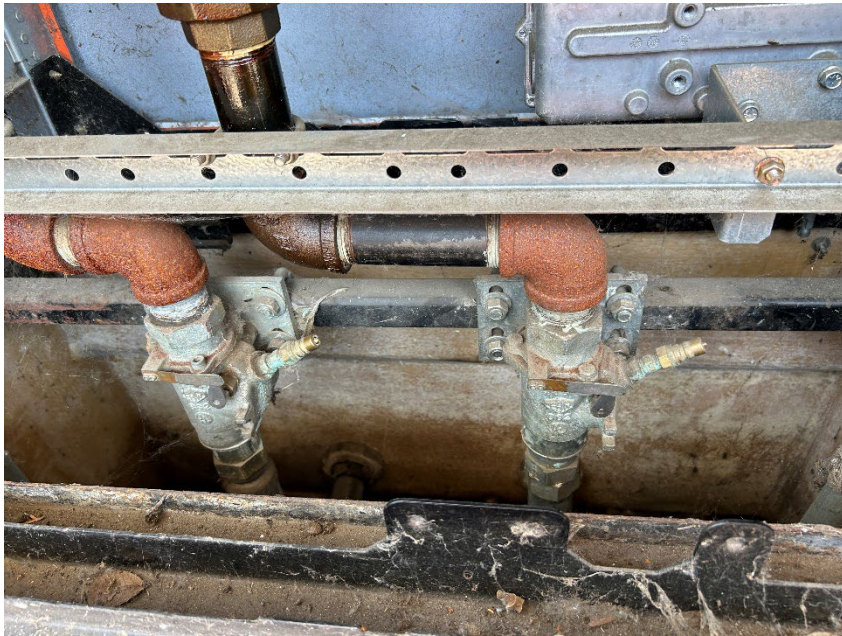
Disp 1/2 test ports on shear valves
