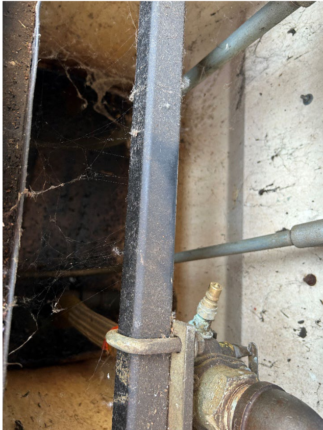
Diesel UDC test port on shear valve
