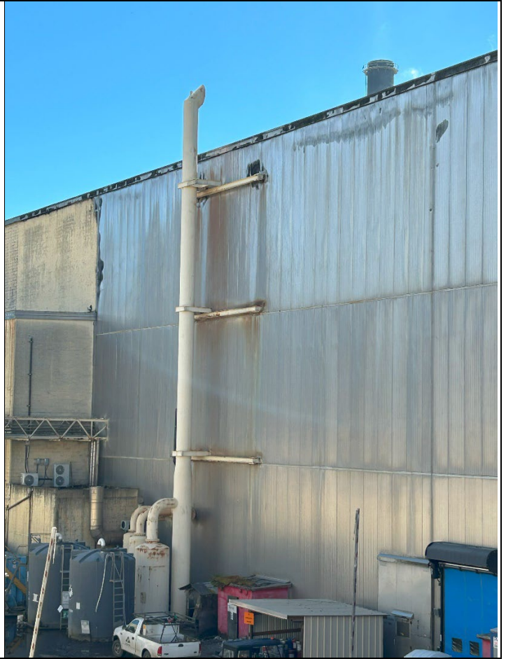
Photo 2: Vent for the vacuum pump at the paper machine area.
