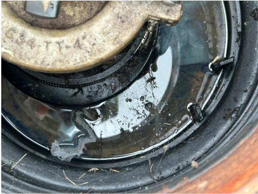
15: Unused fill into gasoline UST
