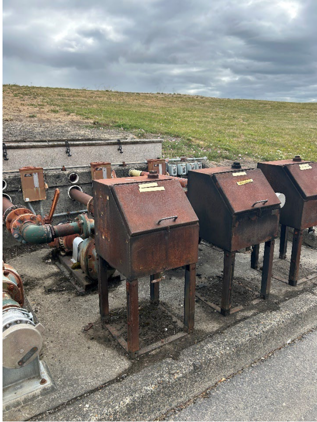
1: 7111 NE Alderwood Dr, Portland, OR 97217 Above ground fills
