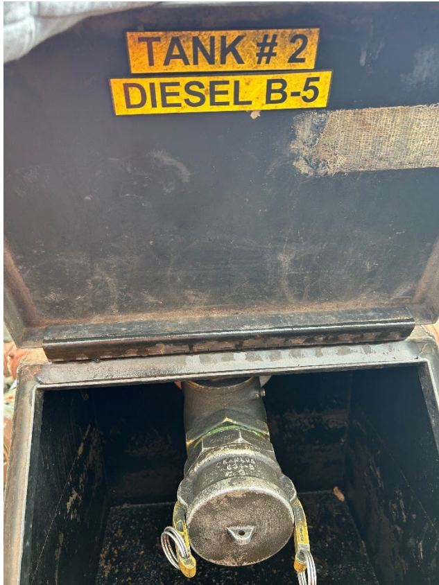
3: Above ground fill for B-5 diesel
