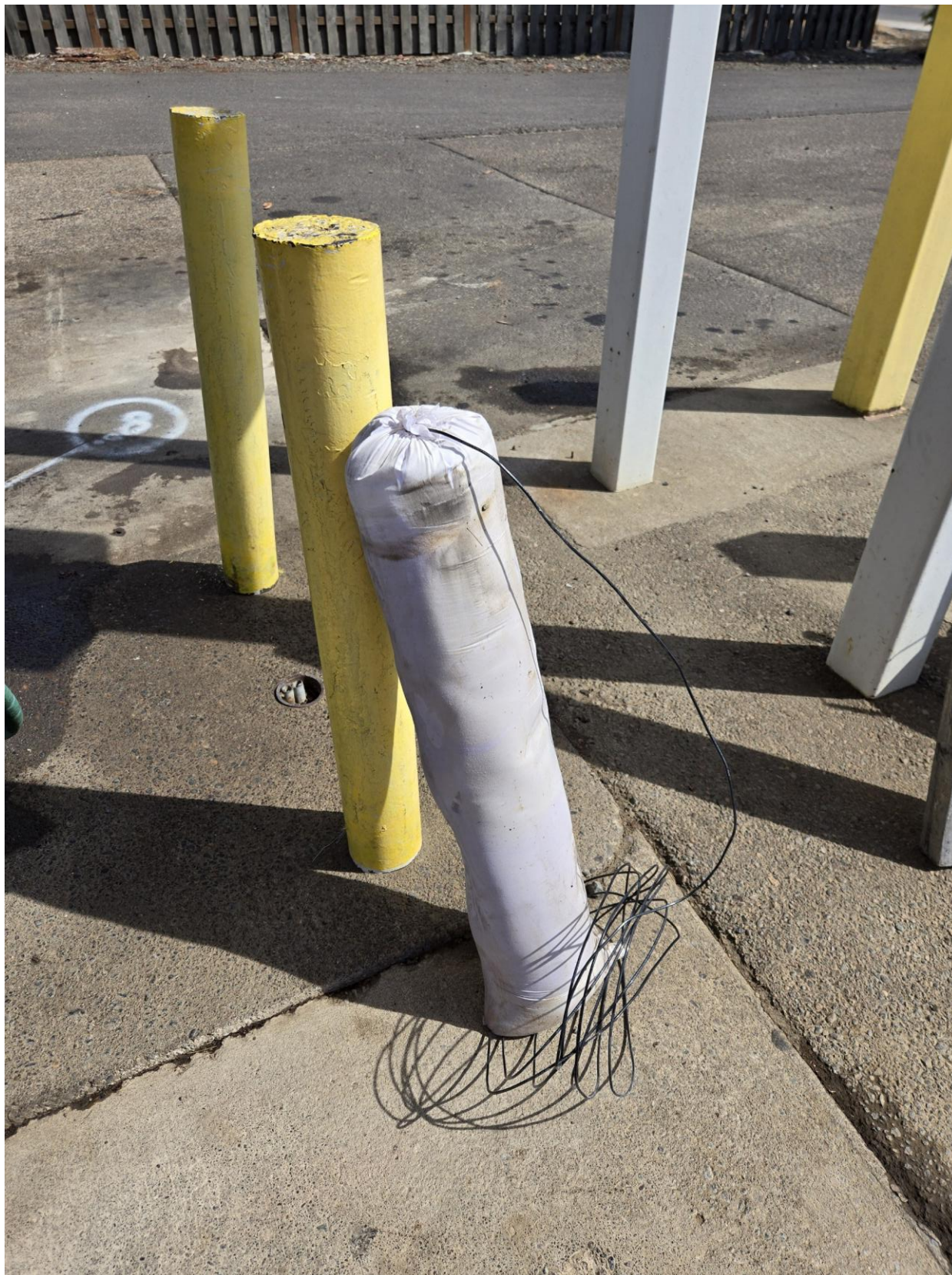
Above: Picture of a 17 lb magnesium anode installed. 6.5" x 29". Pre soaked in water 24 hours prior to install.
