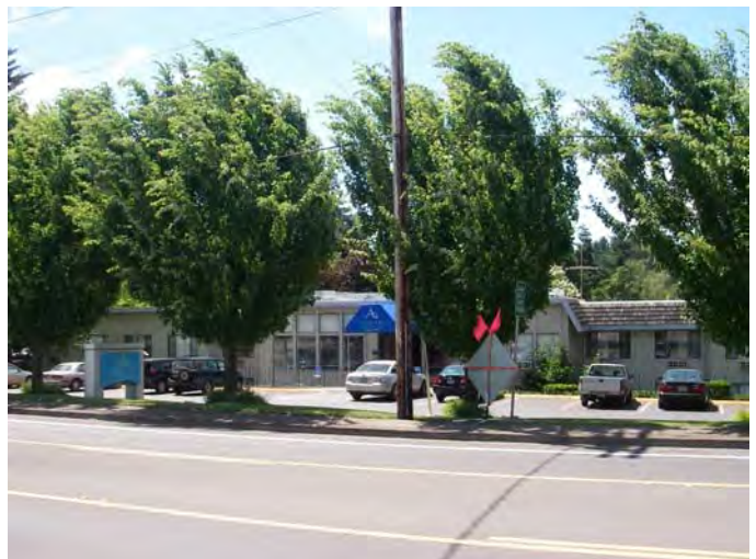
44. View of Sunnyside Road SE and the westerly adjoining commercial property (i.e., Avamere) located beyond the roadway.
