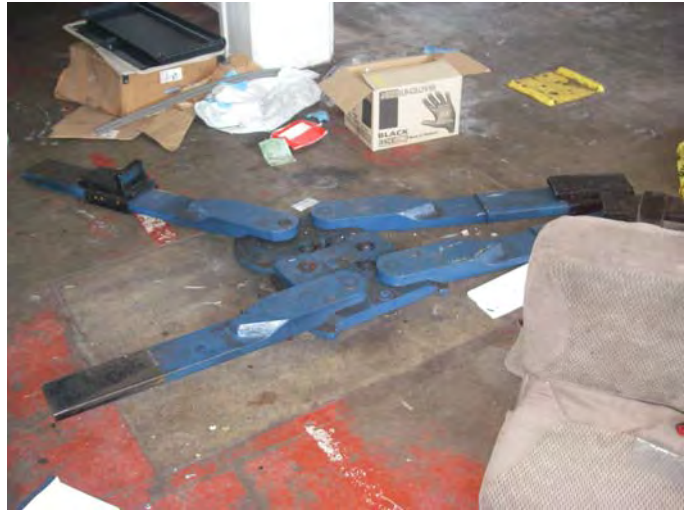
32. 4516 Sunnyside Rd SE: Representative view of intact below-ground hydraulic lifts in the former "Firehouse" building.
