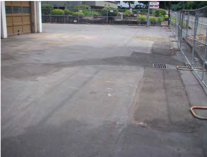
25. 4516 Sunnyside Rd SE: Photograph shows the asphalt-paved driveway and stormwater catch basins to the west of the former "Firehouse" building. View faces south.
