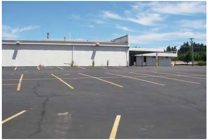
6. 4403 Commercial St. SE: Photograph shows the west side of the Main Building, the breeze way/canopy area, the Annex building, and asphalt-paved parking lot and driveway area to the west of the buildings. View faces east.
