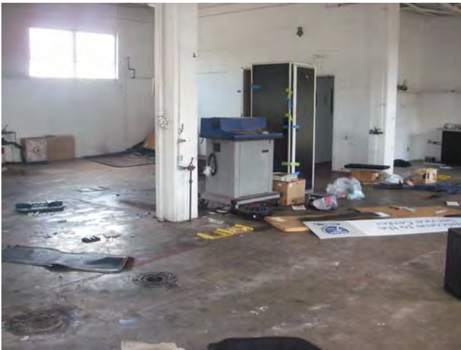
29. 4516 Sunnyside Rd SE: Another interior view of the former "Firehouse" building service area/garage showing below-ground hoists, concrete surface staining, and general debris.
