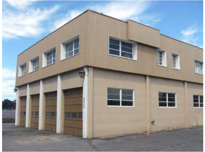
24. 4516 Sunnyside Rd SE: Photograph shows the west and south sides of the former "Firehouse" building. View is from the southwest corner of the subject property facing northeast.
