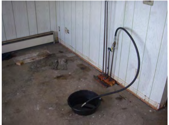
36. 4516 Sunnyside Rd SE: A room within one of four living spaces on the second floor of the former "Firehouse" building utilized to store hydraulic oil drums. Photograph shows hydraulic oil dispenser lines and a pan with some oil.
