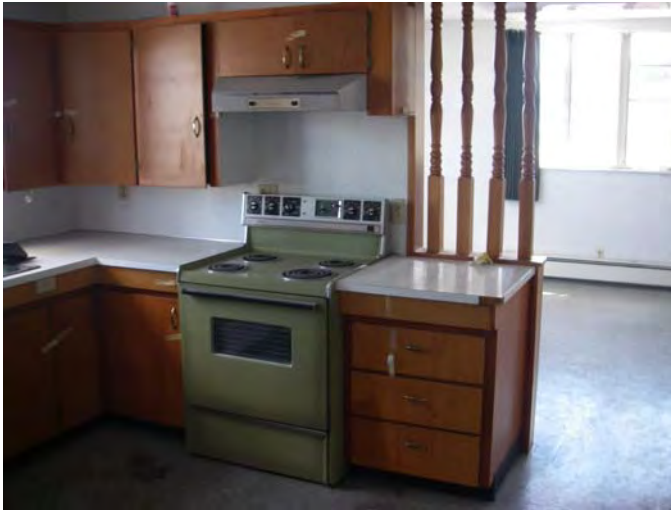
35. 4516 Sunnyside Rd SE: Represent view of one of four living spaces on the second floor of the former "Firehouse" building.
