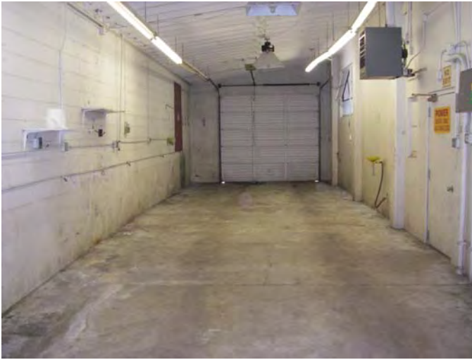
27. 4516 Sunnyside Rd SE: Interior view of the former "Firehouse" building showing the car wash area.
