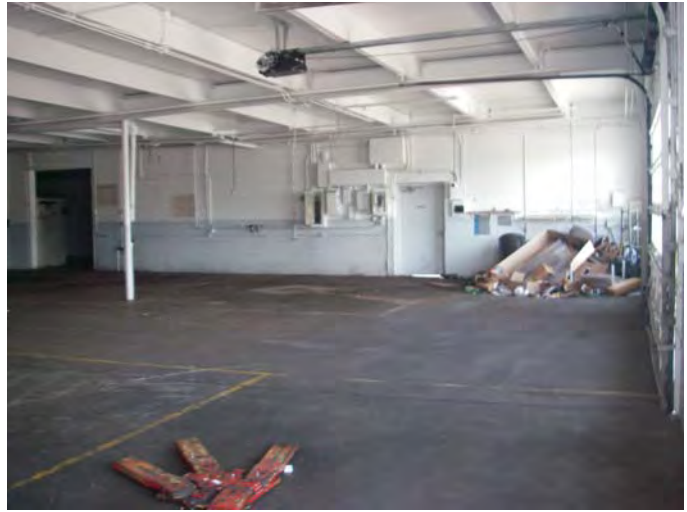
16. 4403 Commercial St. SE: Interior view of the Main Building service area/garage. View is of the northern portion of the garage from the northeast corner, and shows a below-ground hydraulic hoist and a nonhazardous trash/debris pile (including 3 empty 55-gallon poly drums).
