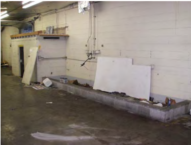
21. 4403 Commercial St. SE: Interior view of the Main Building oil and waste storage area showing secondary containment areas.
