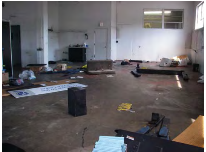
30. 4516 Sunnyside Rd SE: Another interior view of the former "Firehouse" building service area/garage showing below-ground hoists, concrete surface staining, and general debris. Photograph also shows the decommissioned floor drain in the right-central vicinity of the photograph.
