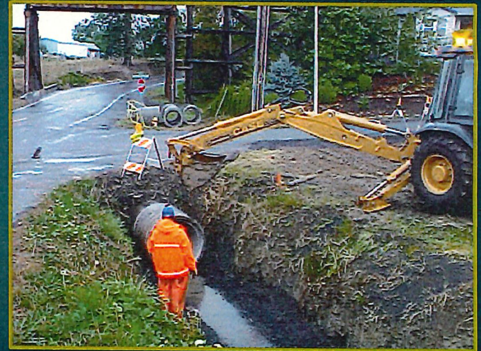
Villa Road Culvert
