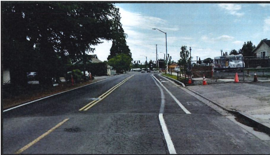
FIGURE 4 LOOKING SOUTH ON ELLIOTT ROAD
