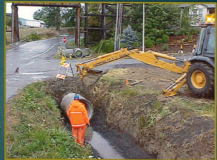
Villa Road Culvert
