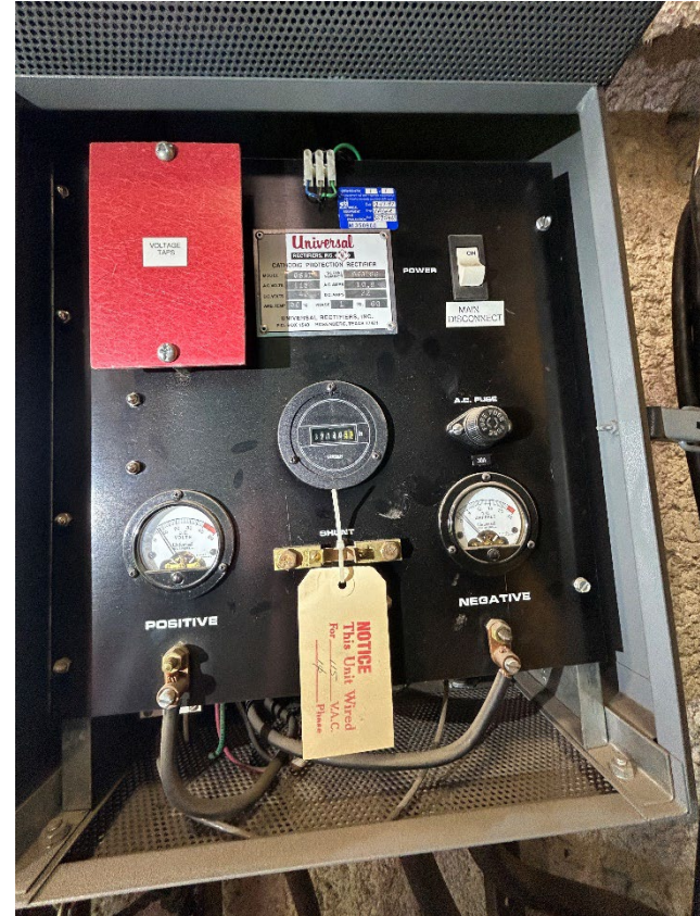
2: Impressed current rectifier
