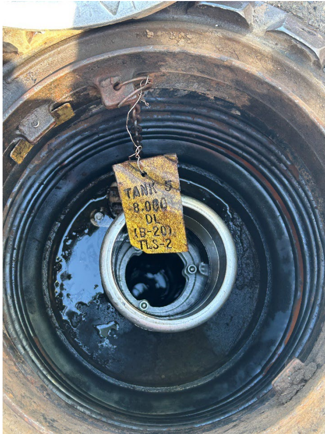
7: Fill for bio diesel 8,000 gallon
