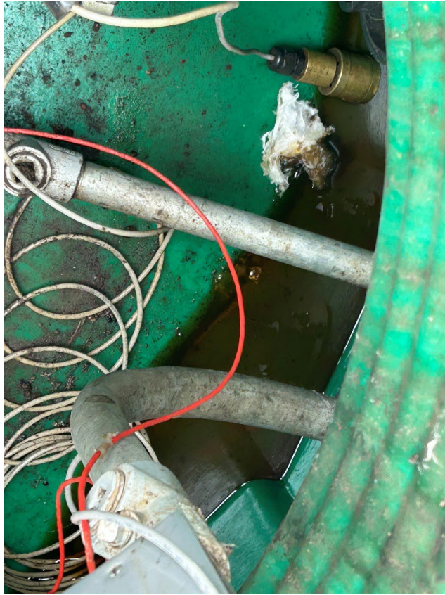
11: Confirmed product in diesel sump #1
