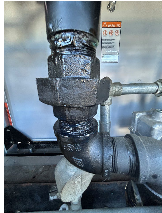
6: Regular pipe weeping in UDC #1/2
