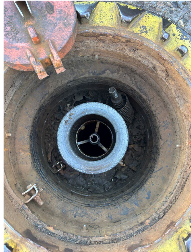
22: Regular vapor return with broken poppet valve
