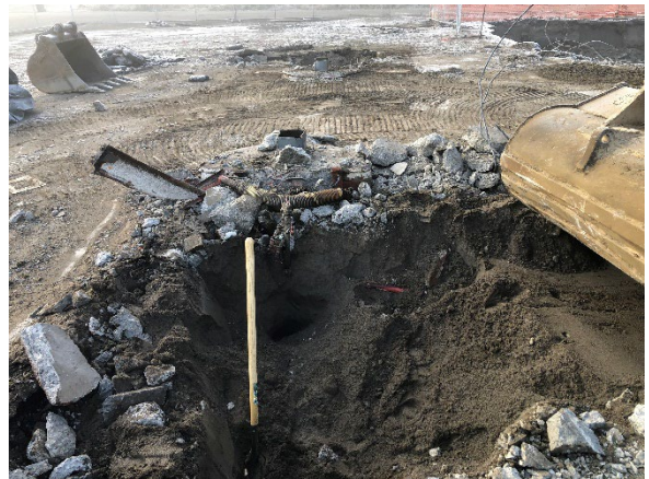
Photo #8 Sampling under dispenser sump following removal
