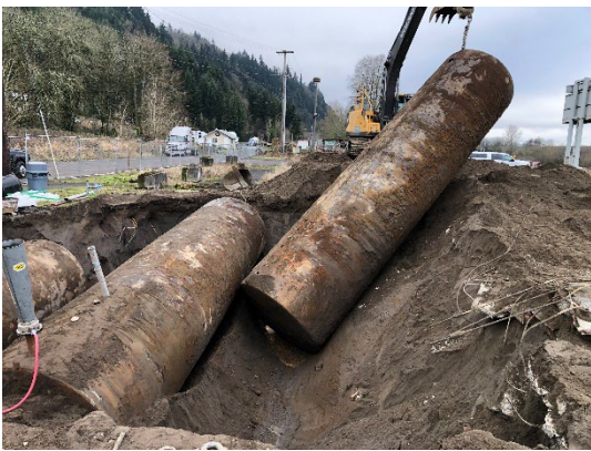
Photo #5 Removing USTs from pit
