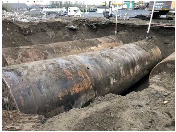
Photo #2 Removing residual product/sludge from USTs prior to cleaning and ventilation
