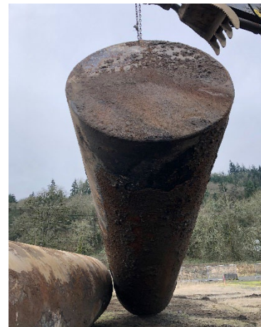
Photo #6 Staging USTs on-site prior to recycling. USTs appear in good condition
