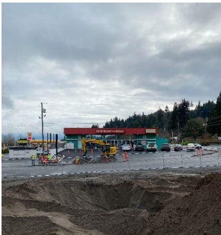
Photo #9 Remedial Excavation at northeast dispenser location
