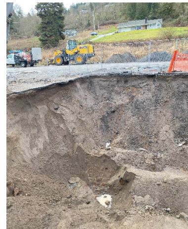
Photo #10 Groundwater in former UST pit on February 3, 2025
