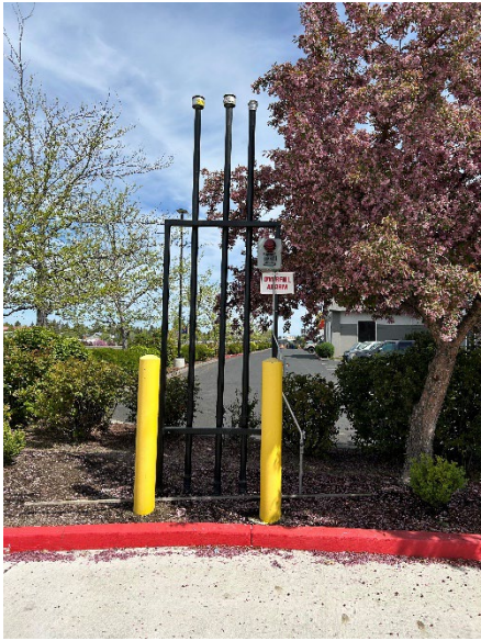
Figure 5 Vents and Overfill Alarm
