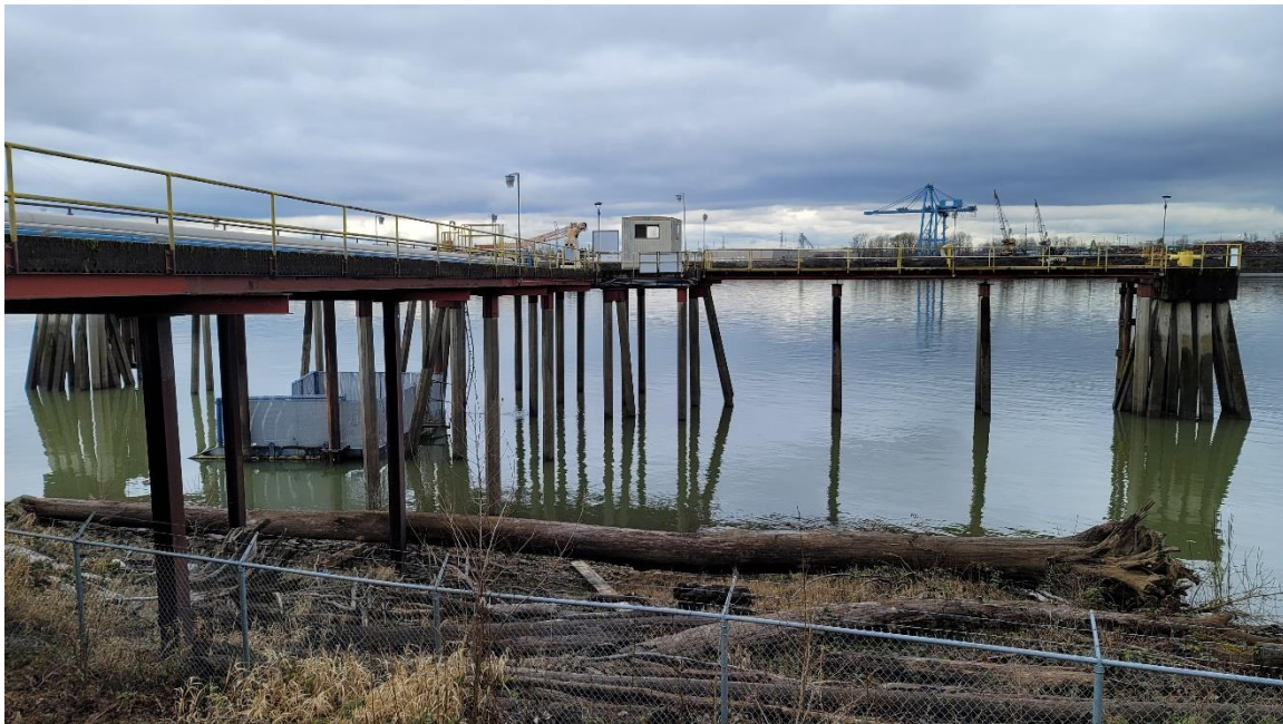
Picture 12. View of dock structure.
