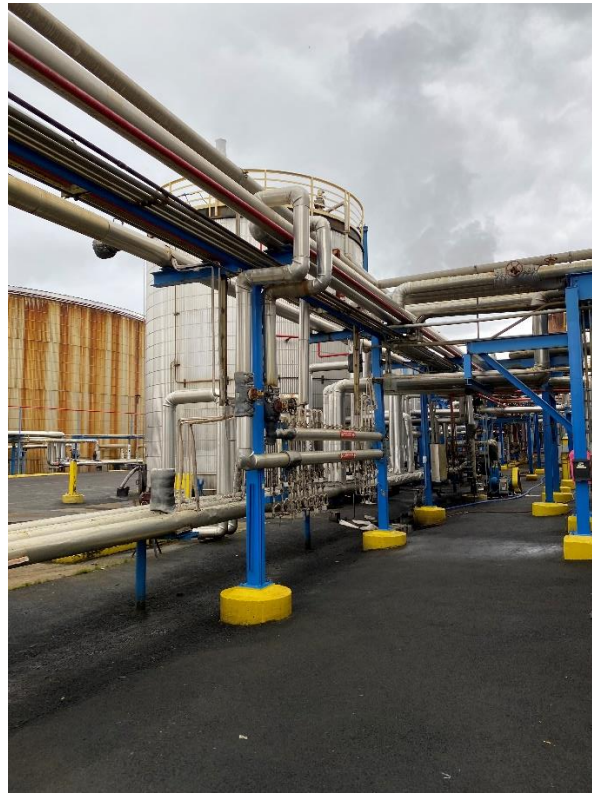
Picture 1. Typical view of Process area.
