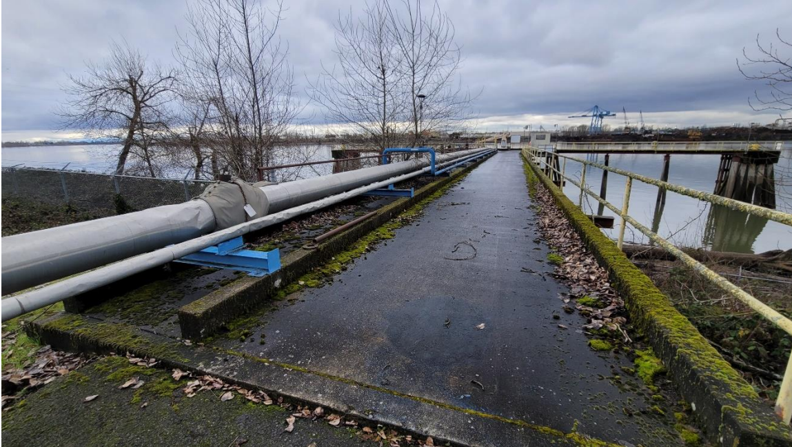
Picture 13. View of piping at dock structure.
