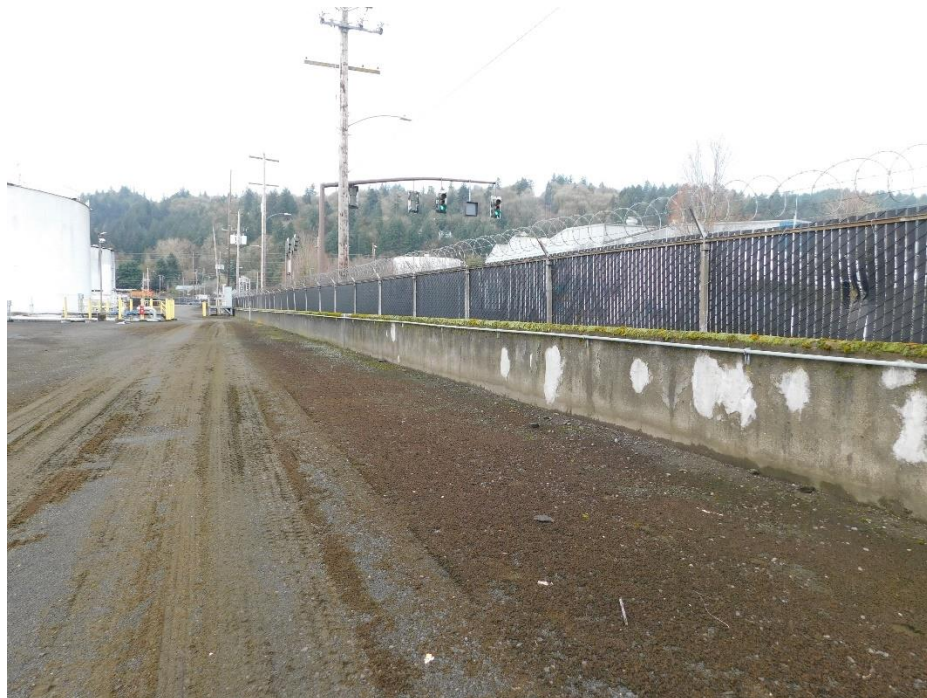
Picture 8. Containment wall structure at North Yard.
