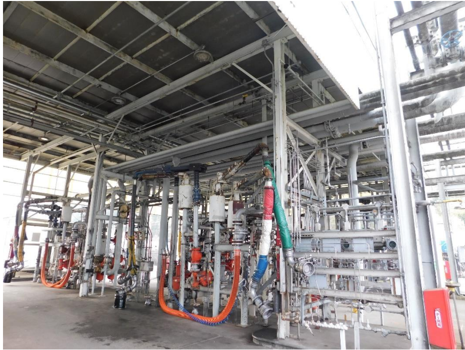
Picture 7. North Yard truck loading rack framing.
