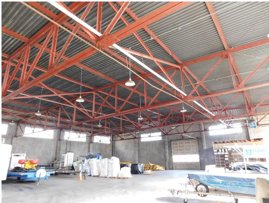
Picture 4. New roof structure at Warehouse A.
