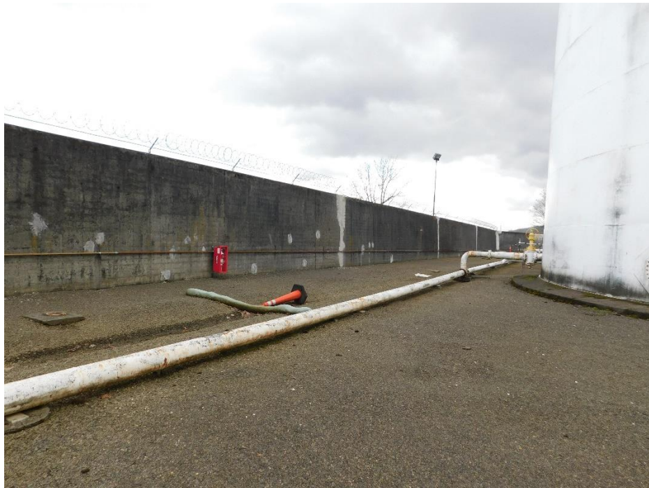
Picture 8. Typical containment wall structure.
