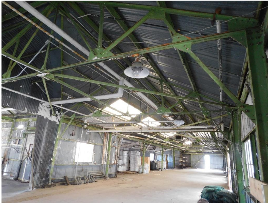
Picture 5. Typical warehouse building at Area 01.
